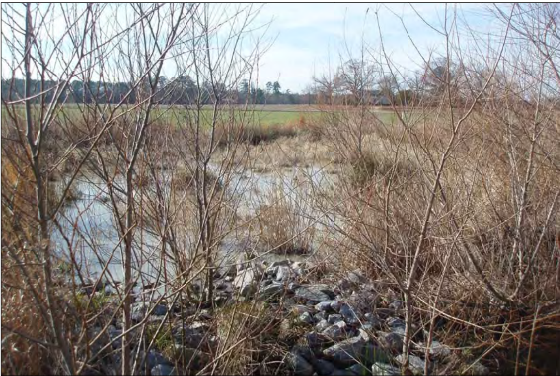
Photo Point S4: View of water quality treatment structure near Station 32+25. 1/12/12 – MY-04
