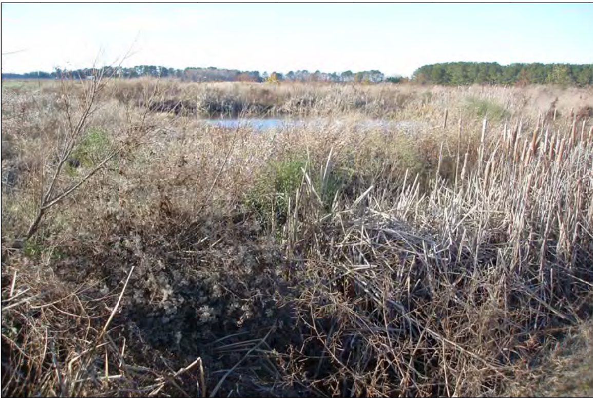
Photo Point S14: View of stream with water quality treatment structure in the background near Station 62+60. 1/12/12 – MY-04
