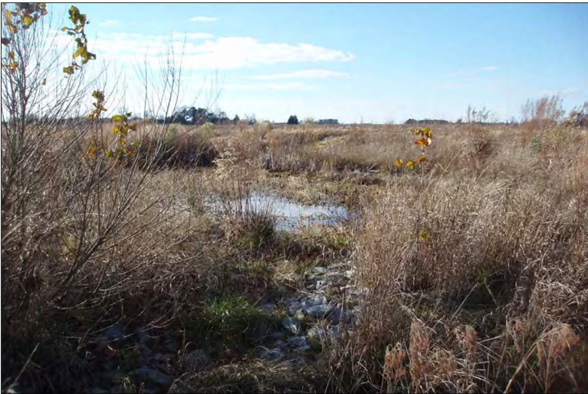
Photo Point S11: View of water quality treatment structure near Station 47+00. 1/12/12 – MY-04
