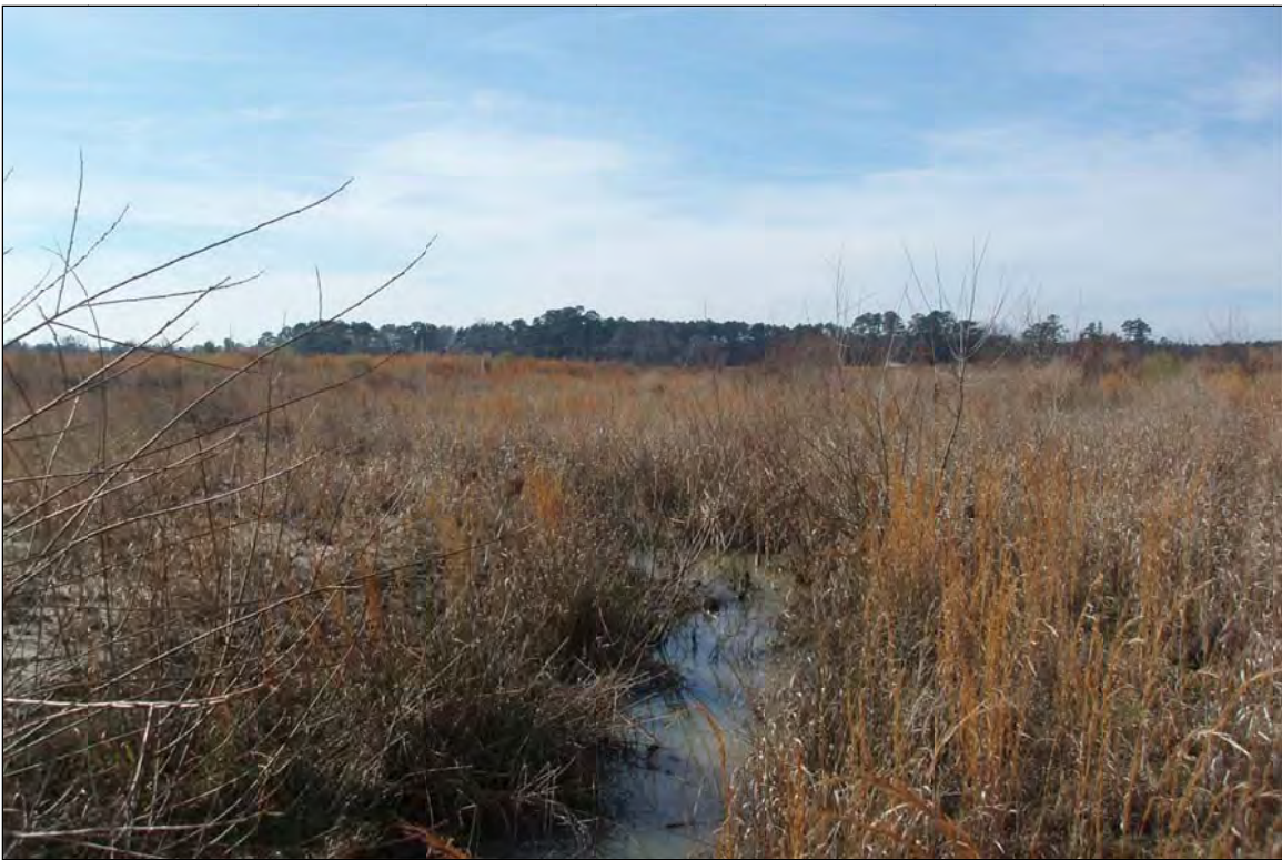
Photo Point S8: View of log drop structure near Station 39+50. 1/12/12 – MY-04
