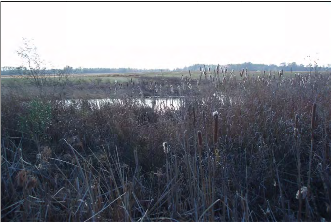
Photo Point S13: View of water quality treatment structure near Station 61+50. 1/12/12 – MY-04
