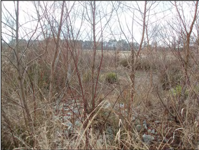
Photo Point S4: View of water quality treatment structure, near Station 32+25. 12/18/12 – MY-05
