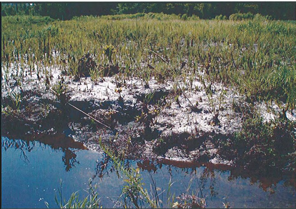
SPA 3. Right bank erosion at UT2 STA 14+50.
