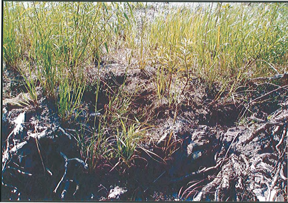
SPA 2. Root wad erosion at UT2 STA 12+50.
