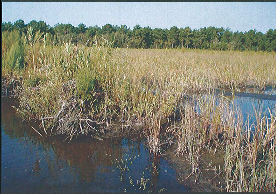
SPA 1. Right bank is washed out behind root wad at UT1A STA 38+00.
