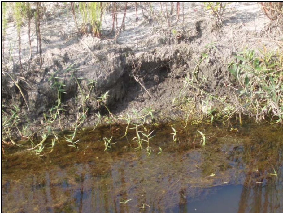
16+75 UT-3 RB. Erosion on both banks below log weir.
