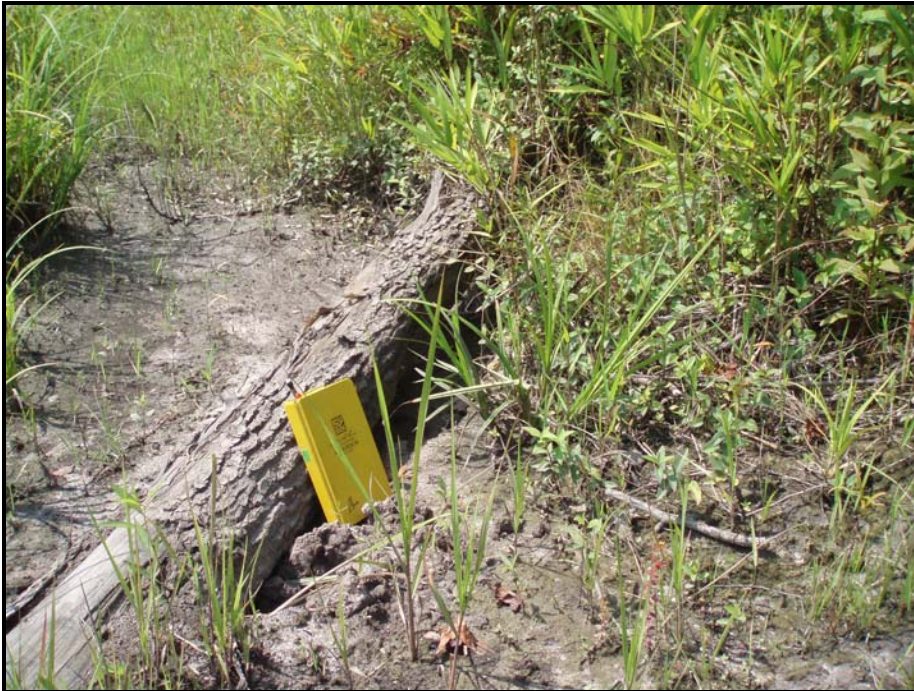
68-85 UT-1B DS. Undercut at log vane. Improper installation
