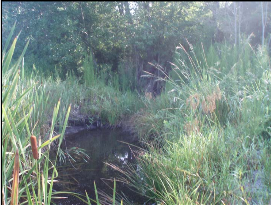
10+00 UT-3 US. Minor erosion on right bank
