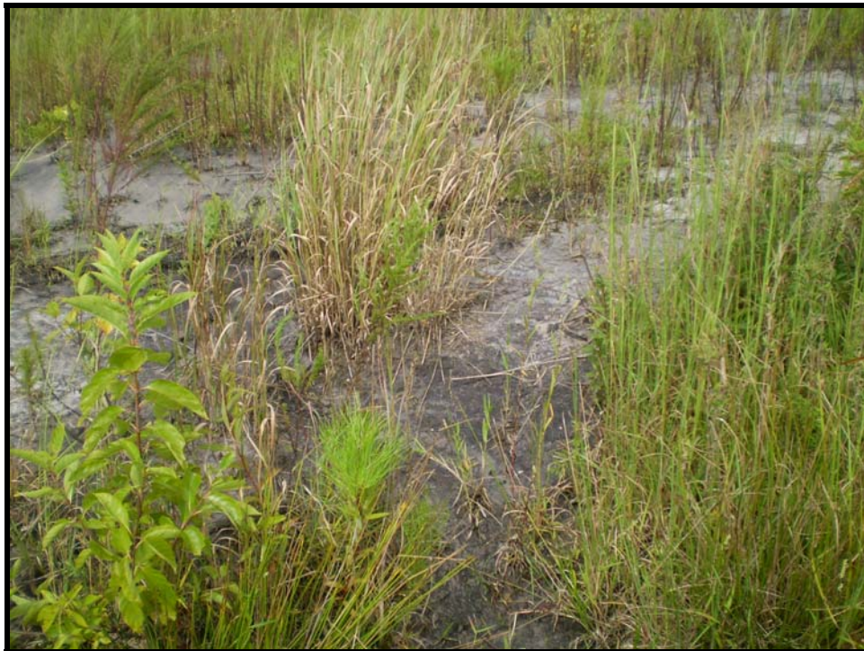
SPA 4. UT2 Sta.29+45 Right bank erosion
