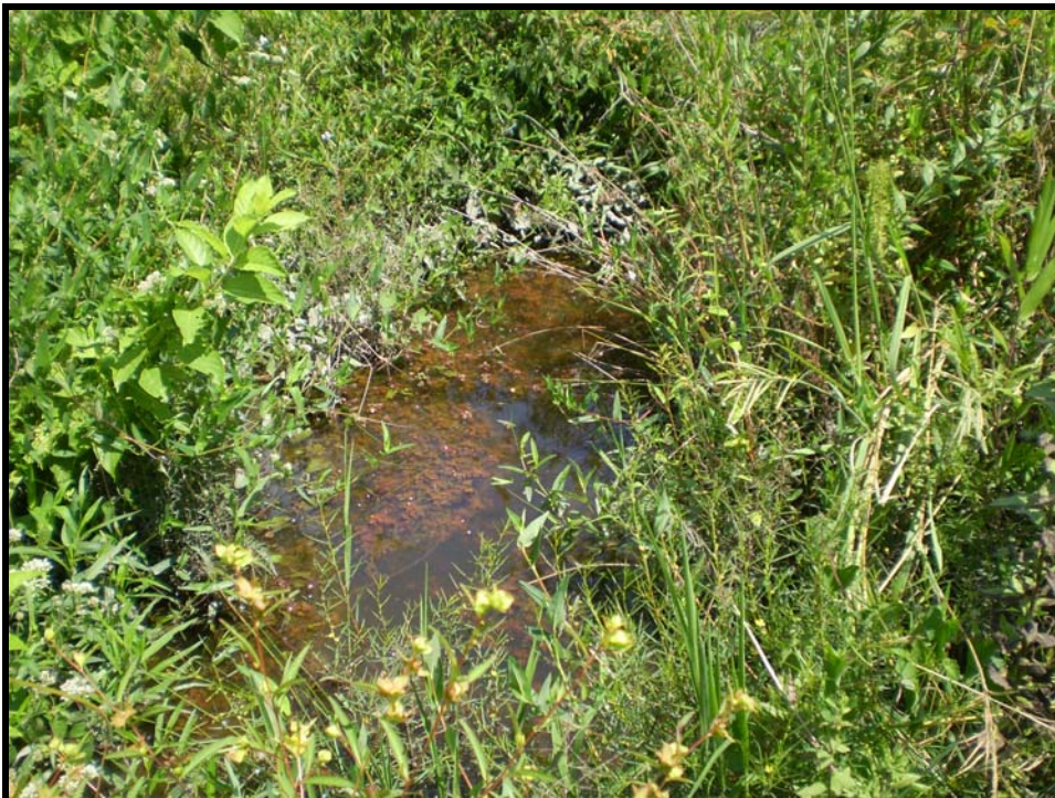
SPA 6 – Settled ditch plug @ Sta. 12+00 (UT3)
