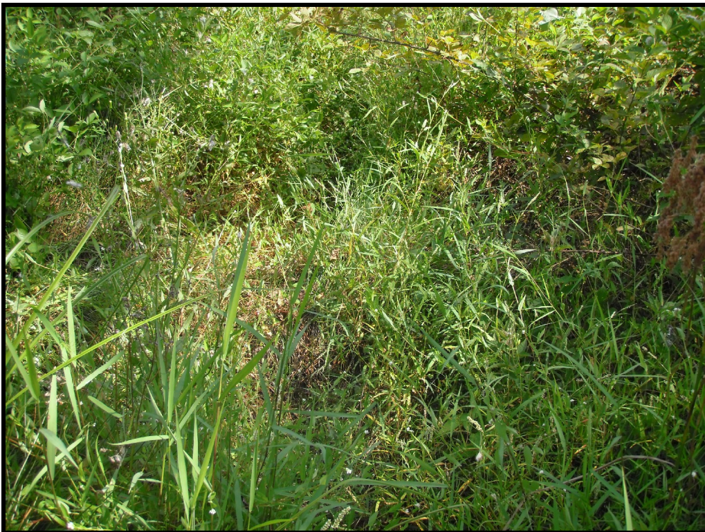
ID #2 – Beaver dam, STA 12+20
