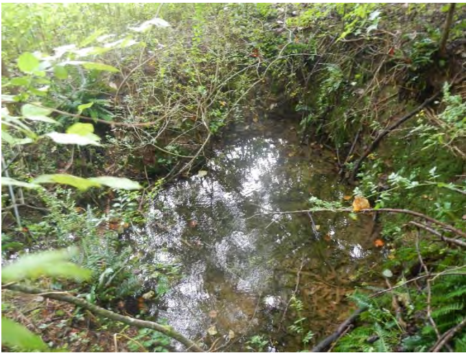
Groundwater seep at US end of UT1B (8/22/2013)
