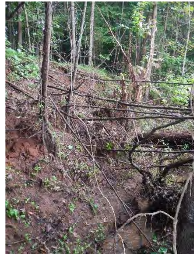
Bank failure along UT1 (8/22/2013)
