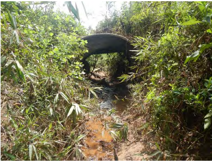
Culvert crossing on lower UT2 (8/22/2013)
