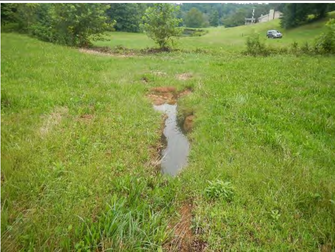
Valley scour adjacent to UT1 (8/22/2013)
