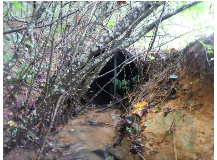
UT1 culvert crossing below UT1B (8/22/2013)
