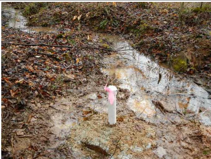
Groundwater gauge installed in Wetland D (3/18/2014)
