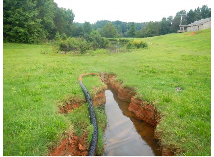
Additional scour in UT1 valley (8/22/2013)
