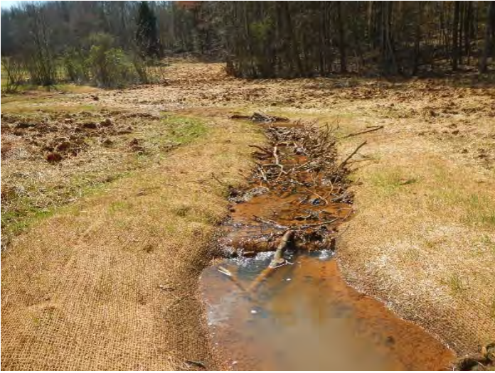
Photo Point 9 – looking upstream UT1 R1 Lower (03/16/2016)
