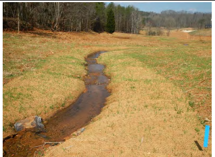
Photo Point 3 – looking downstream UT1 R1 Upper (03/16/2016)
