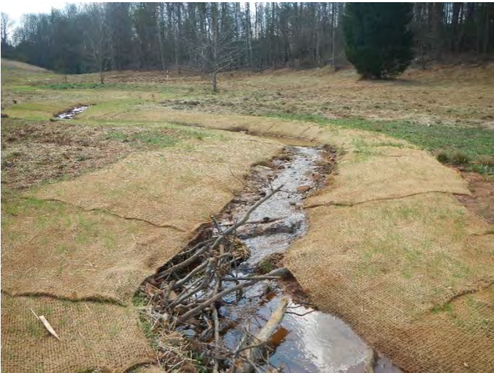
Photo Point 7 – looking upstream UT1 R1 Lower (03/16/2016)
