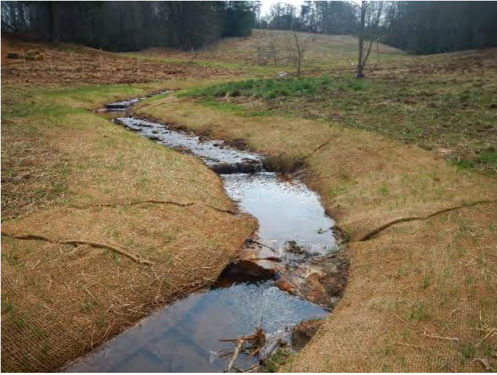
Photo Point 6 – looking upstream UT1 R1 Lower (03/16/2016)
