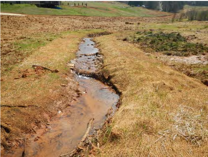
Photo Point 10 – looking upstream UT1 R1 Lower (03/16/2016)
