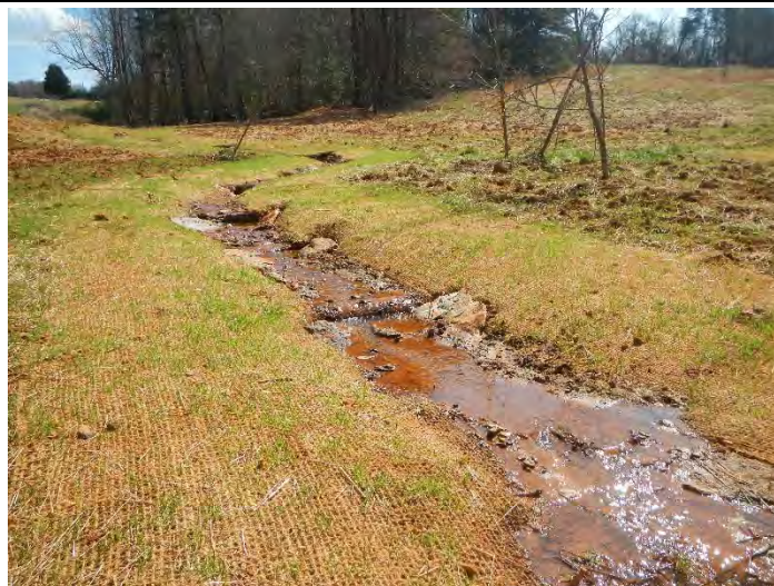
Photo Point 5 – looking upstream of UT1B (03/16/2016)
