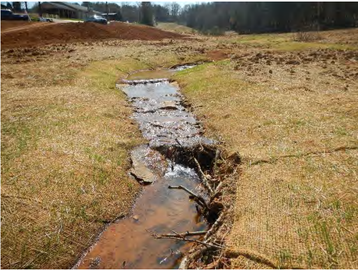
Photo Point 12 – looking upstream UT1 R1 Lower (03/16/2016)
