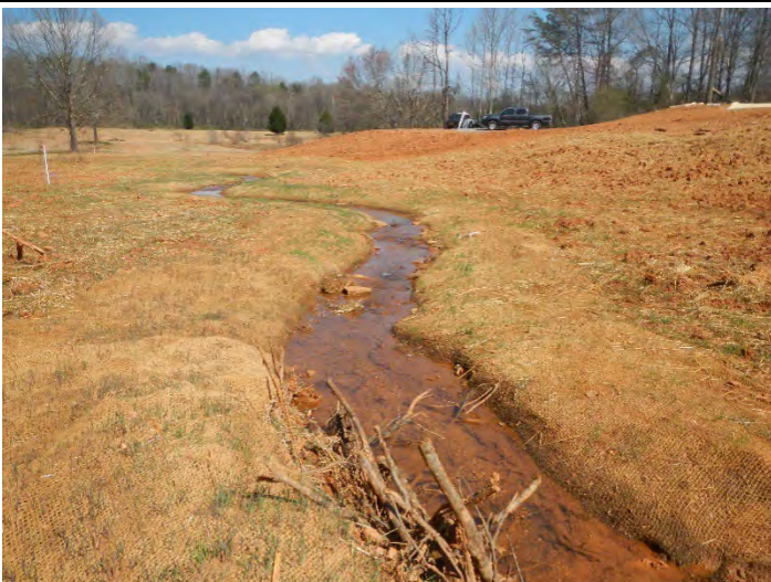
Photo Point 10 –looking downstream UT1 R1 Lower (03/16/2016)
