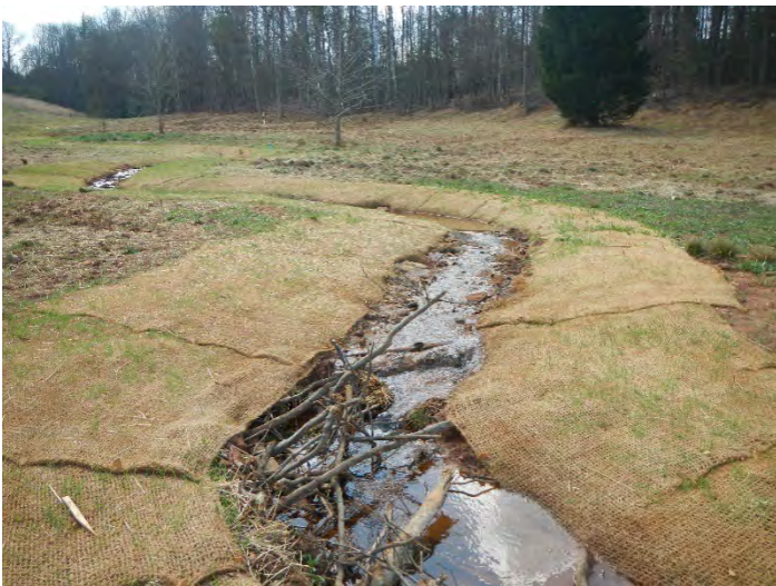
Photo Point 7 – looking upstream UT1 R1 Lower (03/16/2016)
