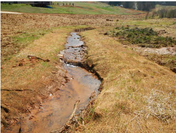
Photo Point 10 – looking upstream UT1 R1 Lower (03/16/2016)
