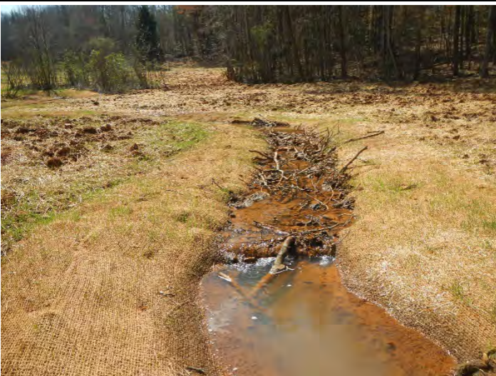
Photo Point 9 – looking upstream UT1 R1 Lower (03/16/2016)
