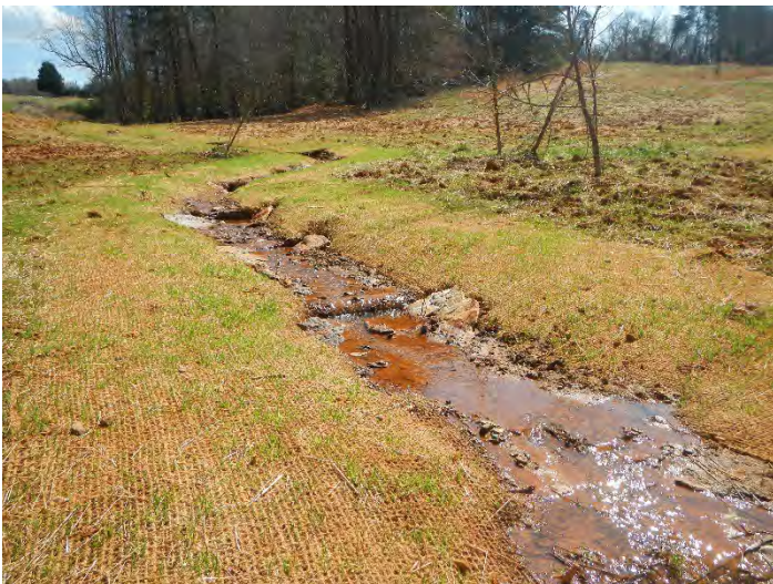
Photo Point 5 – looking upstream of UT1B (03/16/2016)
