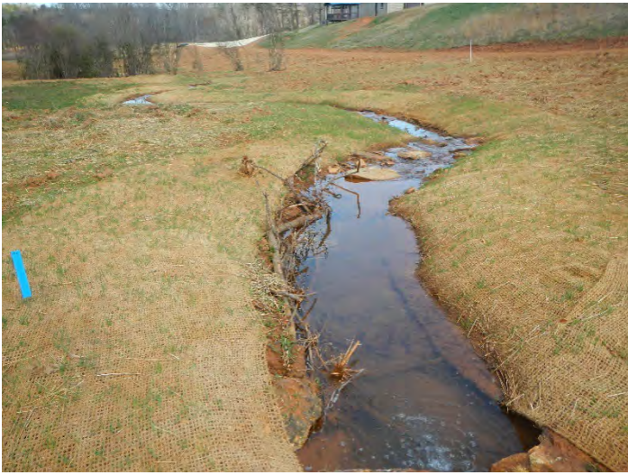
Photo Point 6 – looking downstream UT1 R1 Lower (03/16/2016)
