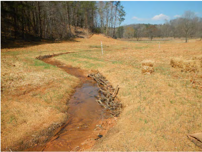
Photo Point 9 – looking downstream UT1 R1 Lower (03/16/2016)
