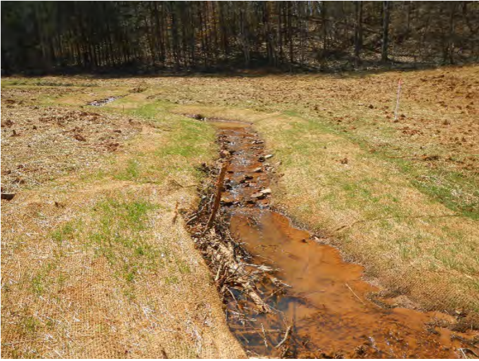
Photo Point 11 – looking upstream UT1 R1 Lower (03/16/2016)
