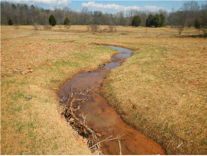
Photo Point 12 –looking downstream UT1 R1 Lower (03/16/2016)
