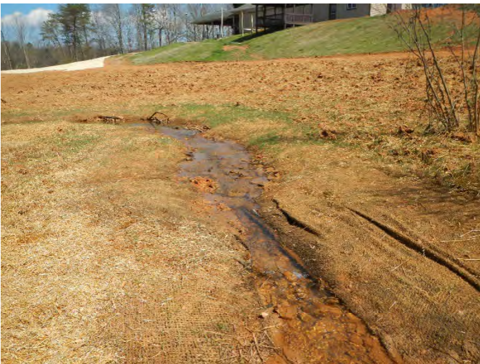
Photo Point 8 – looking downstream UT1 R1 Lower (03/16/2016)
