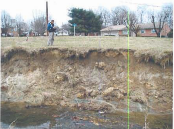
Bank Erosion Downstream
