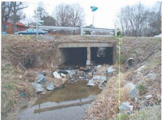
Culvert Downstream of S. Benbow Rd.
