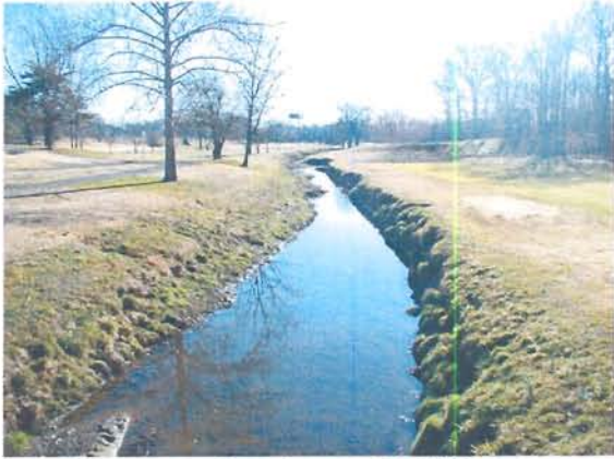
Upstream Section on Golf Course
