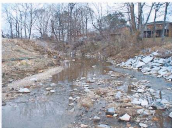
Reach 1 Downstream of Culvert at W. Meadowview
