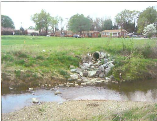
PP5 Reach 1A Constructed Riffle #1 & Step Pool- #1-Year 1
