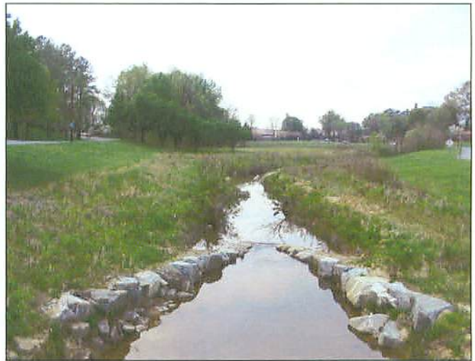
PP13 Reach 1A End (Upstream view)-Year 1
