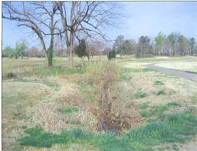
PP30B Managed Buffer Herbaceous Perennials/Live stakes Plot Looking Upstream to Reach 4 from Confluence with Reach 5-Year 1
