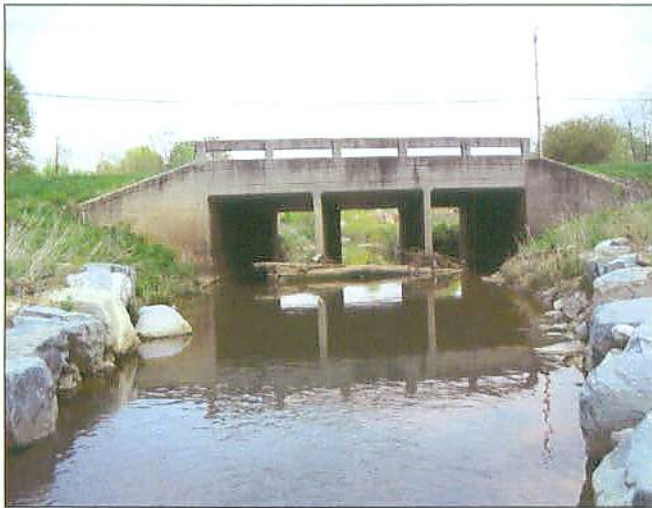
PP12 Reach 1A Cross Vane #1 & Vanstory Culvert-Year 1
