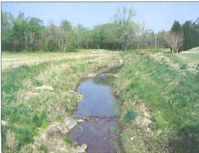
PP4A Reach 1A Looking Upstream-Year 1
