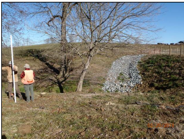
Photo 17- Spillway below Pond 3.
