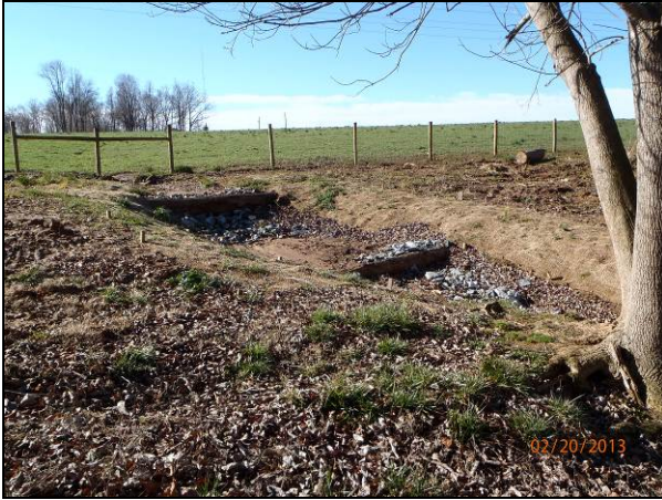
Photo 19- Erosion control structure on UT3.
