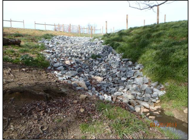
Photo 14-Pond 2 Spillway.
