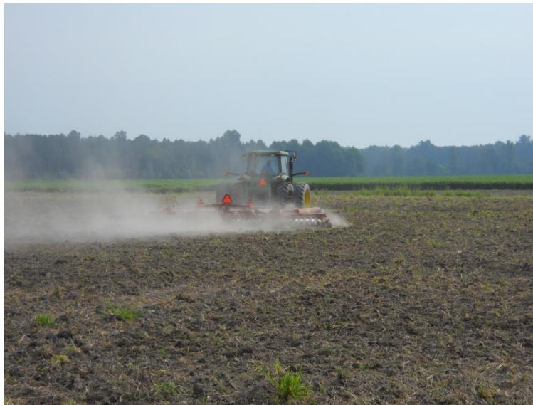
Photo 2: Disking site to remove vegetation prior to construction
