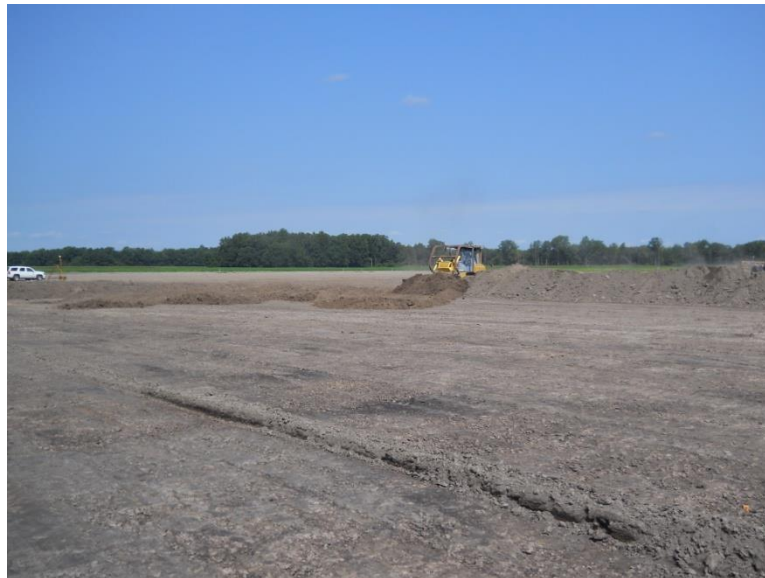
Photo 4: Redistribution of topsoil and final grading
