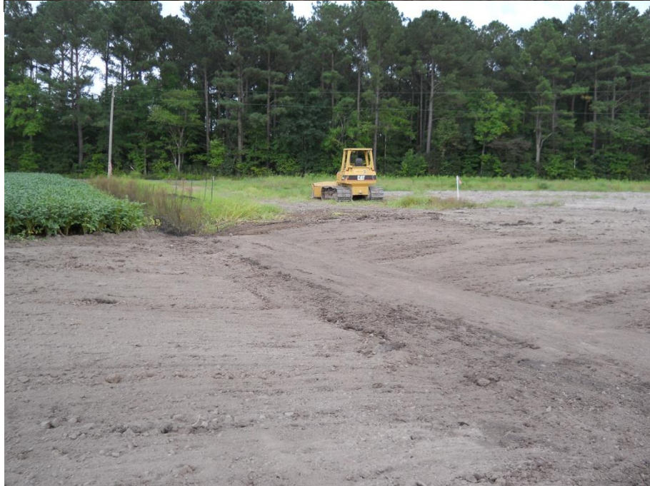
Photos 5&6: Completed ditch plugs after construction
