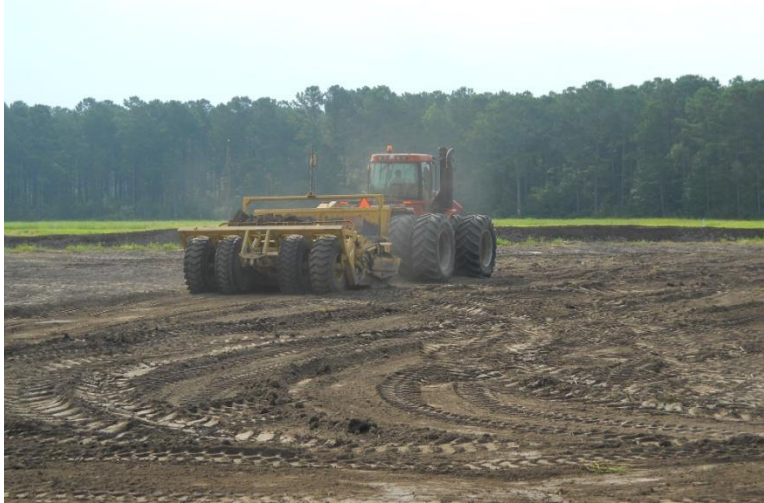
Photo 3: Removal of subsoil during construction
