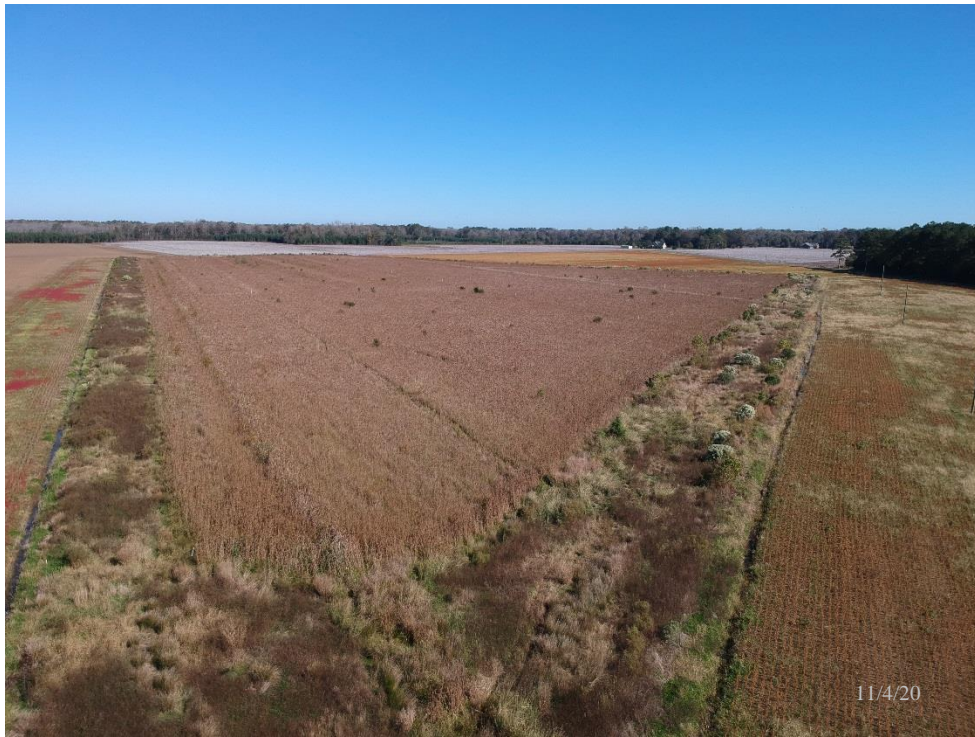
View looking northeast across project
