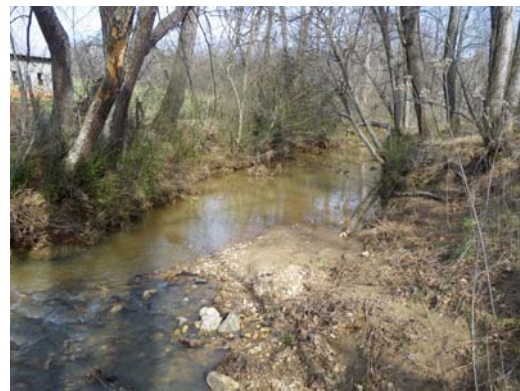
Hogan Creek, looking downstream from station 33+75; narrow buffers; levee on right bank; March 8, 2011
