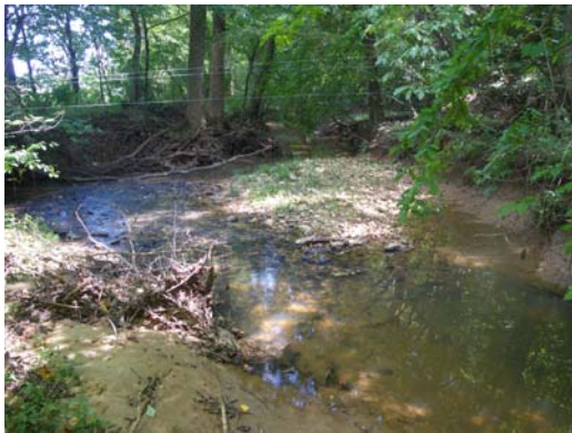
Hogan Creek, looking downstream from station 16+00; leaning trees, bank erosion; mid-channel bar; September 12, 2011
