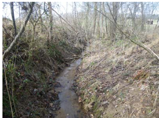
UT3, looking downstream from station 11+00. Straightened channel with levees on both banks; March 8, 2011
