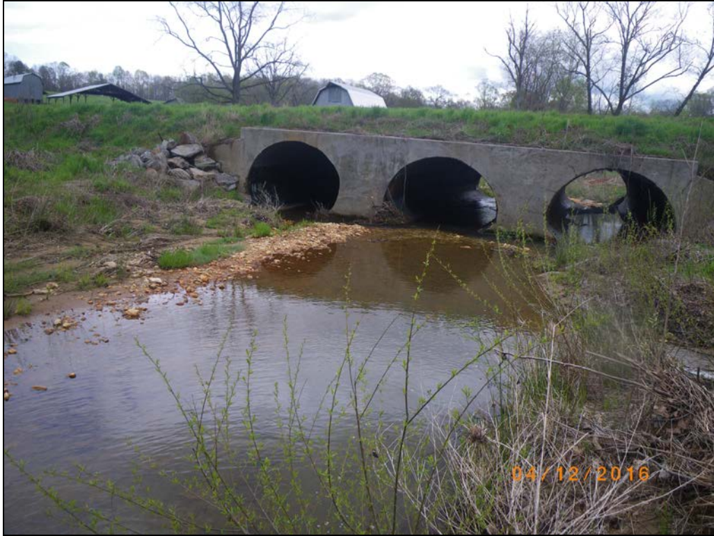
Photo Point 7 – View Downstream, Main Stem UT2
