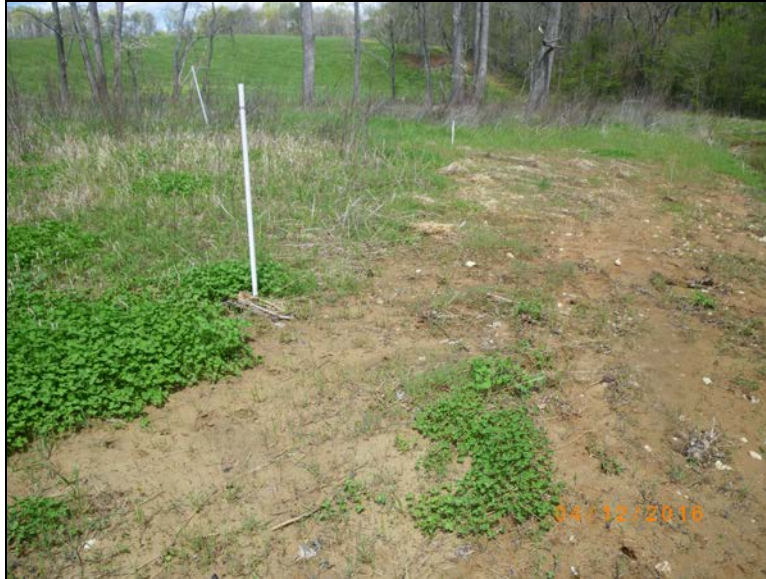
Photo 3. Wrack lines and sediment deposition on Hogan Creek Reach 3 Station 37+00, April 12, 2016
