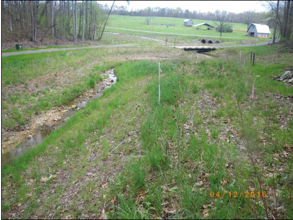
Photo Point 5 – View Downstream, Main Stem UT2
