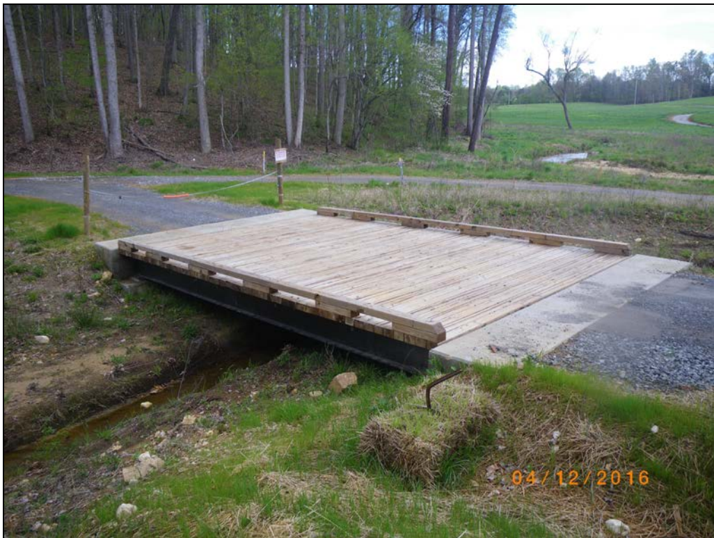
Photo Point 6 – View Downstream, Main Stem UT2
