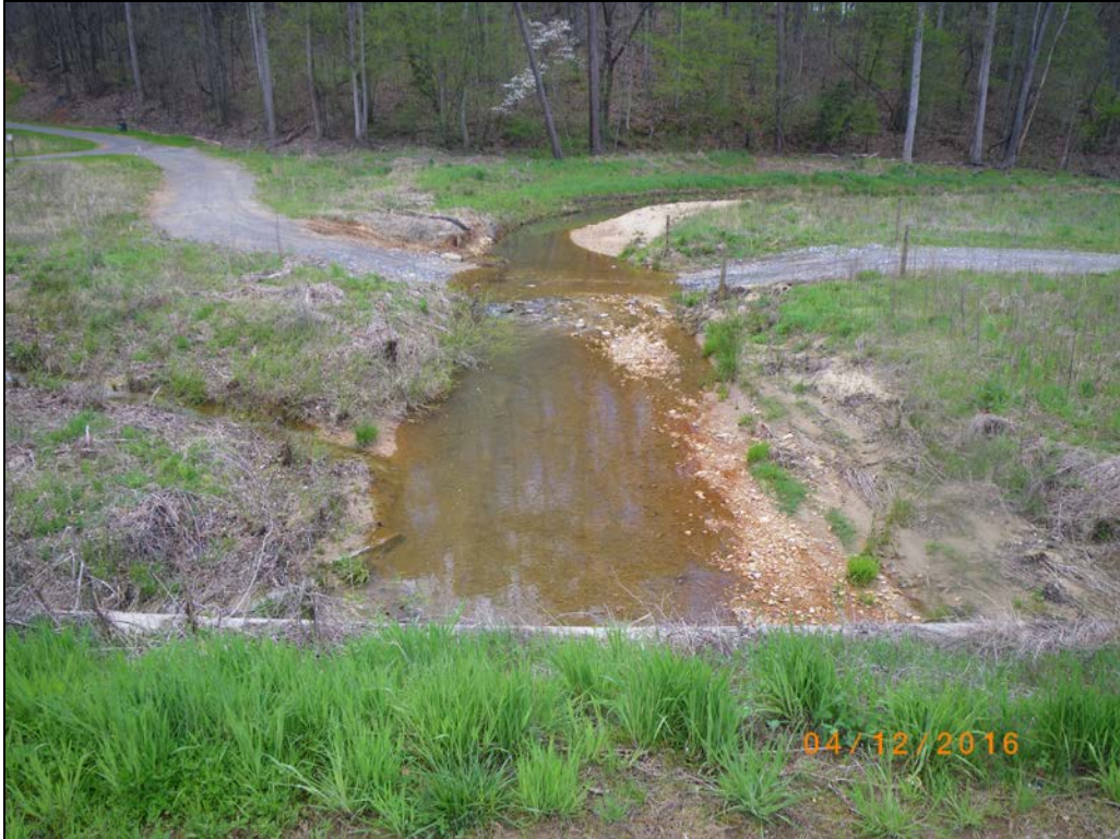
Photo Point 25 – View Upstream, Reach 2 Hogan Creek
