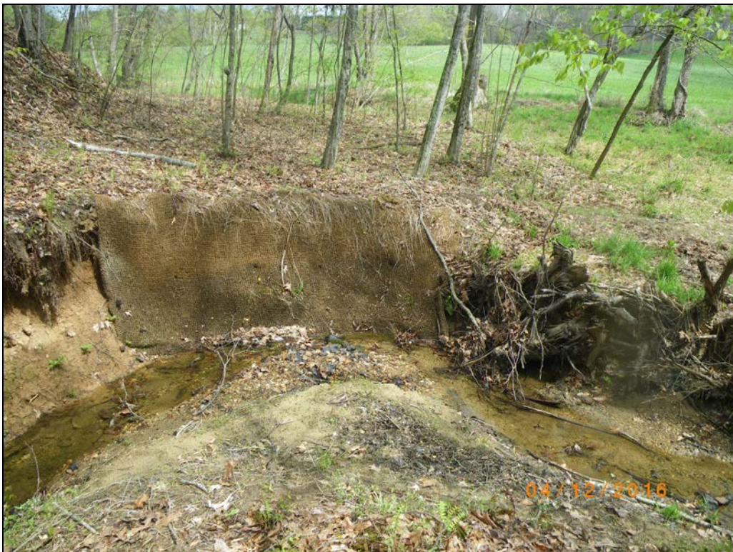
Photo Point 16 – View Downstream, Main Stem UT1
