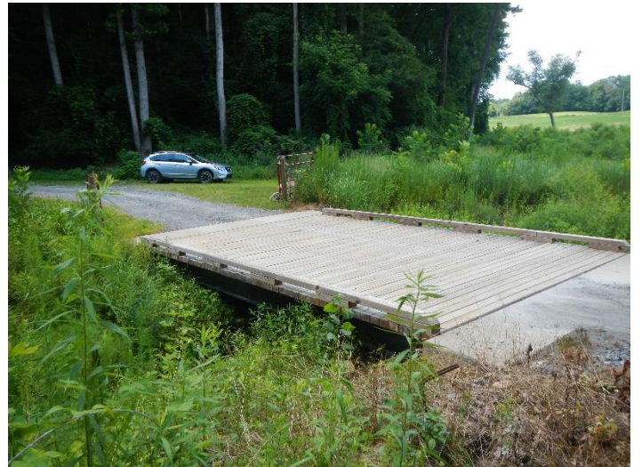
PP6 – Main Stem UT2, looking downstream (07/05/2017)
