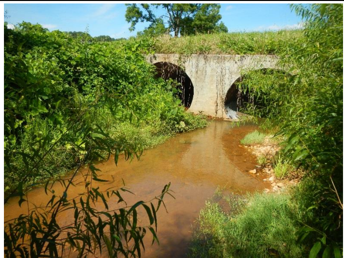
PP7 – Main Stem UT2, looking downstream (07/05/2017)
