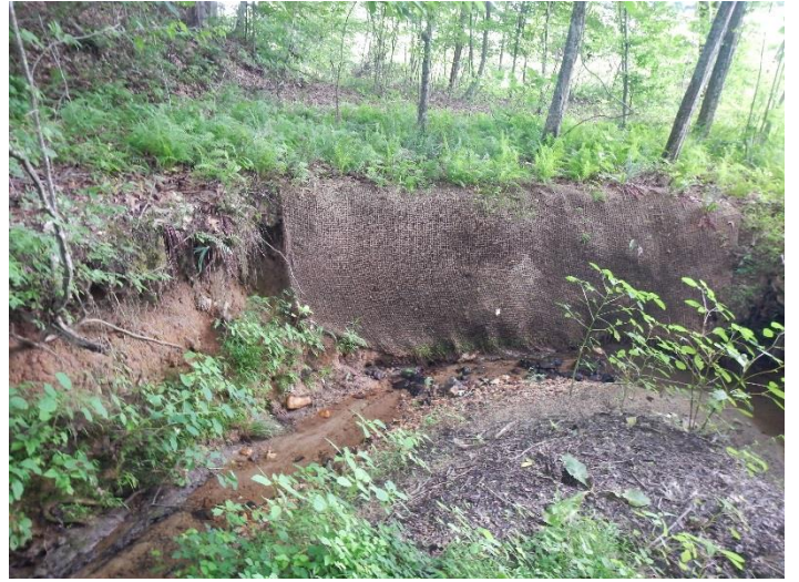
PP16 – Main Stem UT1, looking downstream (07/05/2017)
