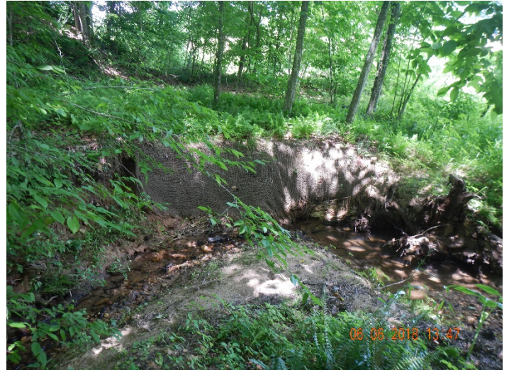
PP16 – Main Stem UT1, looking downstream (6/06/2018)
