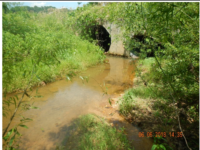
PP7 – Main Stem UT2, looking downstream (6/06/2018)
