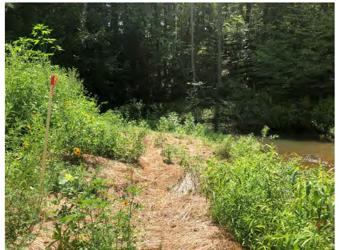
Hogan Creek Reach 1 STA 16+50 left bank repair – (8/19/2019)
