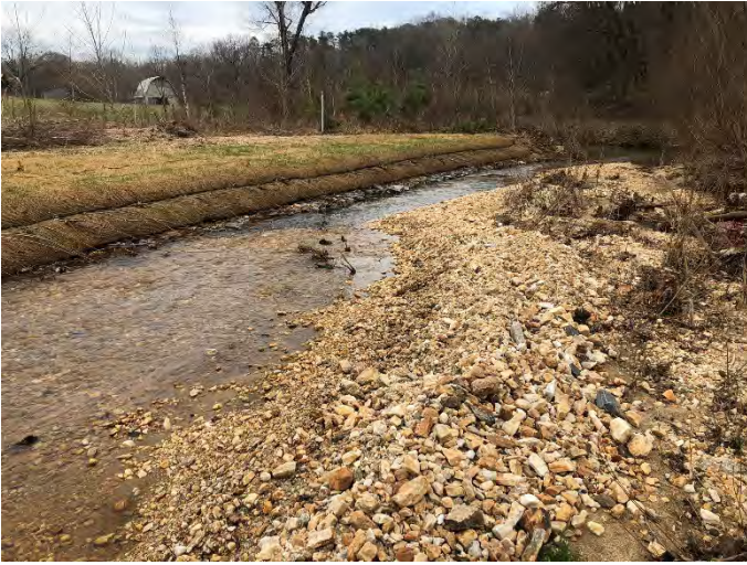
Hogan Creek Reach 1 STA 23+20 left bank repair – (3/13/2019)
