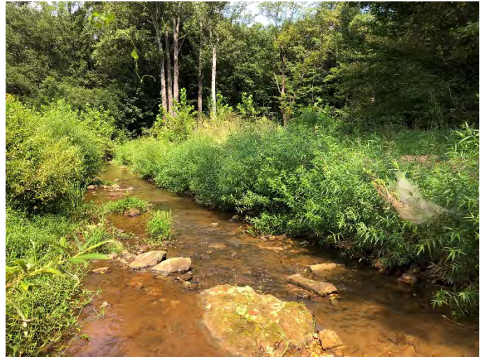
Hogan Creek Reach 2 STA 37+70 right bank repair – (8/19/2019)
