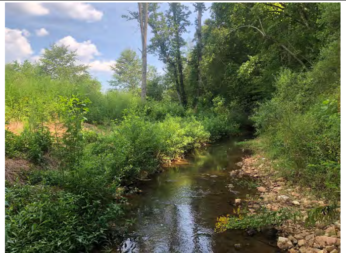
Hogan Creek Reach 1 STA 20+10 left bank repair – (8/19/2019)
