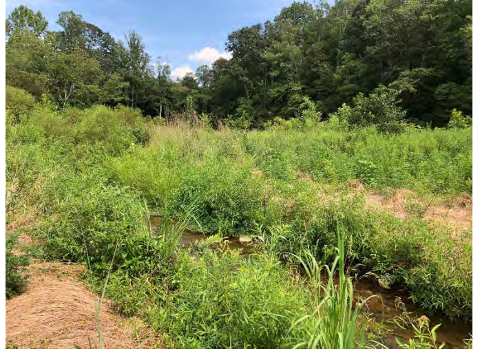
Hogan Creek Reach 2 STA 34+00 repair on both banks view downstream – (8/19/2019)
