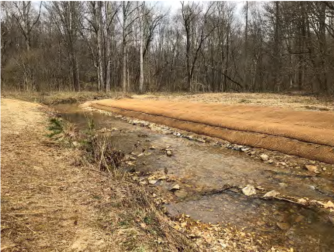
Hogan Creek Reach 2 STA 37+70 right bank repair – (3/13/2019)
