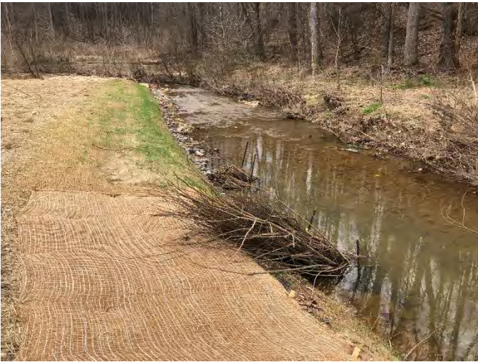
Hogan Creek Reach 1 STA 26+70 left bank repair – (3/13/2019)
