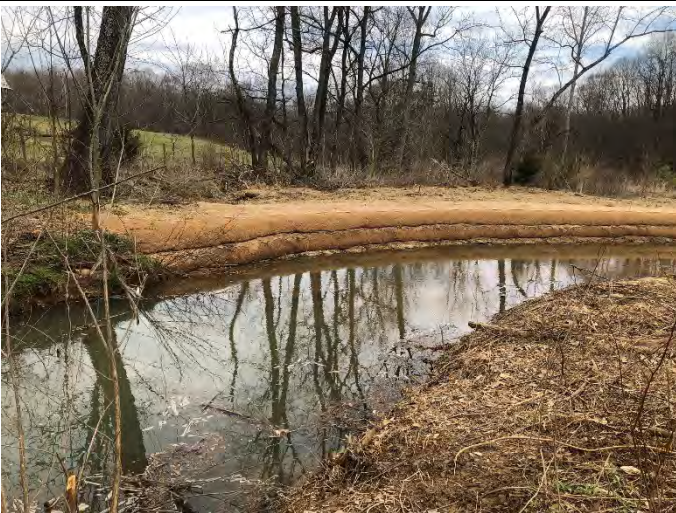
Hogan Creek Reach 2 STA 31+30 left bank repair – (3/13/2019)
