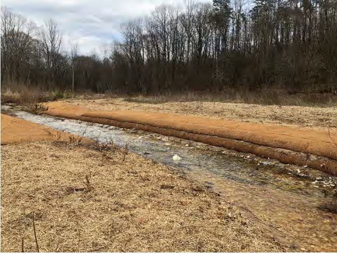
Hogan Creek Reach 2 STA 34+00 repair on both banks view downstream – (3/13/2019)
