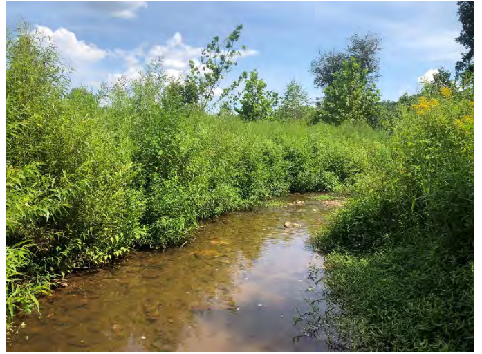
Hogan Creek Reach 1 STA 23+20 left bank repair – (8/19/2019)
