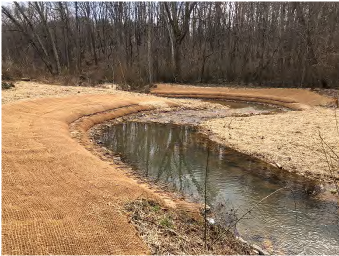
Hogan Creek Reach 1 STA 10+20 left bank and 10+80 right bank repairs – (3/13/2019)
