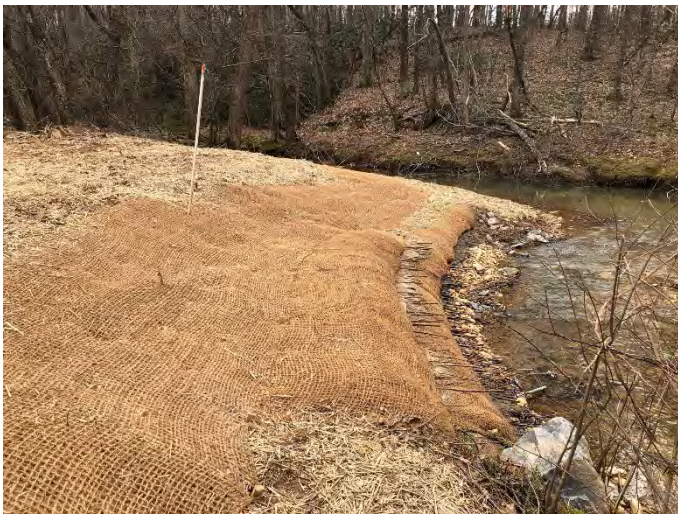
Hogan Creek Reach 1 STA 16+50 left bank repair – (3/13/2019)
