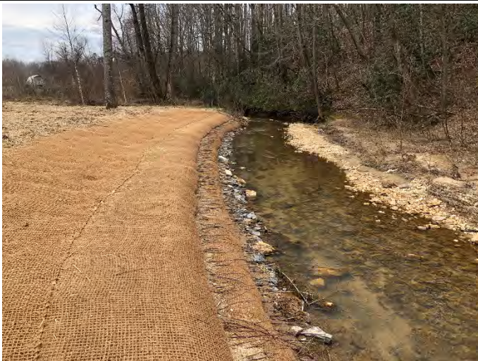
Hogan Creek Reach 1 STA 20+10 left bank repair – (3/13/2019)
