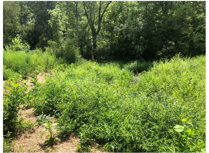
Hogan Creek Reach 1 STA 10+20 left bank and 10+80 right bank repairs – (8/19/2019)
