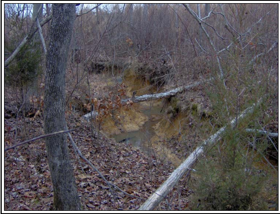
Middle Creek: Pond Outfall
