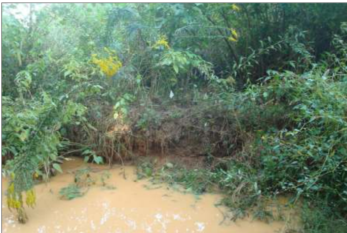
Buckhorn Creek, minor bank scour, Sta 183+40 9/26/11 Photo No. 49
