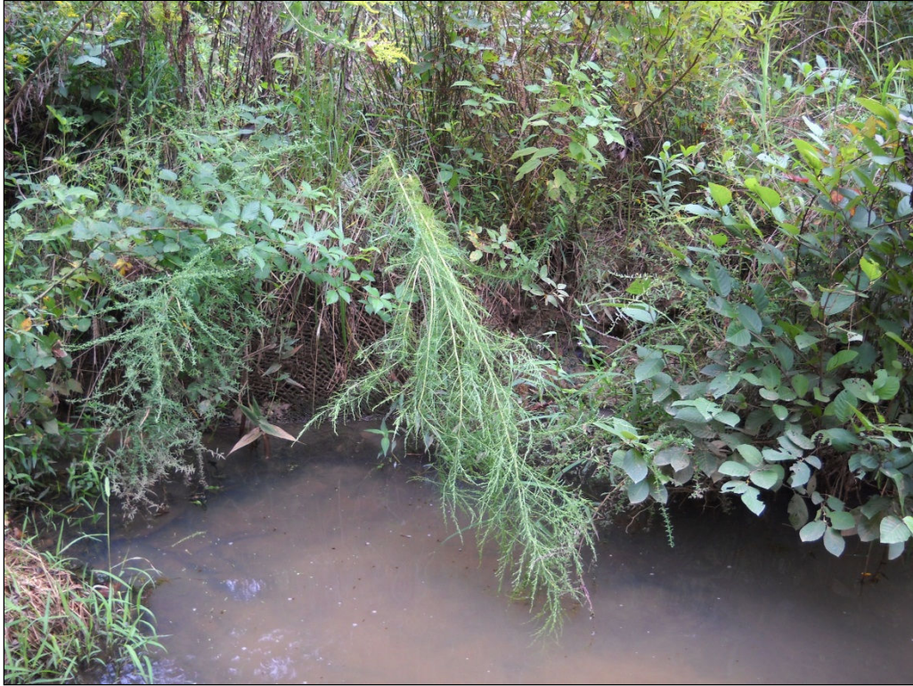
Buckhorn Creek, minor bank scour, Sta 152+90
