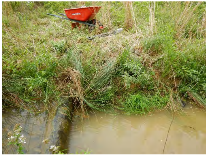
After - Repaired Localized Erosion (5/5/2020)
