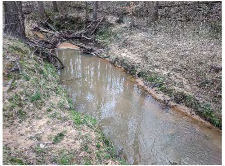
PHOTO POINT 23 UT - PHB – looking downstream (3/3/2020)
