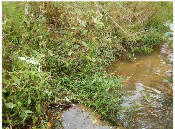
After - Repaired Localized Erosion (9/28/2020)
