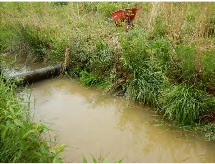
After - Repaired Localized Erosion (5/5/2020)
