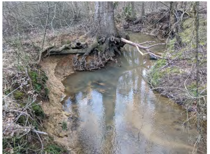
PHOTO POINT 21 UT - PHB – looking downstream (3/3/2020)
