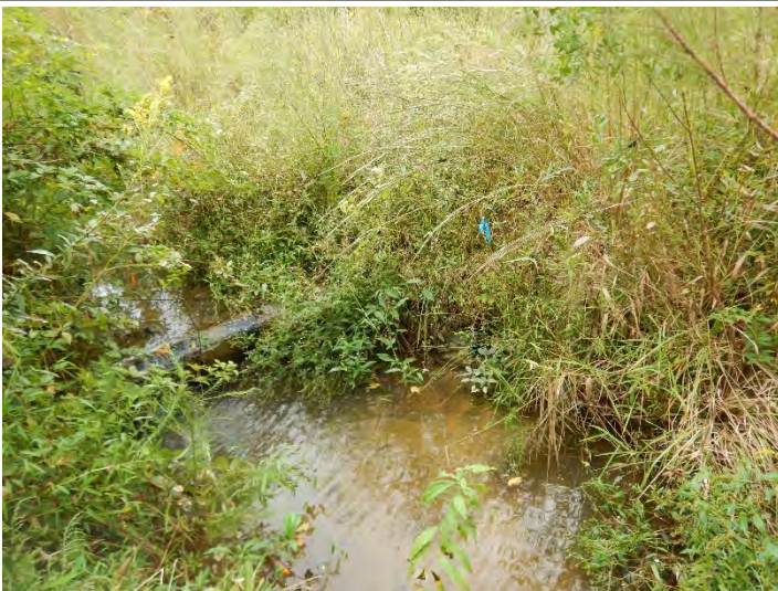
After - Repaired Localized Erosion (9/28/2020)
