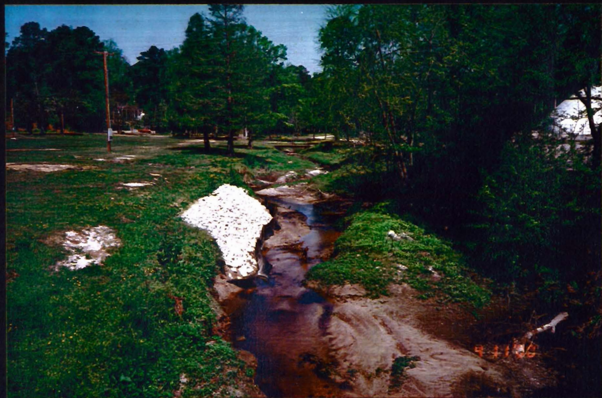
DEGRADED STREAM WITHIN WILSON RECREATION PARK
