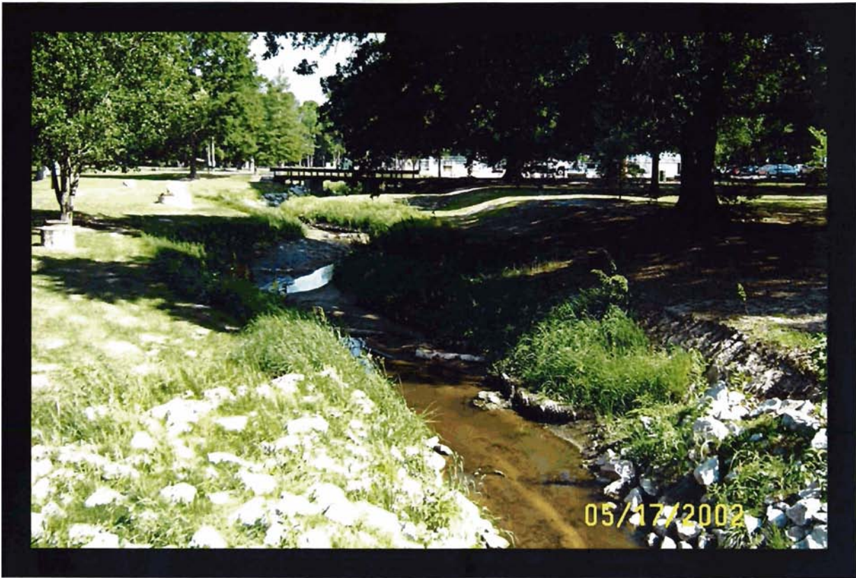
Upstream view from Photo Location #10 (on downstream railroad bridge).
