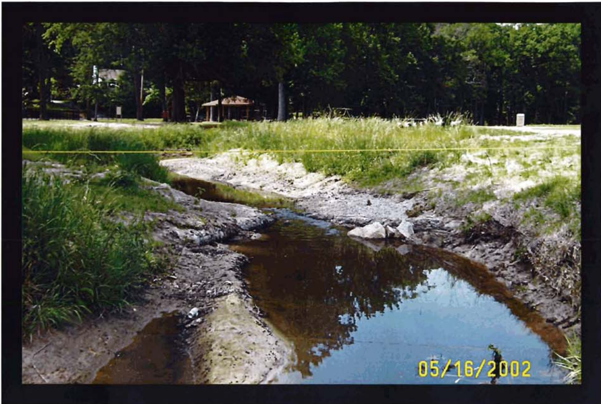
Upstream view at Cross-section #3.
