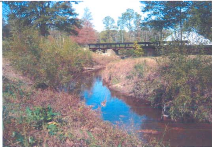
Photo of Cross-Section #4 - Looking Downstream
