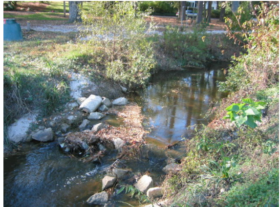
Issue Photo 3. Urban debris blockage.
