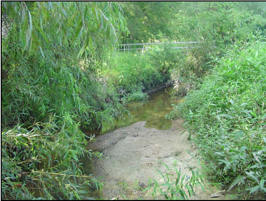
P31. Station 12+15. Aggregation.
