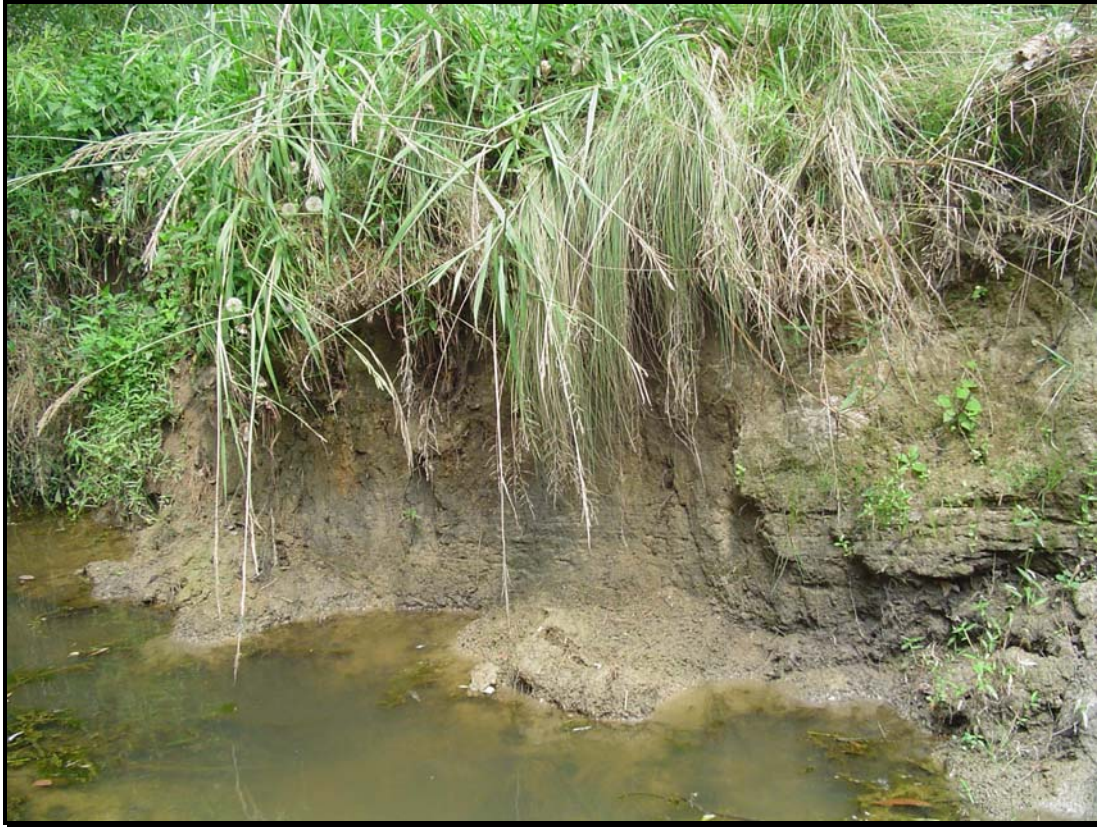
P23. Station 15+25. Erosion on left bank.
