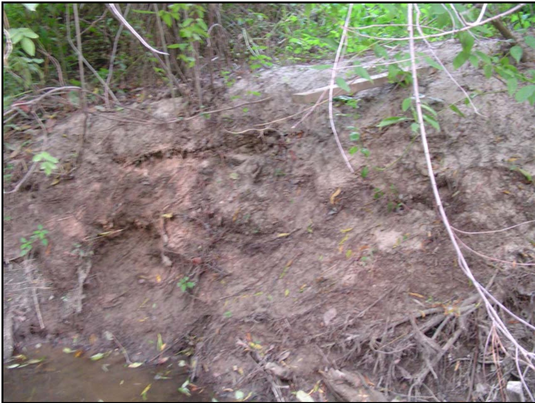
P55. Station 4+15. Erosion on left bank.
