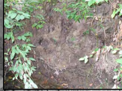
P41 - Left Bank Erosion
