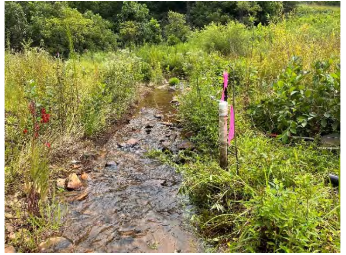
New Automated Crest Gage Location (118+10) – downstream (08/17/2022)
