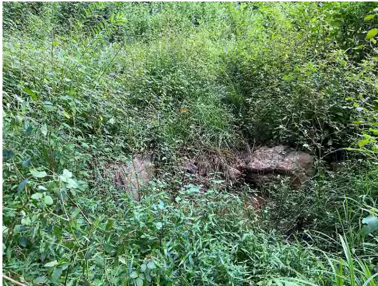
UT6 BMP photo– upstream (08/16/2022)
