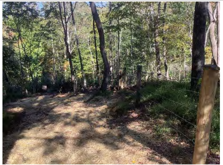
UT5 Fence Repair– (09/30/2022)
