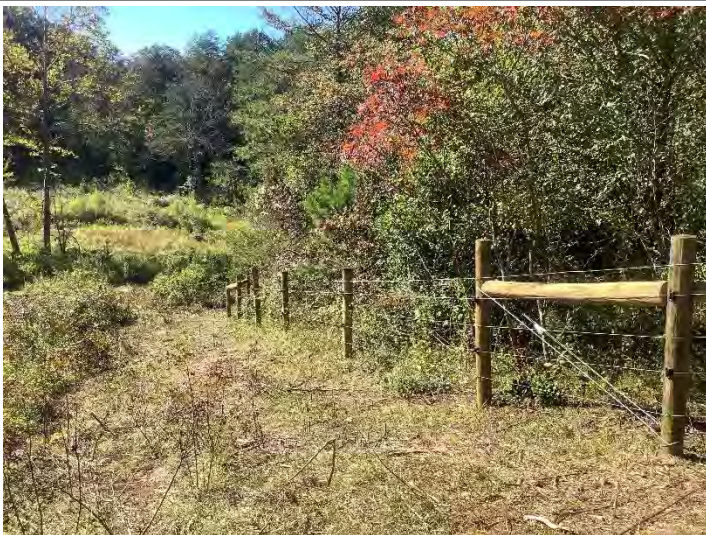
New Easement Fence Installed on Field Adjacent to Venable Creek R4– (09/30/2022)
