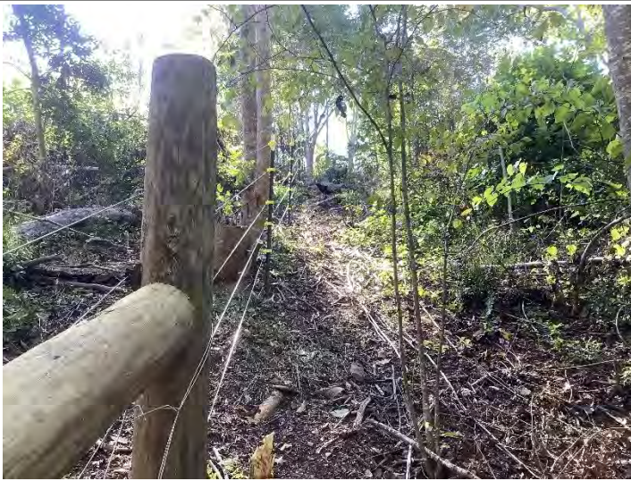
UT5 Fence Repair– (09/30/2022)
