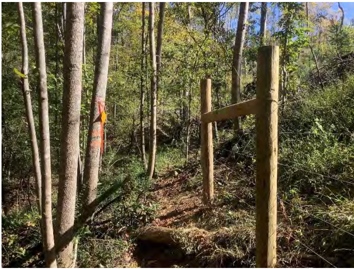
UT2 Fence Repair– (09/30/2022)
