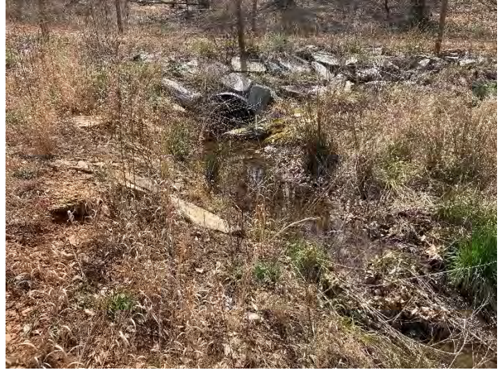
UT2 Crossing Culvert – Outlet (03/23/2023)
