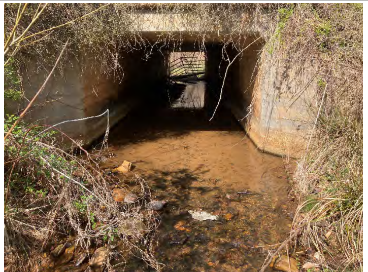
UT1 Culvert – Outlet (03/23/2023)
