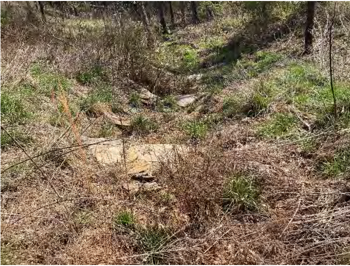
UT3 BMP – Looking Downstream (03/23/2023)
