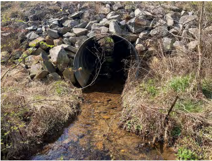
Venable Creek R1 Culvert – Outlet (03/23/2023)
