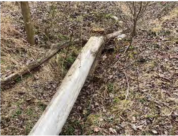
PHOTO POINT 8 UT2 R1 Headcut – upstream (03/23/2023)
