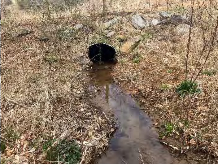
UT2 Crossing Culvert – Inlet (03/23/2023)
