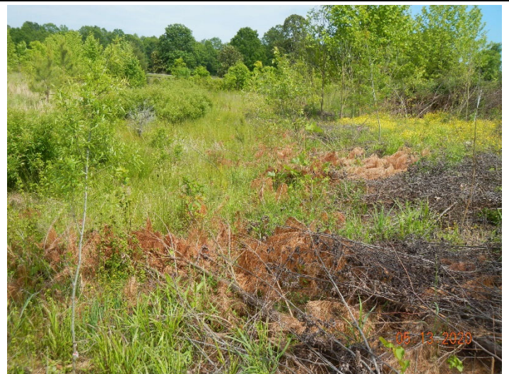
Left hillside at Station 303+50 – looking upstream (05/13/2020)
