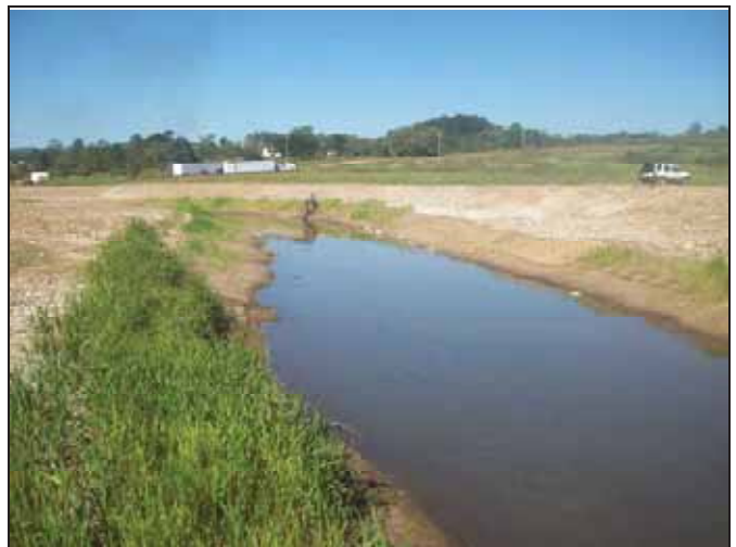
South Muddy Creek PID 18 – Constructed Riffle
