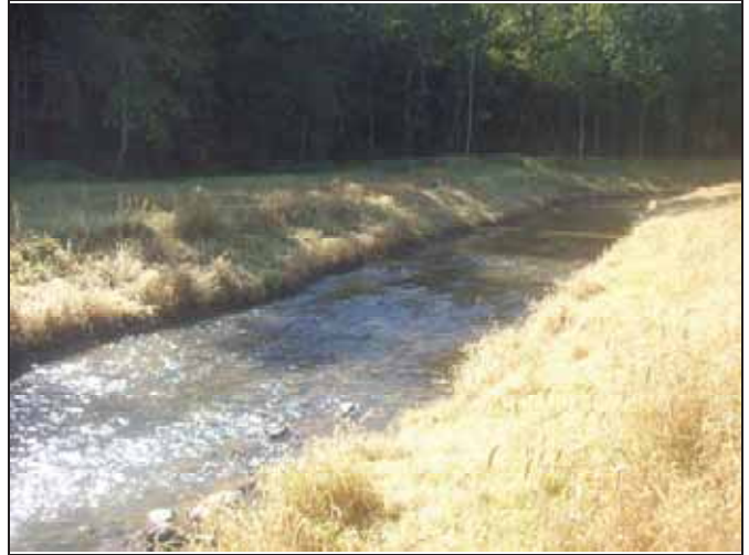
South Muddy Creek PID 2 –Constructed Riffle,
