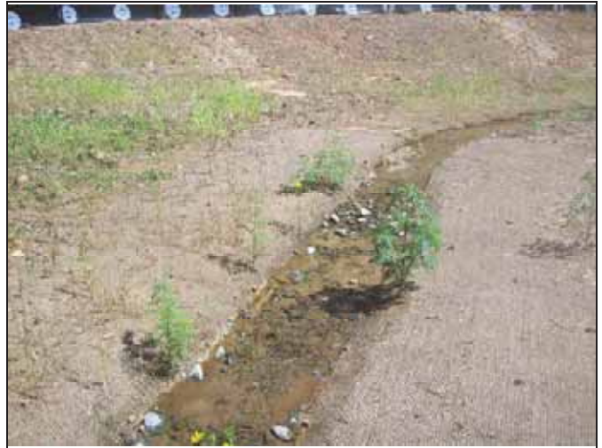
UT1 PID 8 – Constructed Riffle
