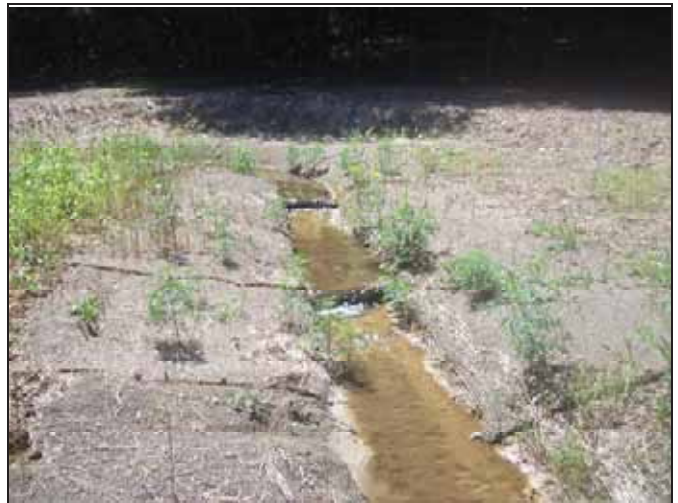
UT1 PID 10 – Log Sills
