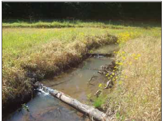
SFHC PID 6 – Log Sills and Root Wad
