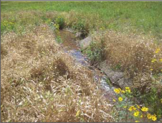
UT1 PID 19 – Constructed Riffle
