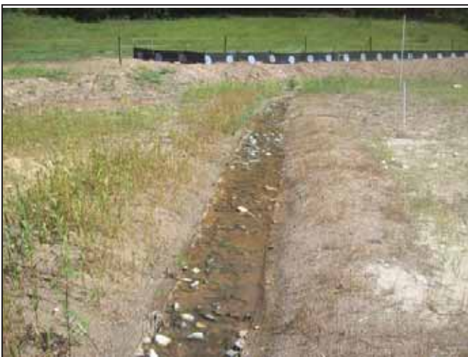
UT1 PID 11 – Constructed Riffle
