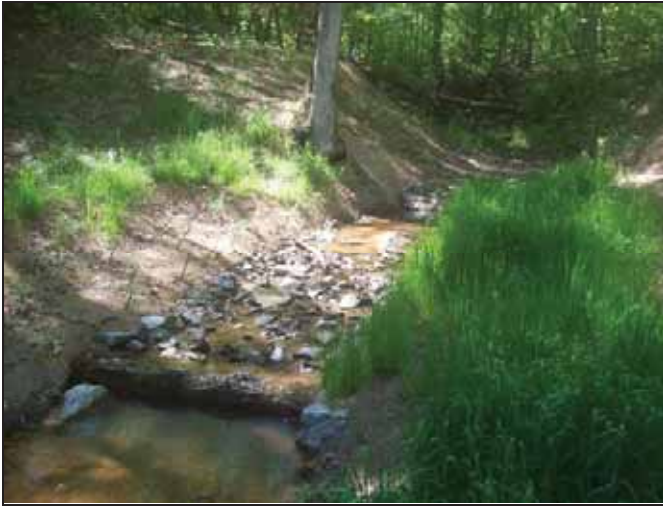
UT2 PID 1 – Constructed Riffle & Log Sill
