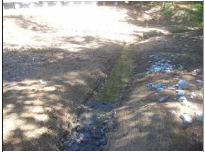
UT1 PID 2 – Constructed Riffle
