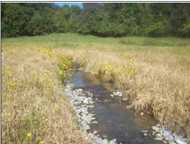
SFHC PID 5 – Constructed Riffle
