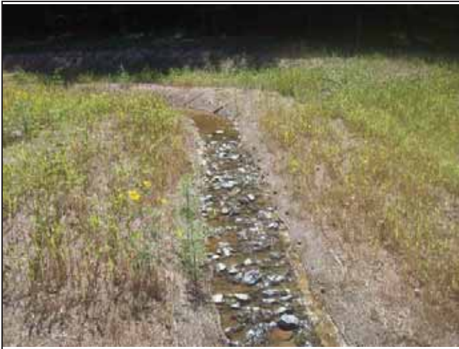
UT1 PID 13 – Constructed Riffle
