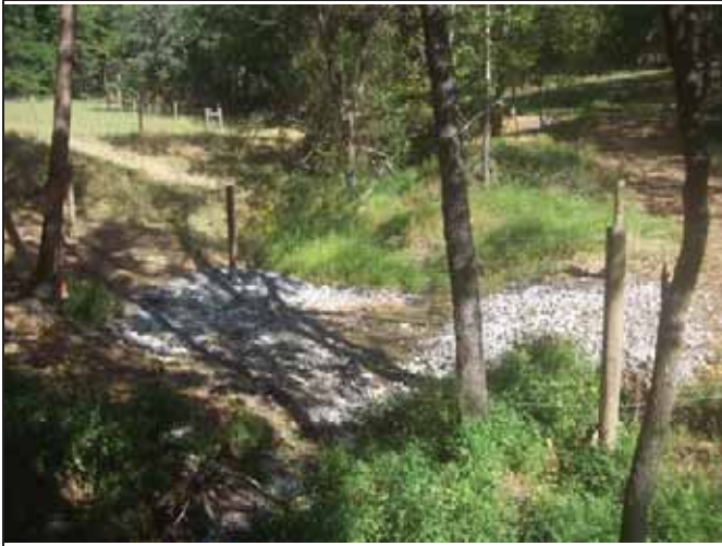
UT2 PID 3 – Stream crossing
