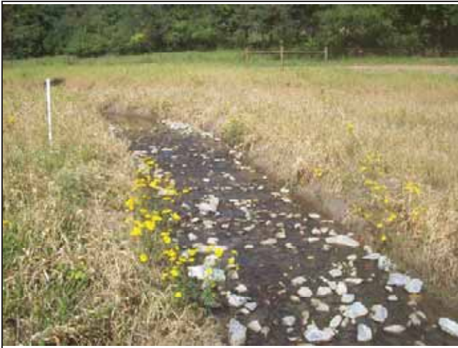
SFHC PID 7 – Constructed Riffle
