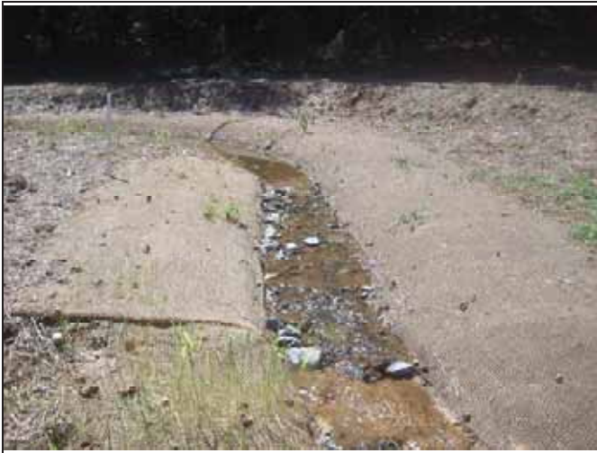
UT1 PID 7 – Constructed Riffle
