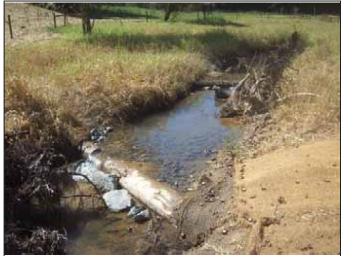
SFHC PID 14 – Log Sills & Root Wad
