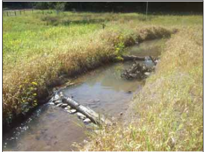
SFHC PID 8 – Log Sills & Root Wad
