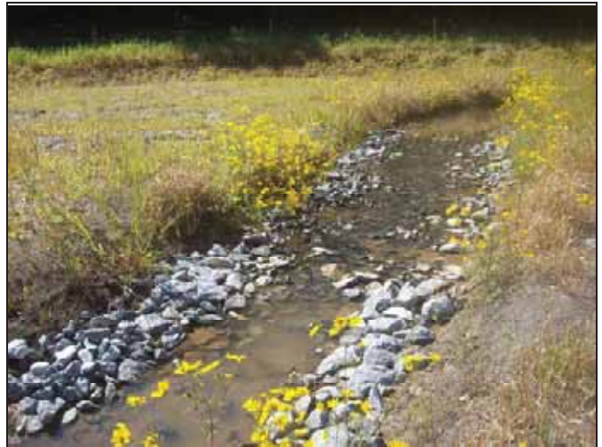
SFHC PID 4 – Constructed Riffle
