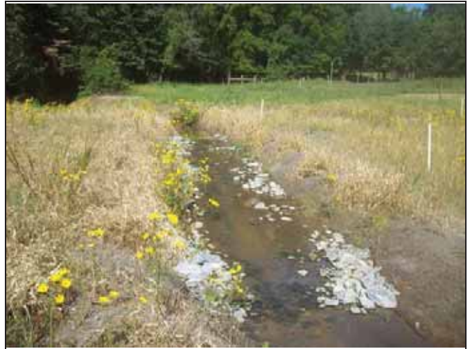
SFHC PID 2 – Constructed Riffle
