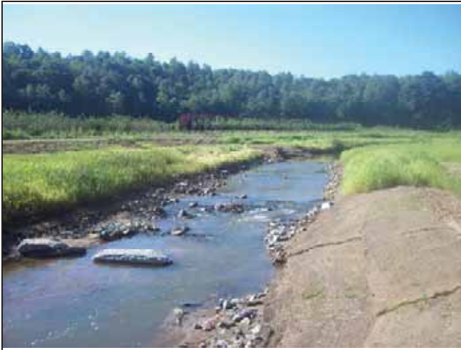
South Muddy Creek PID 13 – Constructed Riffle
