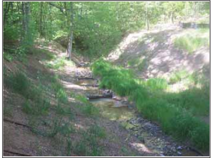
UT2 PID 2 – Constructed Riffles & Log Sills
