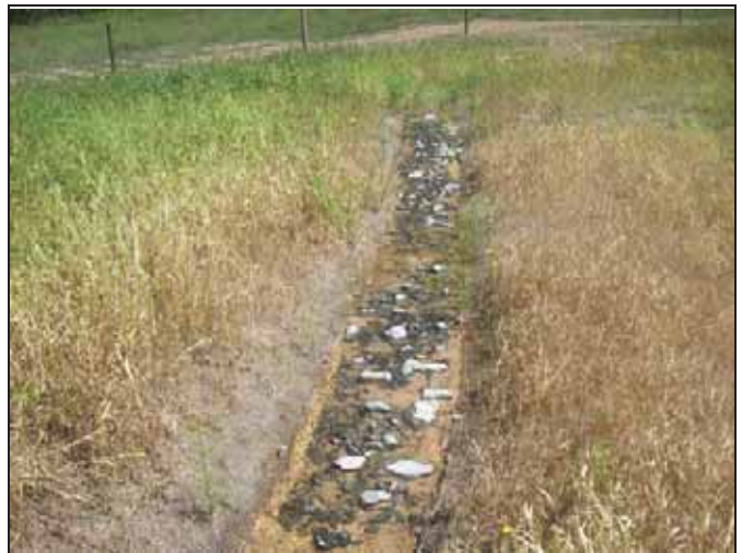
UT1 PID 16 – Constructed Riffle
