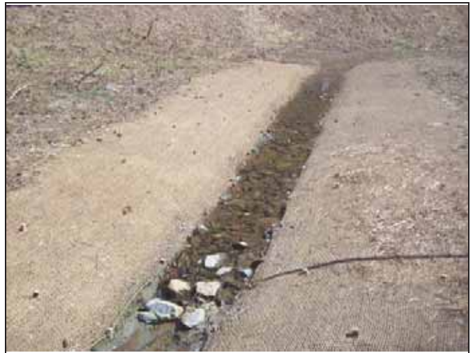
UT1 PID 4 – Constructed Riffle
