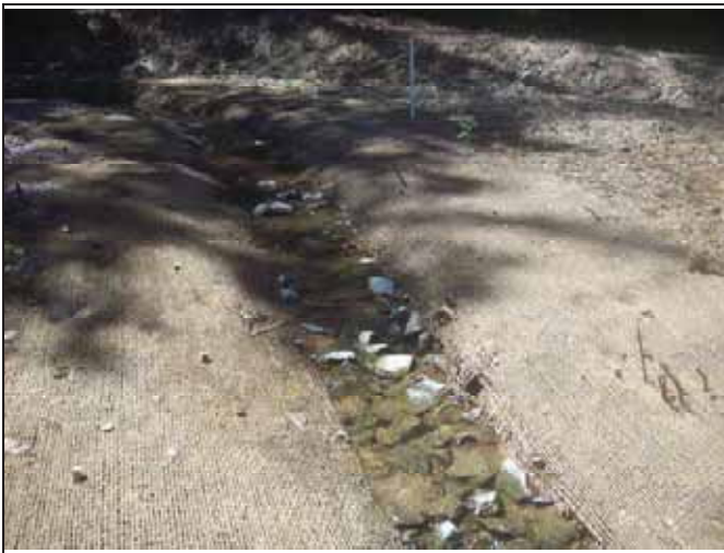
UT1 PID 3 – Constructed Riffle
