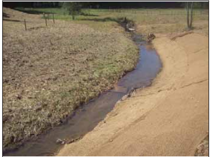
SFHC PID 16 – Log Vane & Matted Bank
