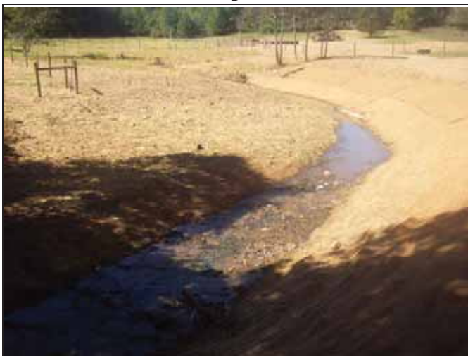
SFHC PID 17 – Constructed Riffle at downstream terminus of project
