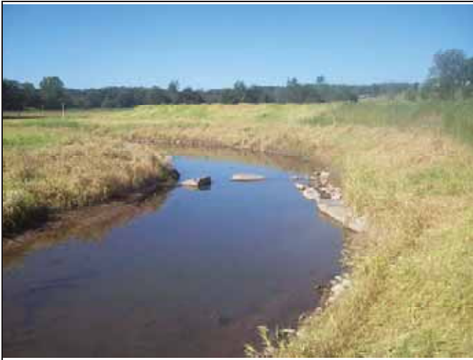
South Muddy Creek PID 7 – J-Hook in Meander
