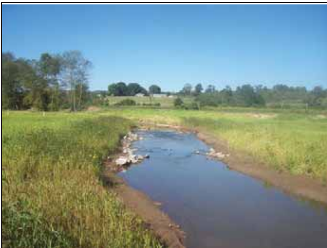
South Muddy Creek PID 11 – Constructed Riffle
