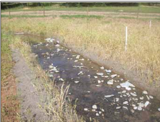
SFHC PID 9 – Constructed Riffle
