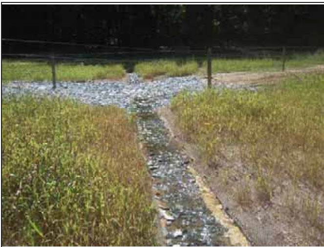
UT1 PID 15 – Constructed Riffle below stream crossing
