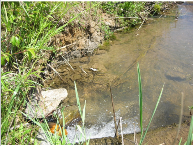
SPA1 – SFHC Reach 1 Left bank scour
