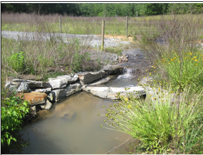
SPA3 – SFHC Reach 2 Piping of cross vane
