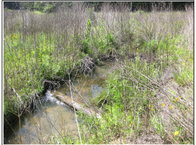
SFHC PID 8 – Log Sills & Root Wad
