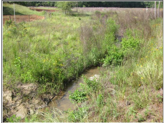
SFHC PID 16 – Log Vane & Matted Bank
