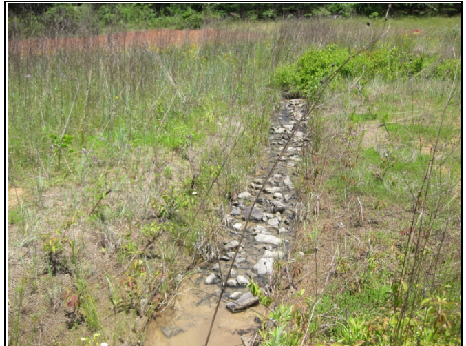
UT1 PID 16 – Constructed Riffle
