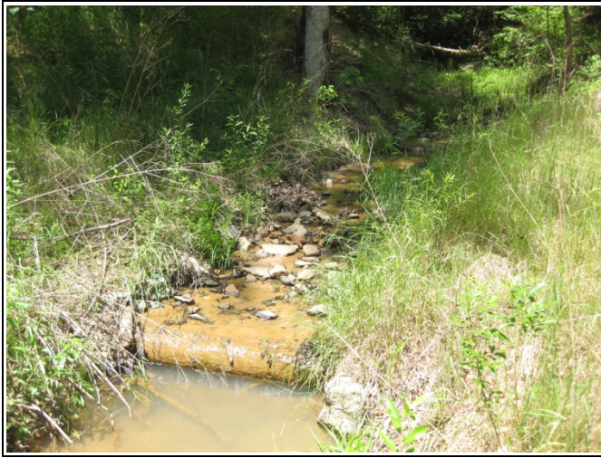
UT2 PID 1 – Constructed Riffle & Log Sill
