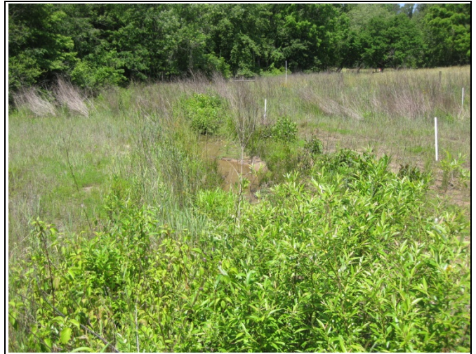
SFHC PID 2 – Constructed Riffle
