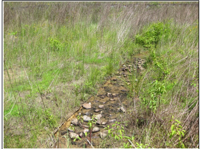
UT1 PID 8 – Constructed Riffle
