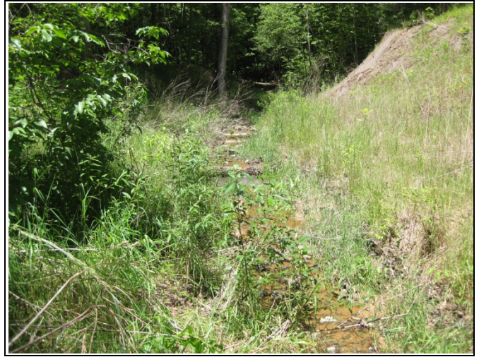
UT2 PID 2 – Constructed Riffles & Log Sills
