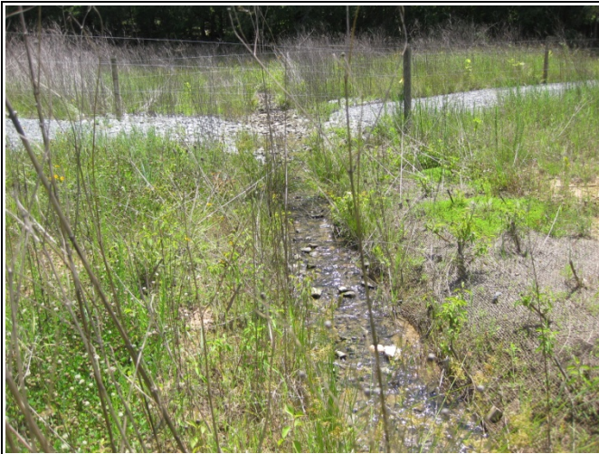
UT1 PID 15 – Constructed Riffle below stream crossing
