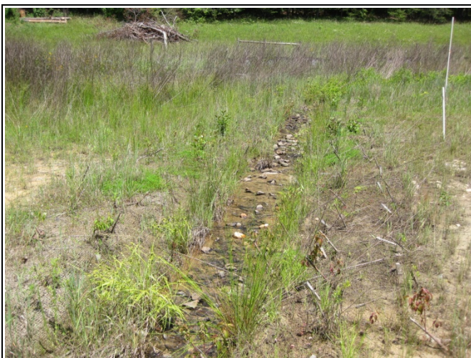
UT1 PID 11 – Constructed Riffle
