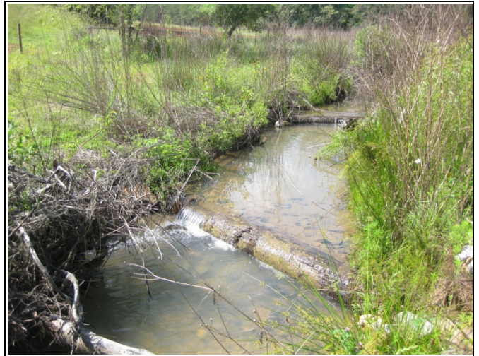
SFHC PID 14 – Log Sills & Root Wad
