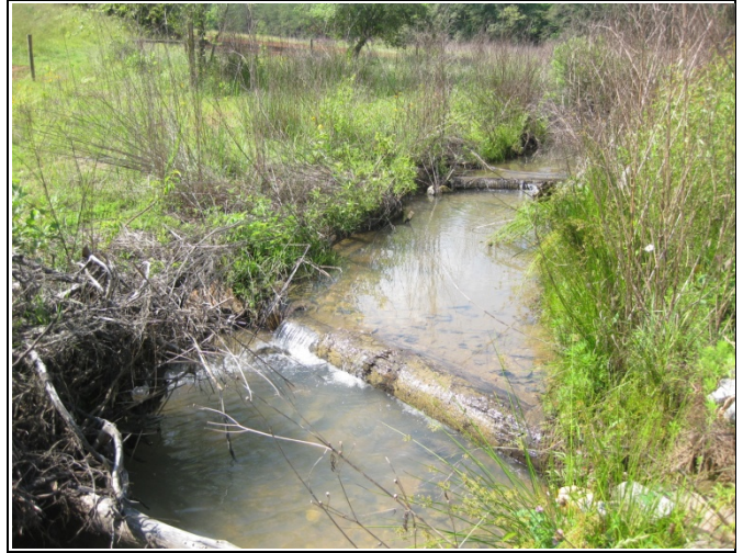
SFHC PID 14 – Log Sills & Root Wad
