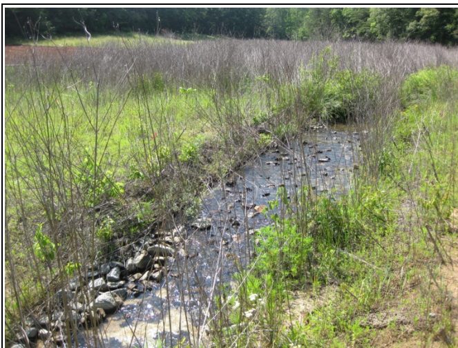
SFHC PID 11 – Constructed Riffle
