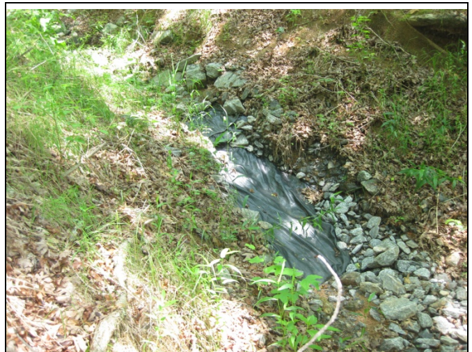
SPA 6 – Ephemeral drainage channel bed erosion
