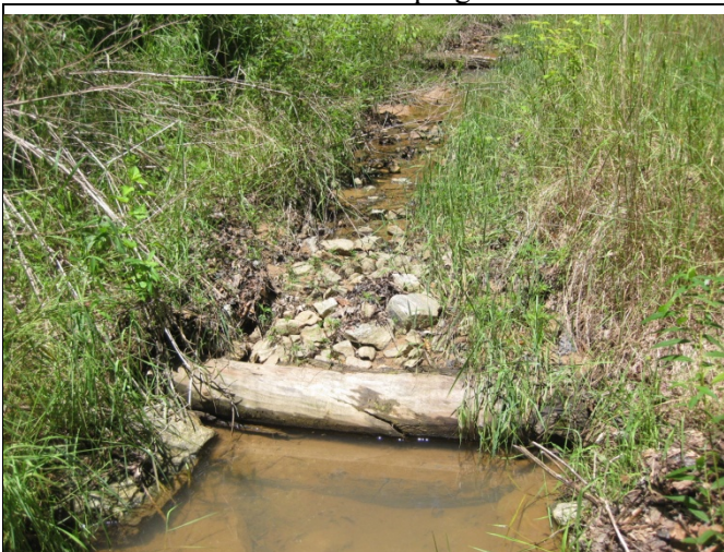
SPA5 – UT2 Reach A Piping within riffle cascade around log sill
