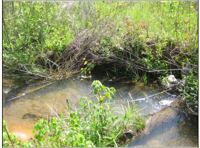
SPA2 – SFHC Reach 1 Right bank scour
