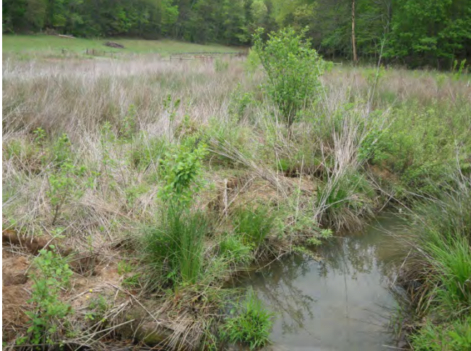
SPA2-2 – SFHC Reach 1 Right bank slumping
