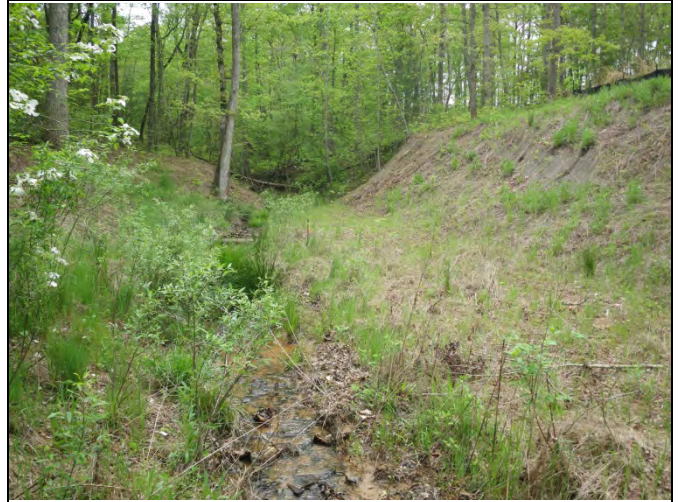
UT2 PID 2 – Constructed Riffles & Log Sills
