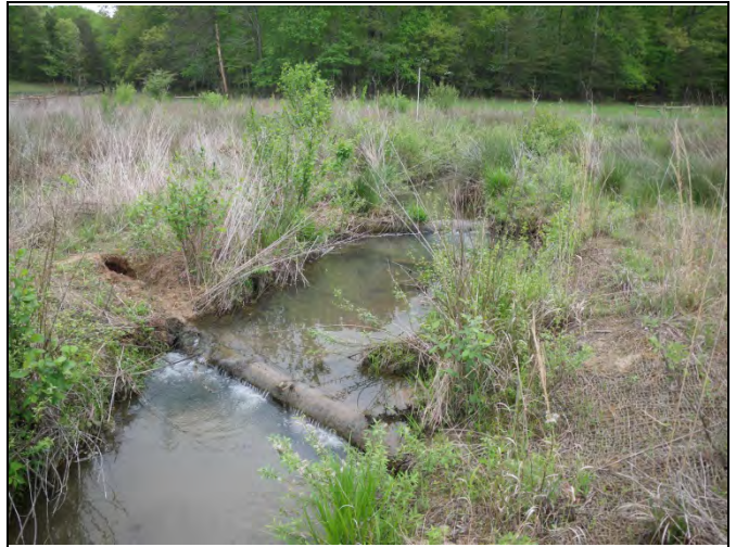
SFHC PID 8 – Log Sills & Root Wad
