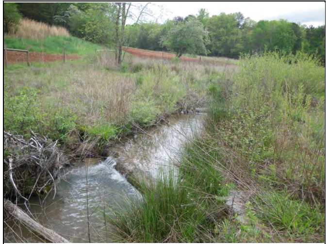
SFHC PID 14 – Log Sills & Root Wad
