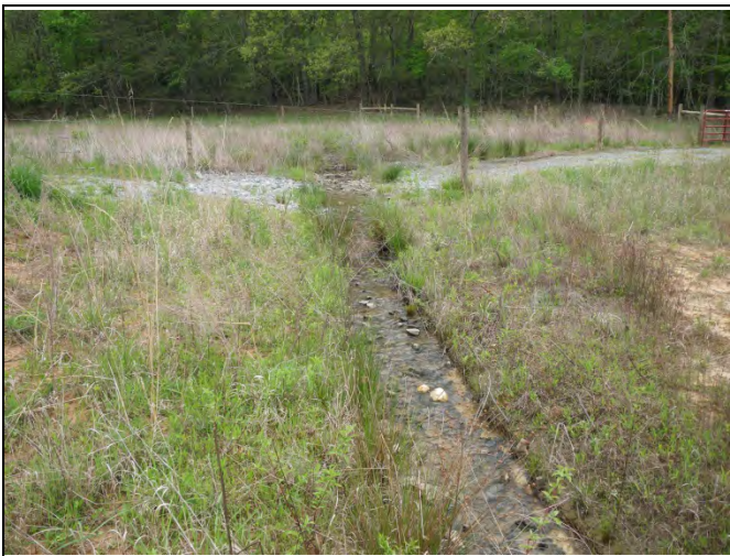
UT1 PID 15 – Constructed Riffle below stream crossing
