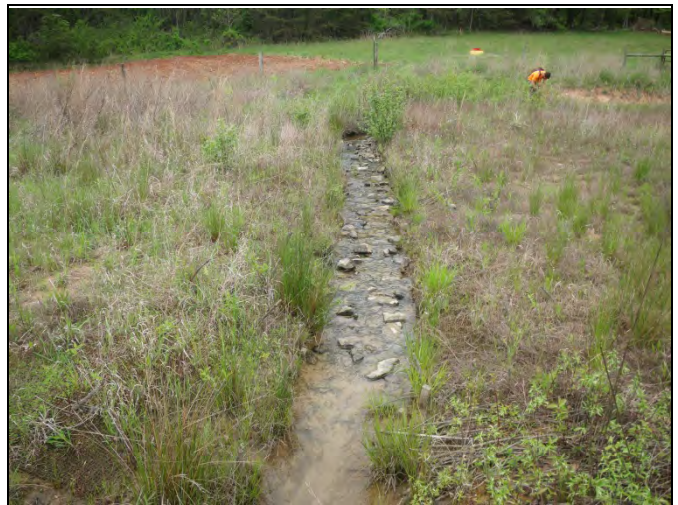
UT1 PID 16 – Constructed Riffle
