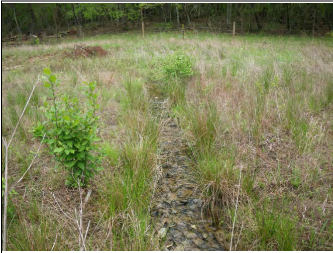
UT1 PID 13 – Constructed Riffle
