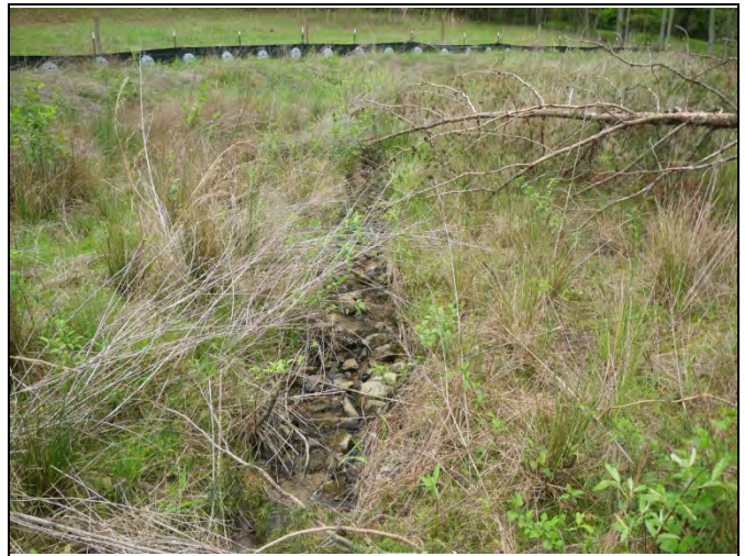
UT1 PID 4 – Constructed Riffle
