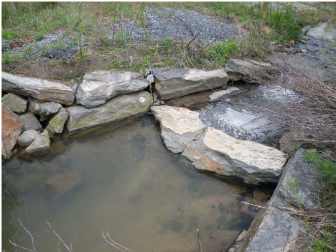
SPA1-3 – SFHC Reach 2 Piping of cross vane
