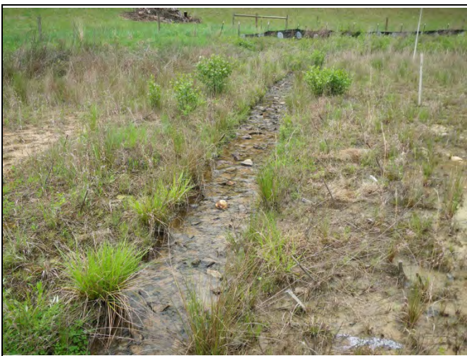
UT1 PID 11 – Constructed Riffle
