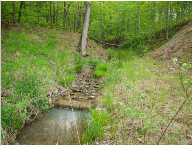
UT2 PID 1 – Constructed Riffle & Log Sill
