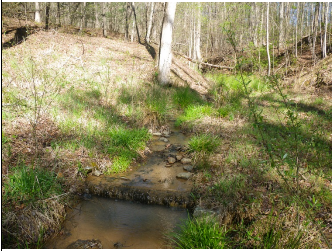
UT2 PID 1 – Constructed Riffle & Log Sill
