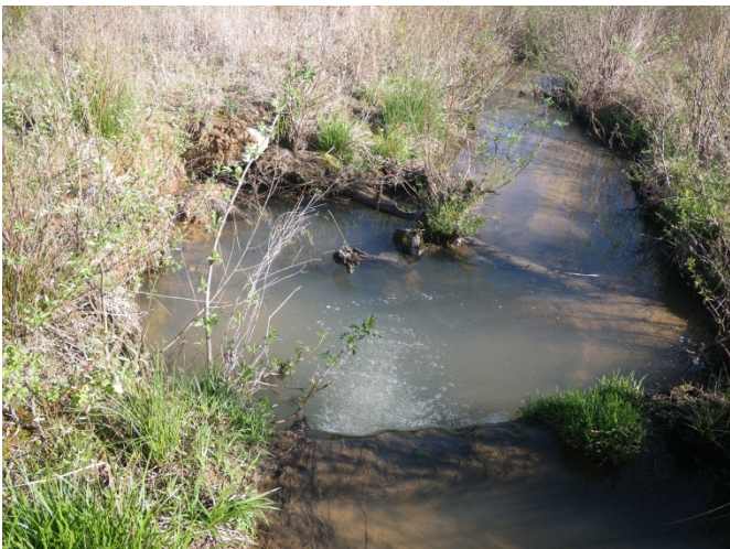
SPA2-1 – SFHC Reach 1 Rootwad failure along left bank due to undercutting along bank
