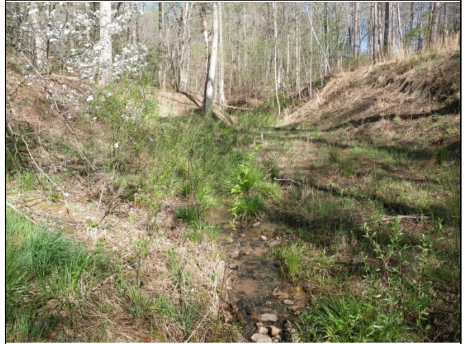
UT2 PID 2 – Constructed Riffles & Log Sills
