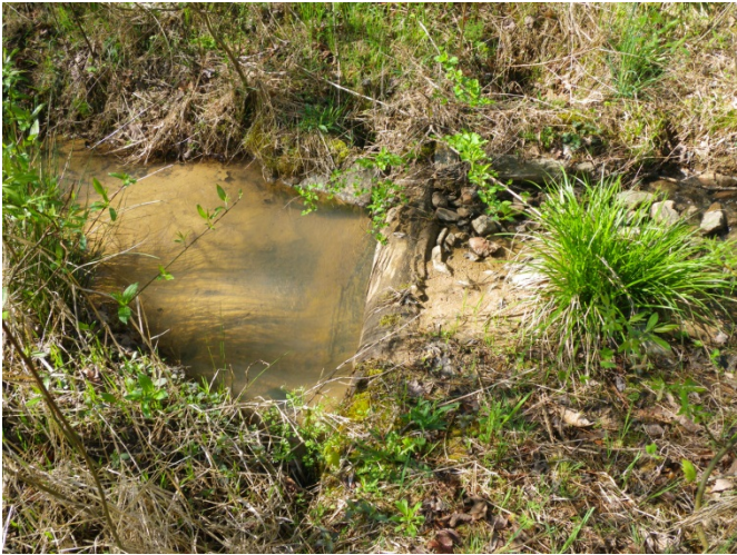
SPA1-5 – UT2 Reach A Piping within riffle cascade around log sill
