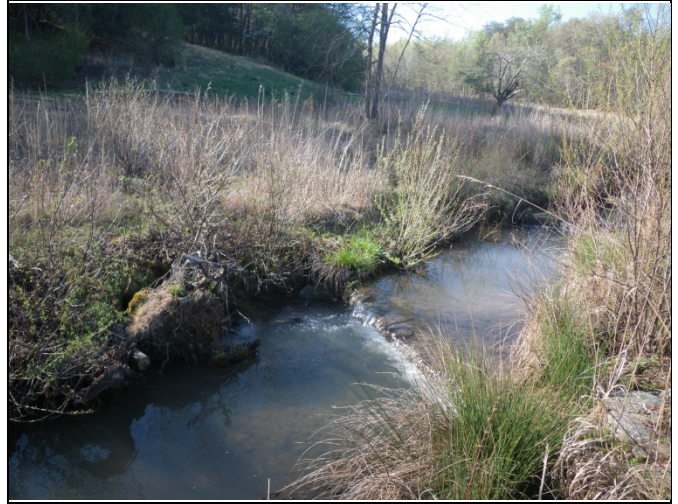
SFHC PID 14 – Log Sills & Root Wad
