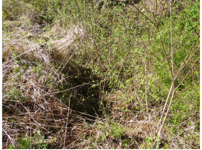
SPA2-4 – UT2 Reach B Left bank slumping
