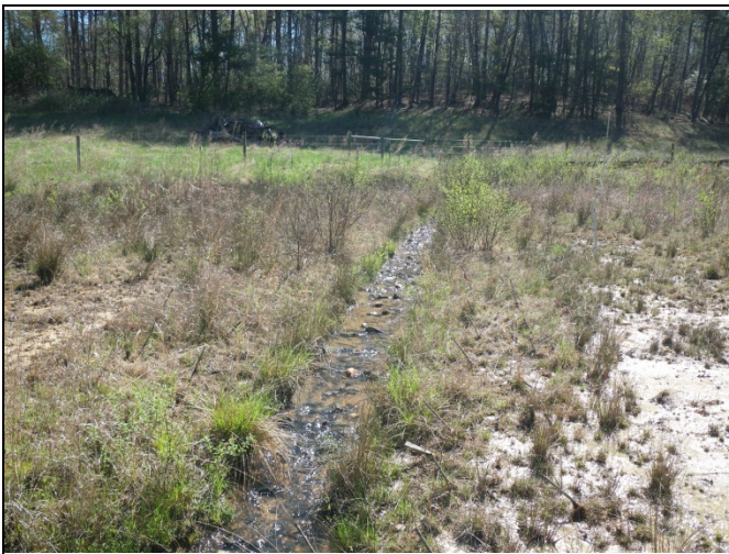
UT1 PID 11 – Constructed Riffle
