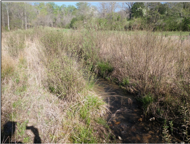
SFHC PID 5 – Constructed Riffle
