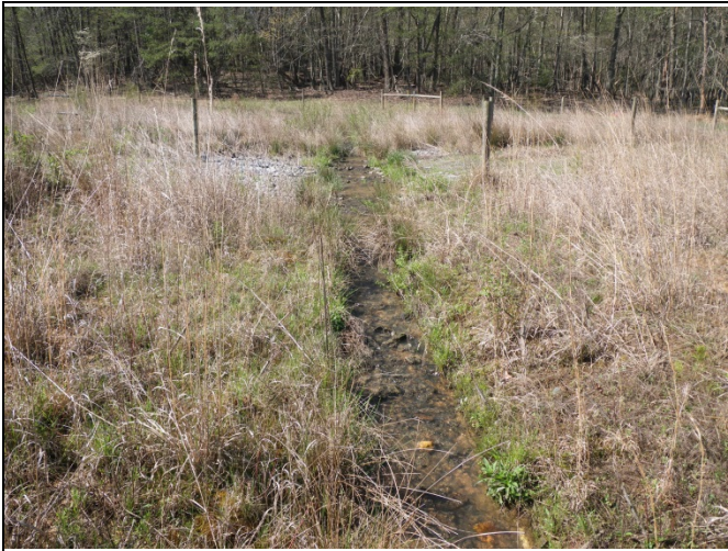
UT1 PID 15 – Constructed Riffle below stream crossing
