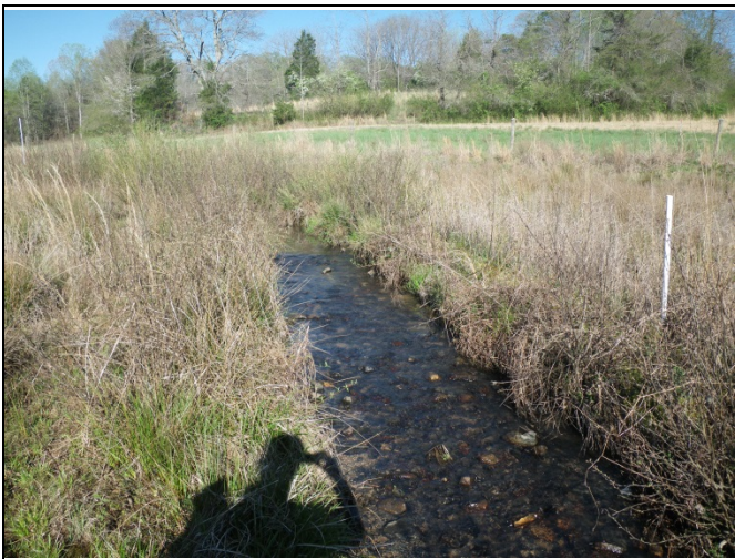
SFHC PID 9 – Constructed Riffle
