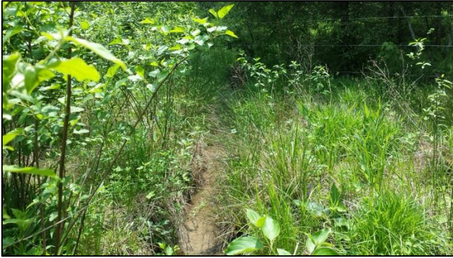
UT1 PID 1 – Constructed riffle
