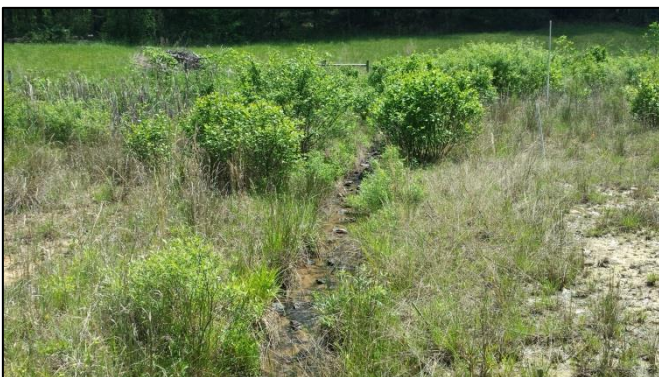
UT1 PID 11 – Constructed riffle
