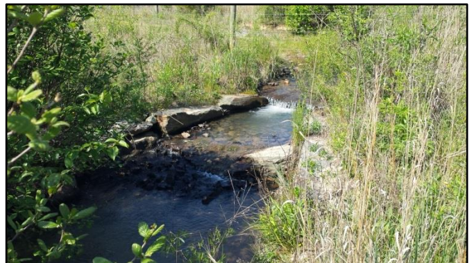
SFHC PID 12 – Double drop cross vane below crossing
