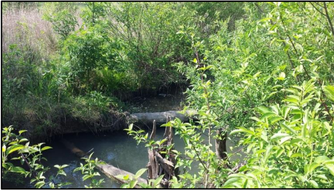
SFHC PID 13 – Log sills & root wad
