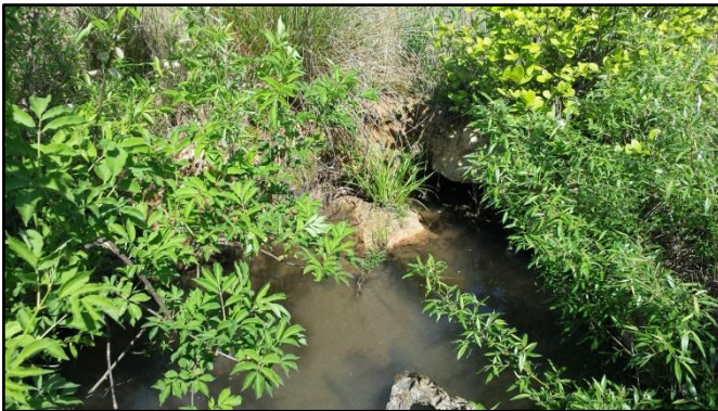
SPA2-1 – SFHC Reach 1: Rootwad failure along left bank due to undercutting along bank.
