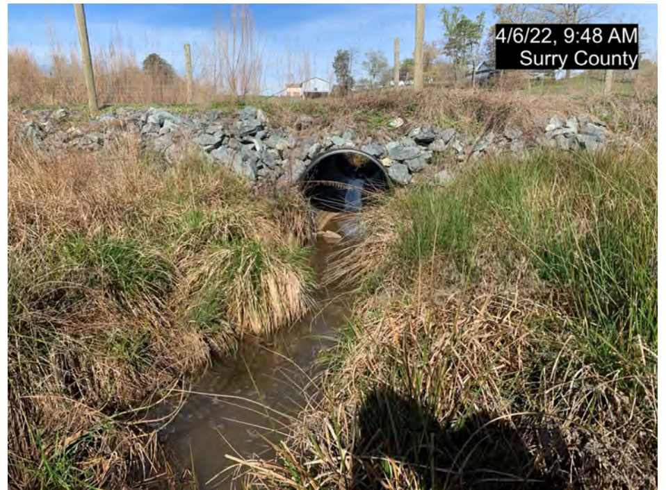
PS-1, R1, Culvert Crossing, Upstream (MY-03)
