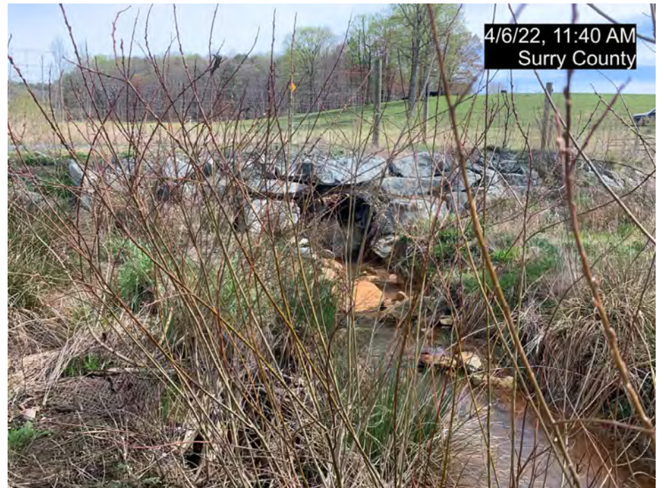
PS-6, R5, Culvert Crossing, Upstream (MY-03)
