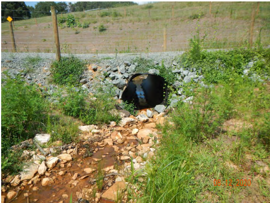
PS-2, R2, Culvert Crossing, Downstream (MY-00)
