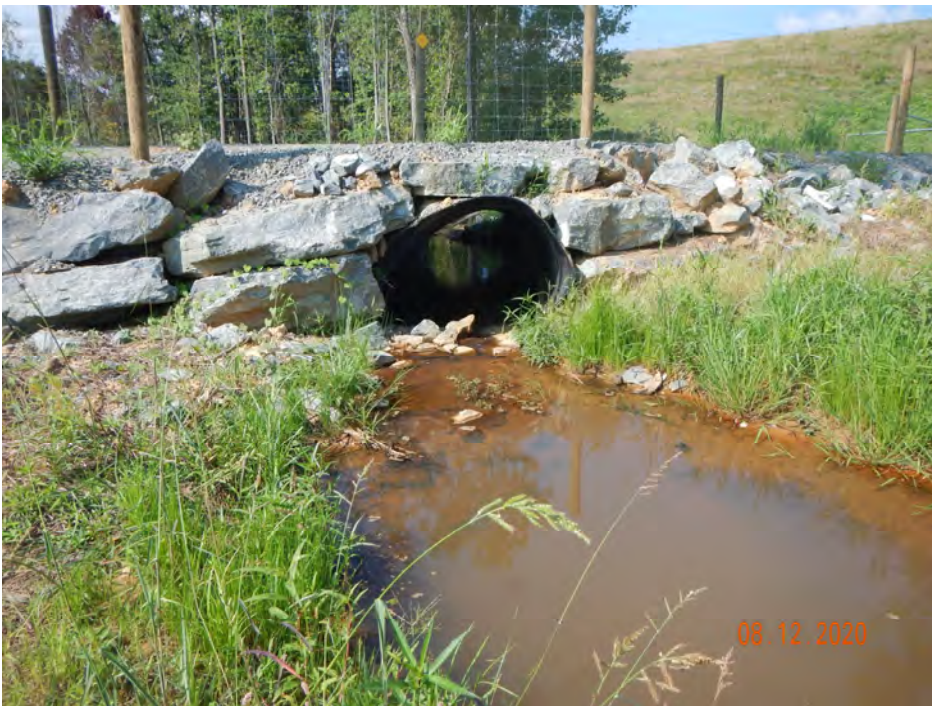
PS-6, R5, Culvert Crossing, Downstream (MY-00)
