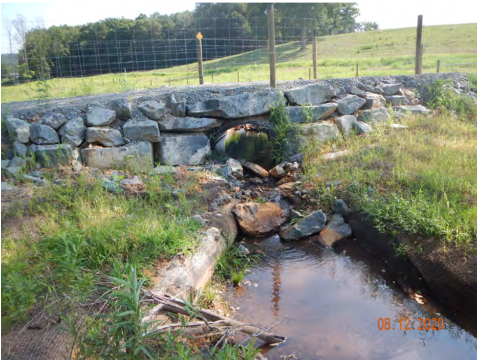
PS-6, R5, Culvert Crossing, Upstream (MY-00)
