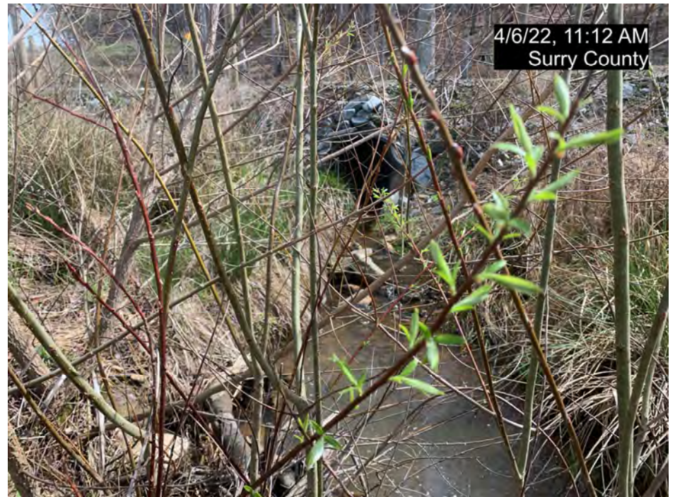
PS-3, R4, Culvert Crossing, Upstream (MY-03)
