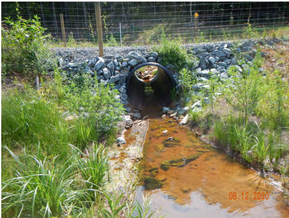
PS-2, R2 Culvert Crossing, Upstream (MY-00)
