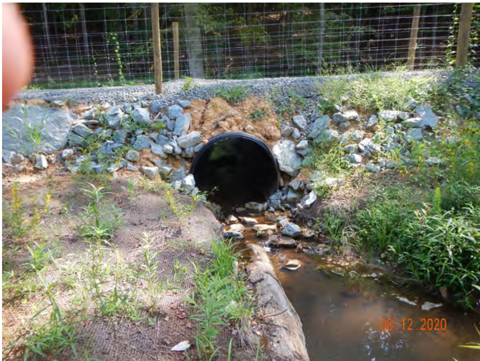
PS-3, R4, Culvert Crossing, Upstream (MY-00)
