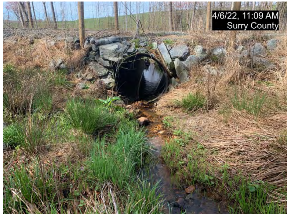
PS-3, R4, Culvert Crossing, Downstream (MY-03)
