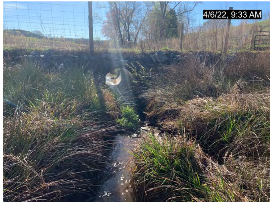
PS-1, R1, Culvert Crossing, Downstream (MY-03)
