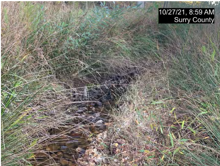
SPA8, R4, STA 20+75, Channel Bed Erosion (MY-02)
