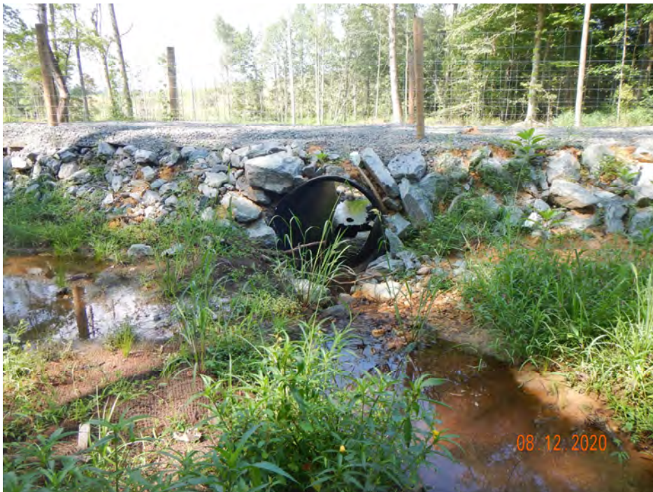
PS-3, R4, Culvert Crossing, Downstream (MY-00)
