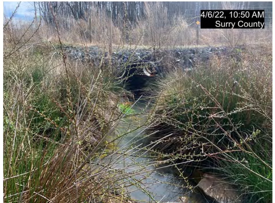
PS-2, R2, Culvert Crossing, Upstream (MY-03)
