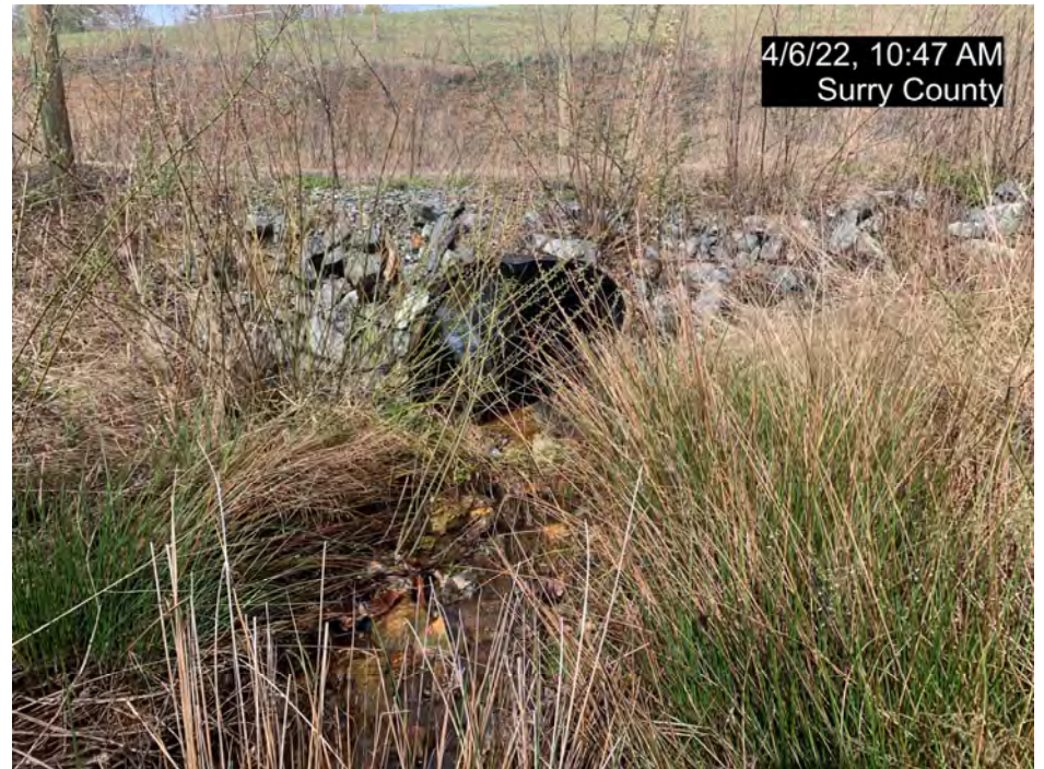
PS-2, R2, Culvert Crossing, Downstream (MY-03)
