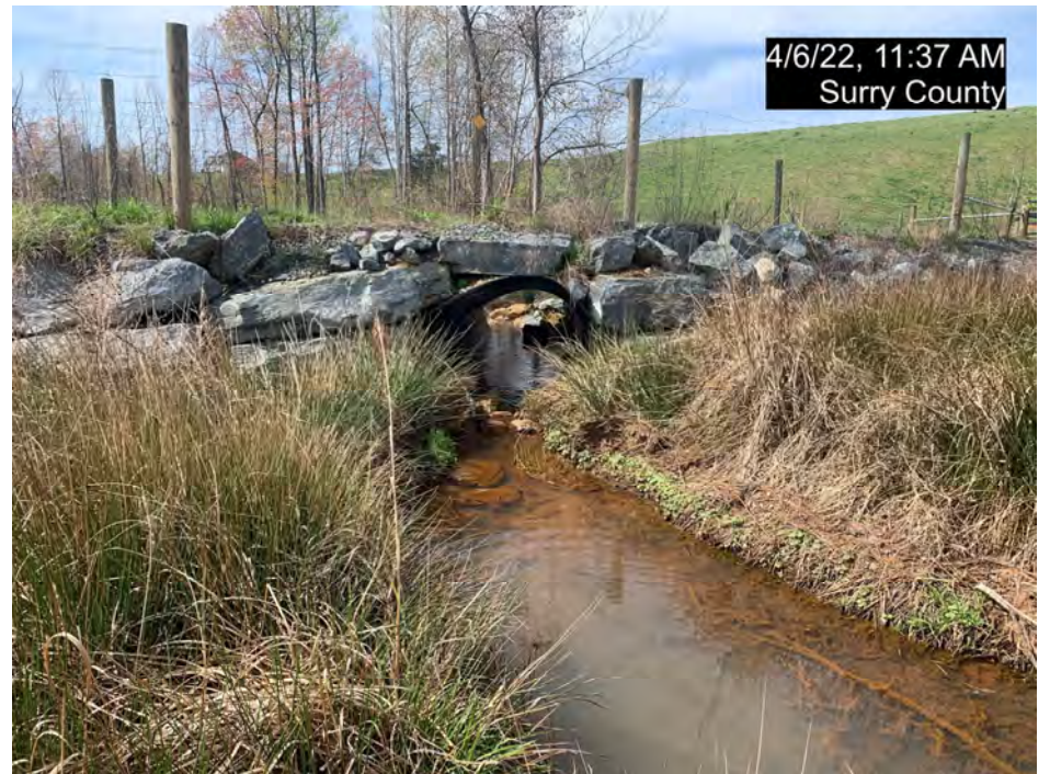
PS-6, R5, Culvert Crossing, Downstream (MY-03)
