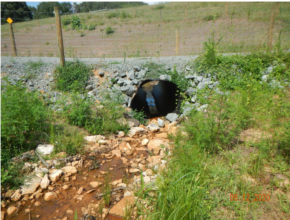
PS-2, R2, Culvert Crossing, Downstream (MY-00)
