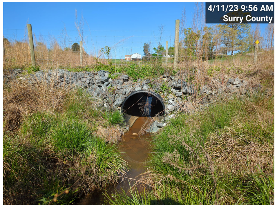
PS-1, R1, Culvert Crossing, Upstream (MY-04)
