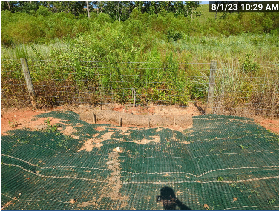
SPA5, R5 Side Slope, After repair (MY-04)
