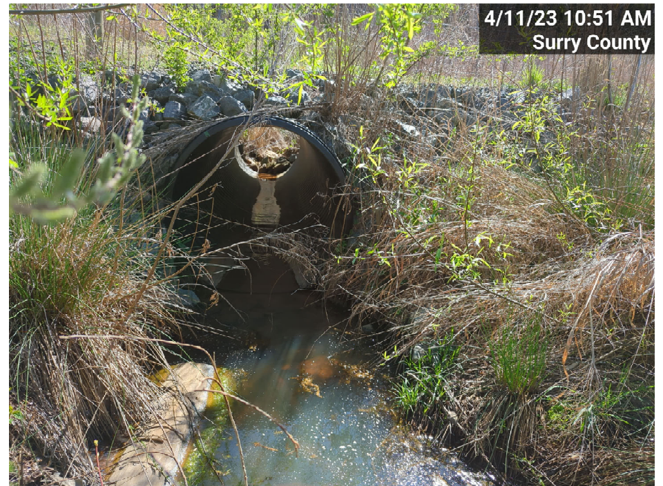
PS-2, R2, Culvert Crossing, Upstream (MY-04)
