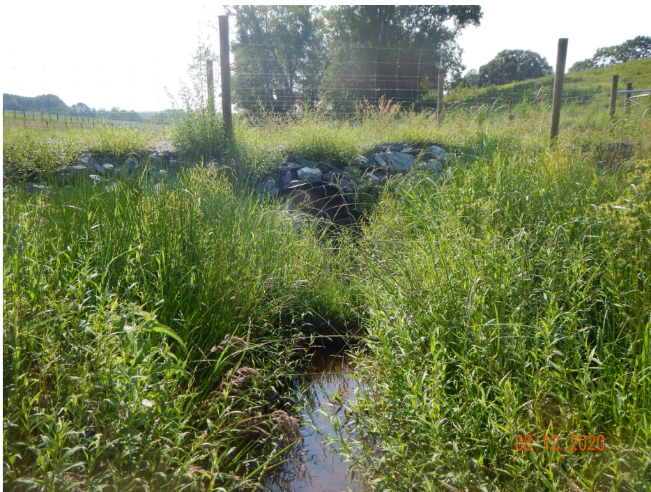
PS-1, R1, Culvert Crossing, Downstream (MY-00)
