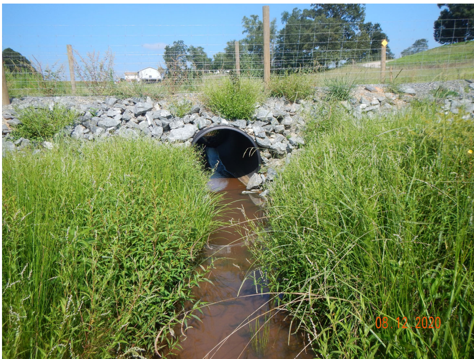
PS-1, R1, Culvert Crossing, Upstream (MY-00)
