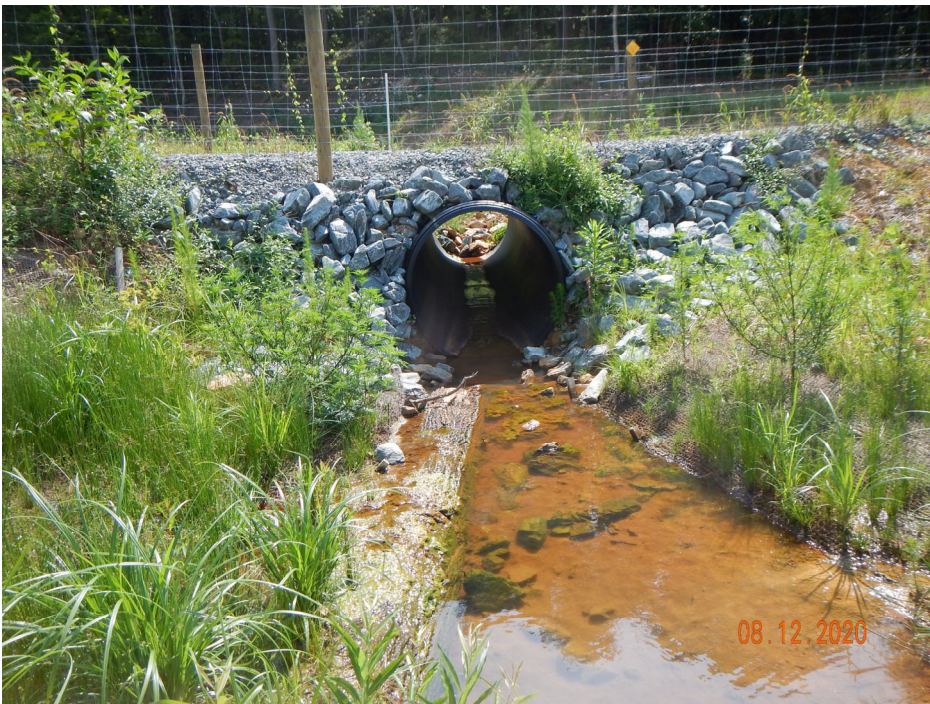
PS-2, R2 Culvert Crossing, Upstream (MY-00)
