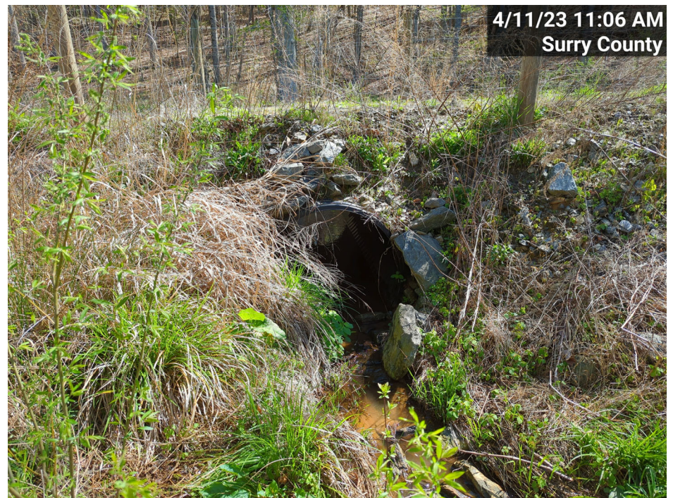
PS-3, R4, Culvert Crossing, Upstream (MY-04)
