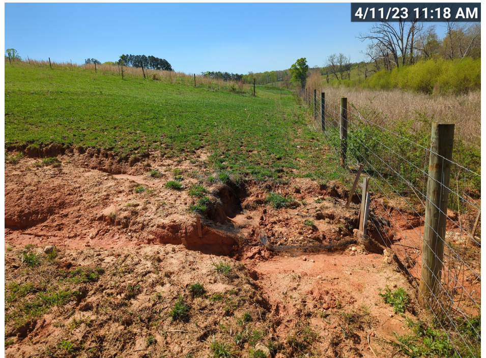
SPA5, R5 Side Slope, Minor deposition and erosion as a result of erosion outside of the easement (MY-04)
