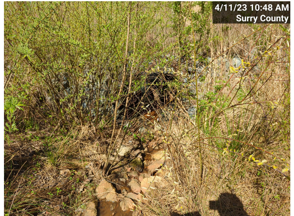
PS-2, R2, Culvert Crossing, Downstream (MY-04)
