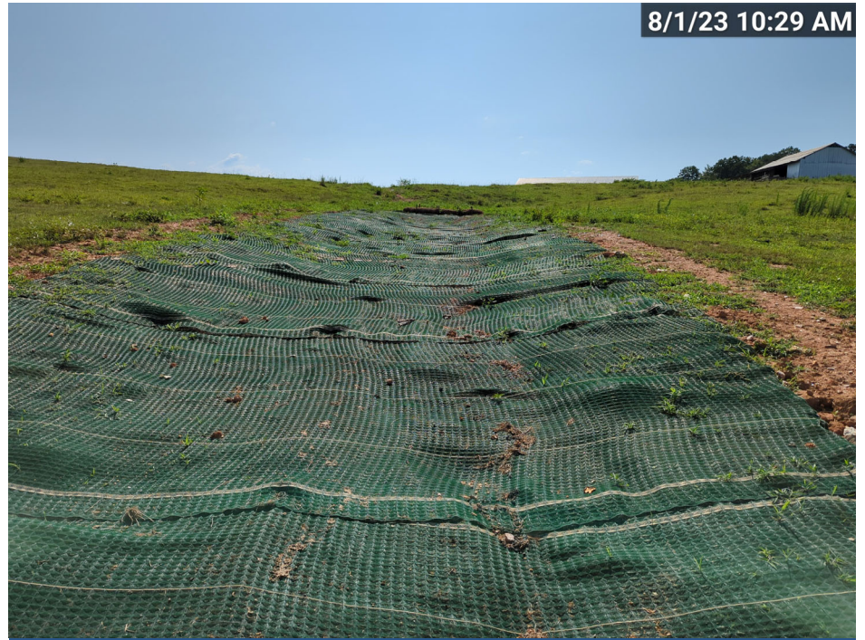
SPA5, R5 Side Slope, After repair (MY-04)
