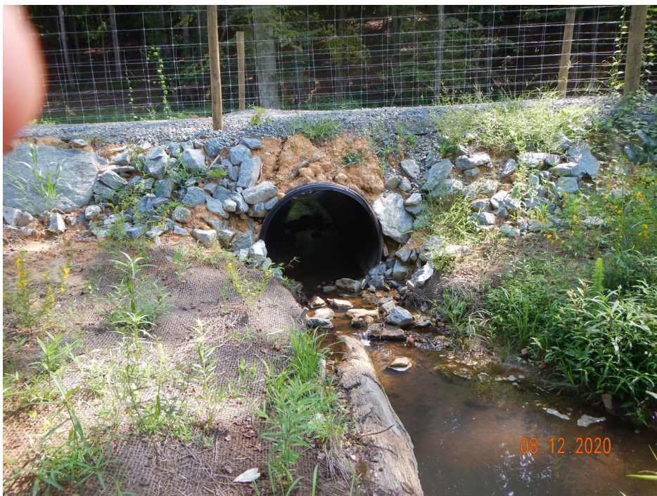
PS-3, R4, Culvert Crossing, Upstream (MY-00)
