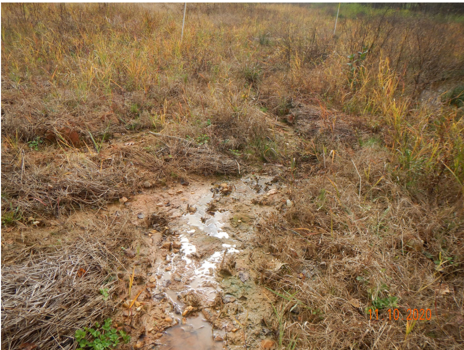
SPA5, R5 Left Floodplain, R5 Side Slope, Minor deposition and erosion as a result of erosion outside of the easement (MY-01)
