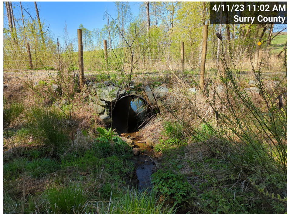
PS-3, R4, Culvert Crossing, Downstream (MY-04)
