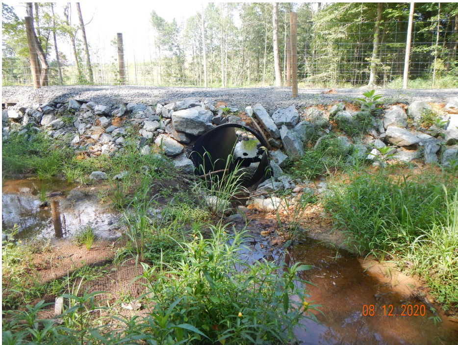
PS-3, R4, Culvert Crossing, Downstream (MY-00)
