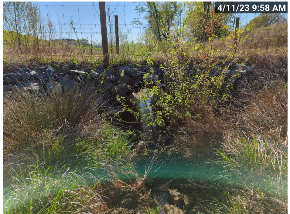
PS-1, R1, Culvert Crossing, Downstream (MY-04)
