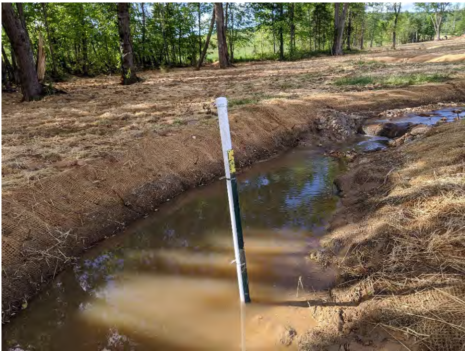
Crest Gauge (Pressure Transducer) – R5
