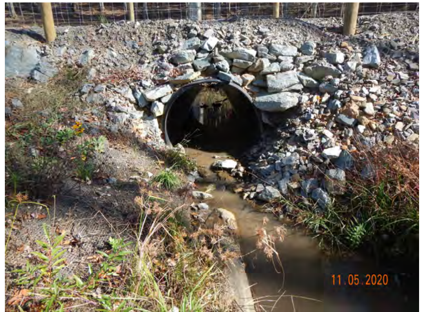
PS-3, R4, Culvert Crossing, Upstream (MY-01)
