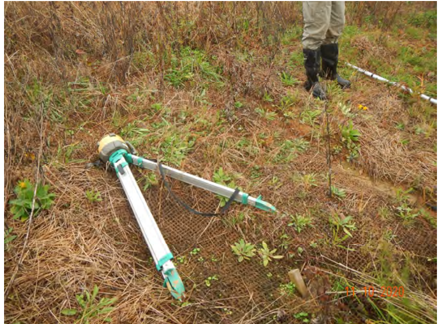
SPA2, R1 Left Floodplain, Minor Erosion (MY-01)
