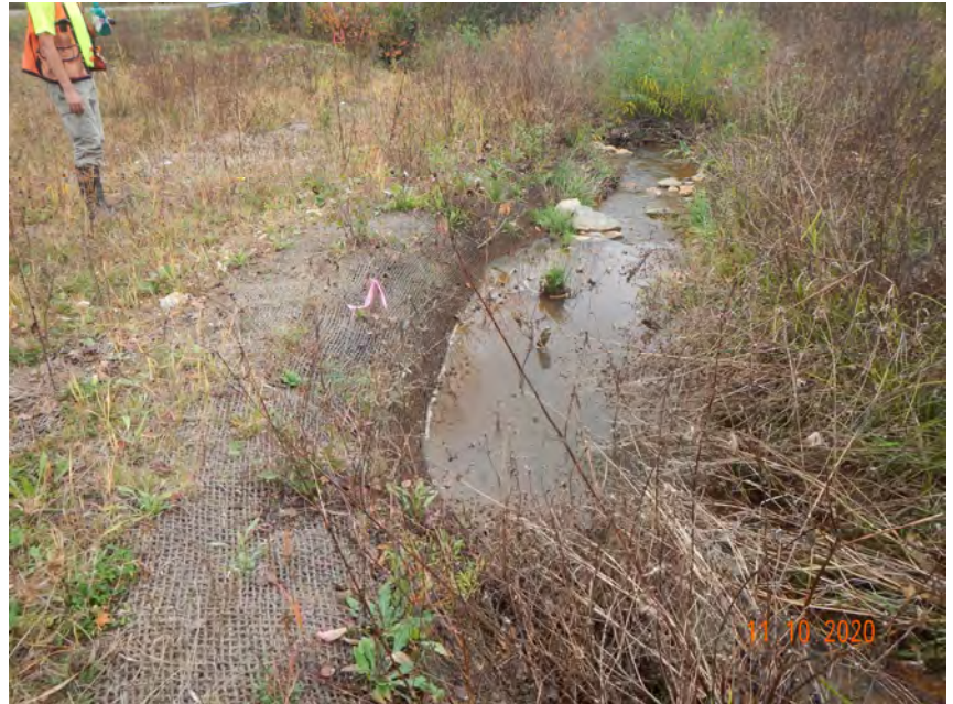
SPA7, R5 Left Bank, Functioning at Risk (MY-01)
