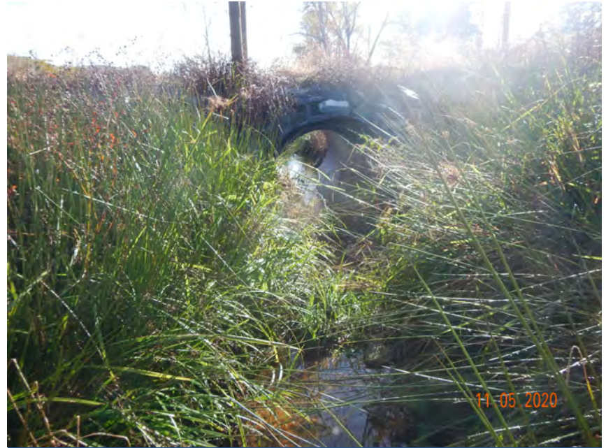
PS-1, R1, Culvert Crossing, Downstream (MY-01)
