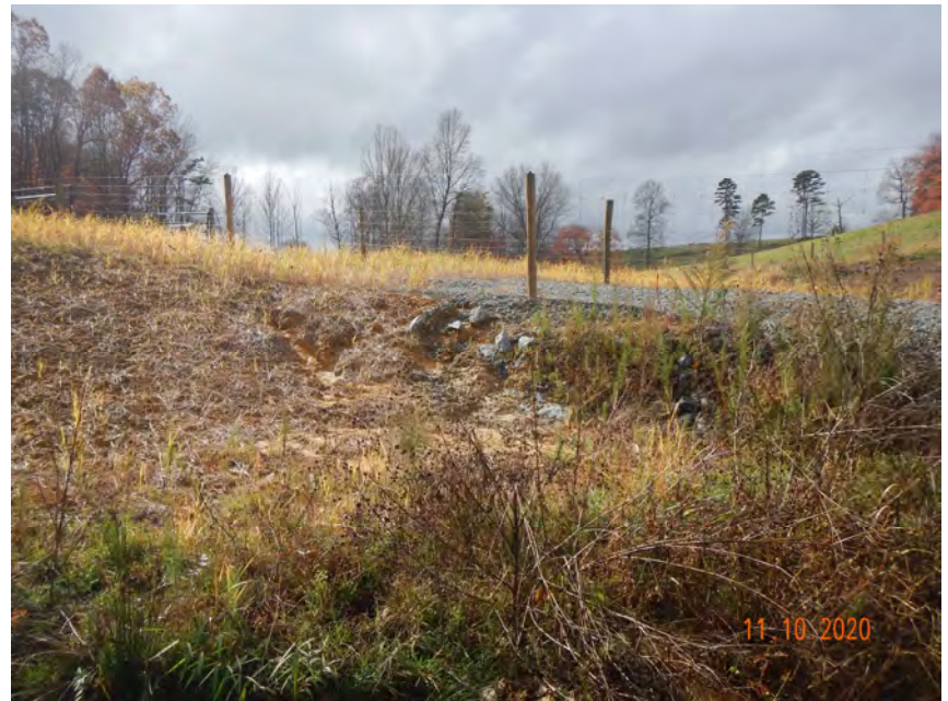
SPA4, R2 Right Floodplain, Minor Erosion (MY-01)
