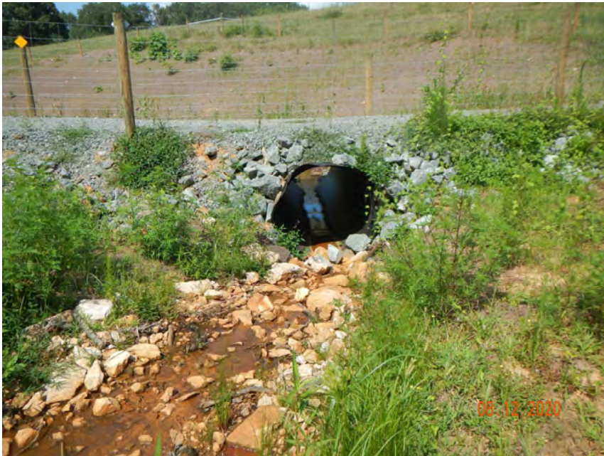
PS-2, R2, Culvert Crossing, Downstream (MY-00)
