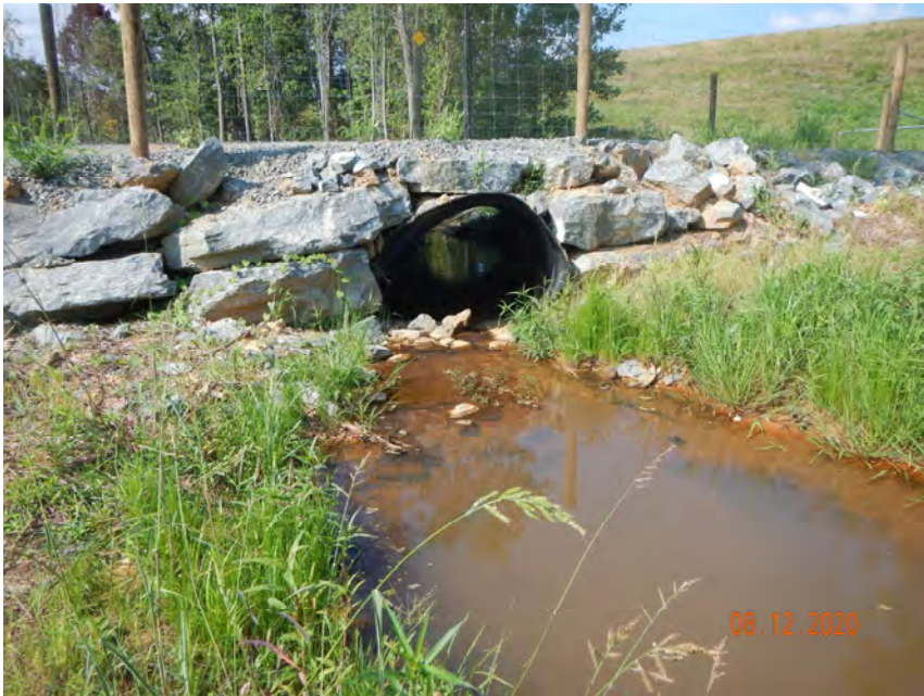
PS-6, R5, Culvert Crossing, Downstream (MY-00)
