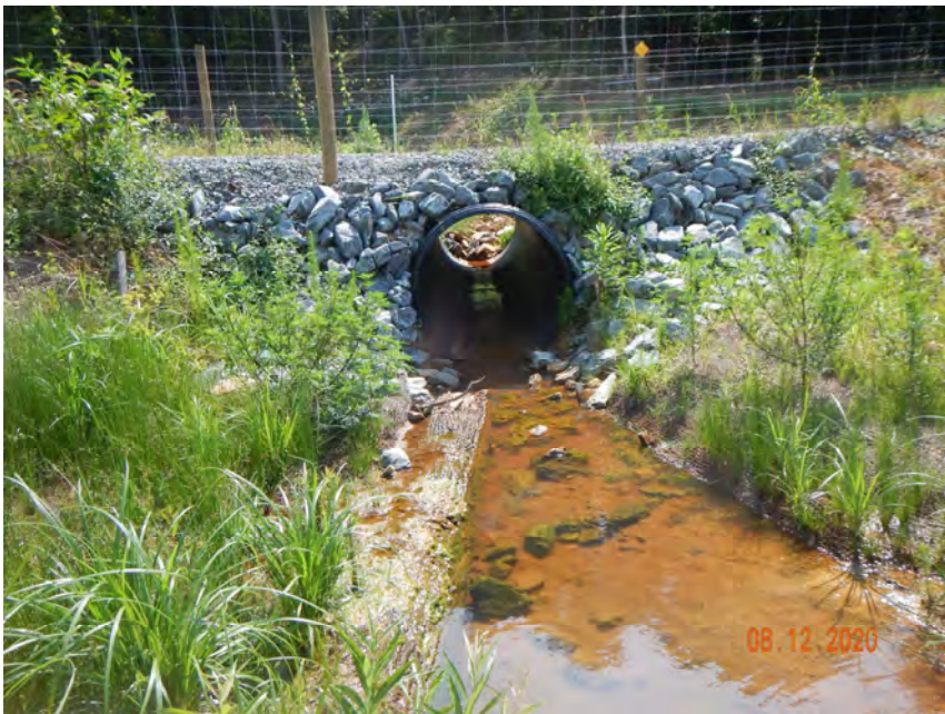
PS-2, R2 Culvert Crossing, Upstream (MY-00)
