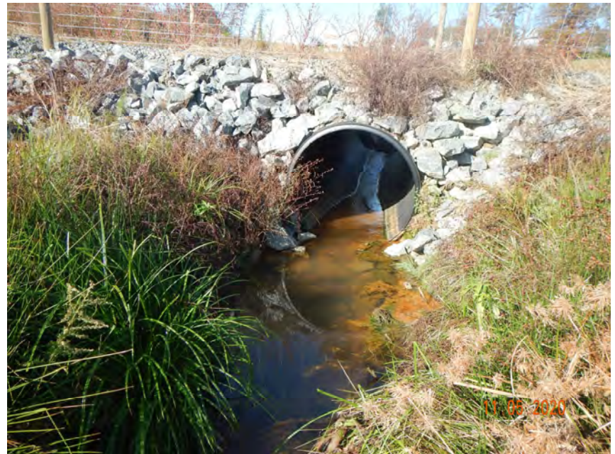
PS-1, R1, Culvert Crossing, Upstream (MY-01)
