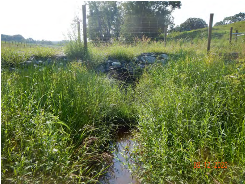
PS-1, R1, Culvert Crossing, Downstream (MY-00)
