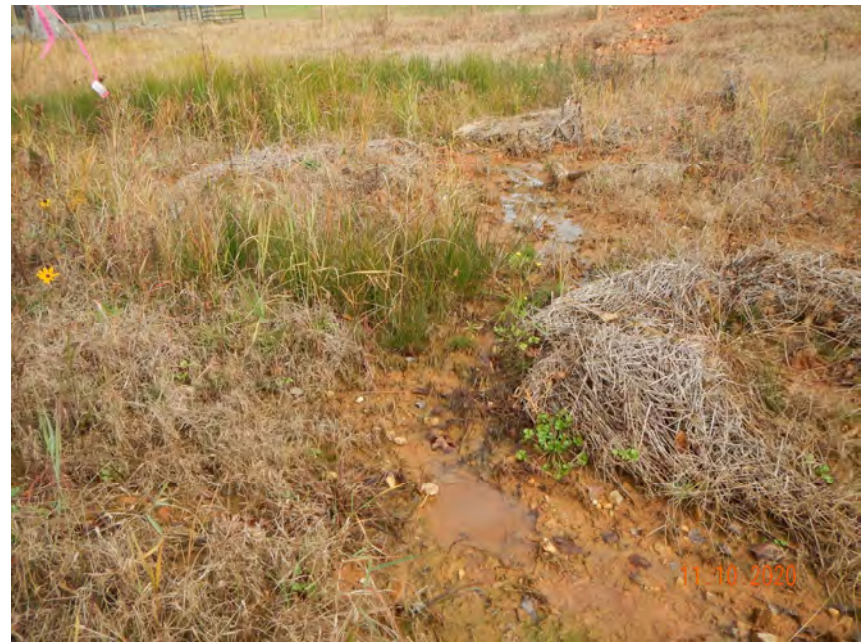
SPA5, R5 Left Floodplain, Minor Erosion (MY-01)
