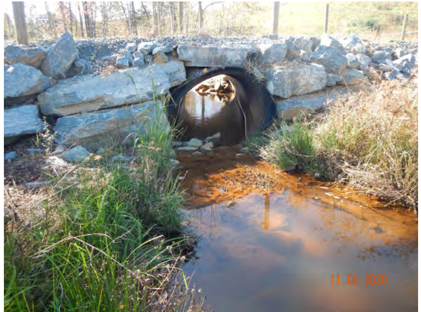
PS-6, R5, Culvert Crossing, Downstream (MY-01)
