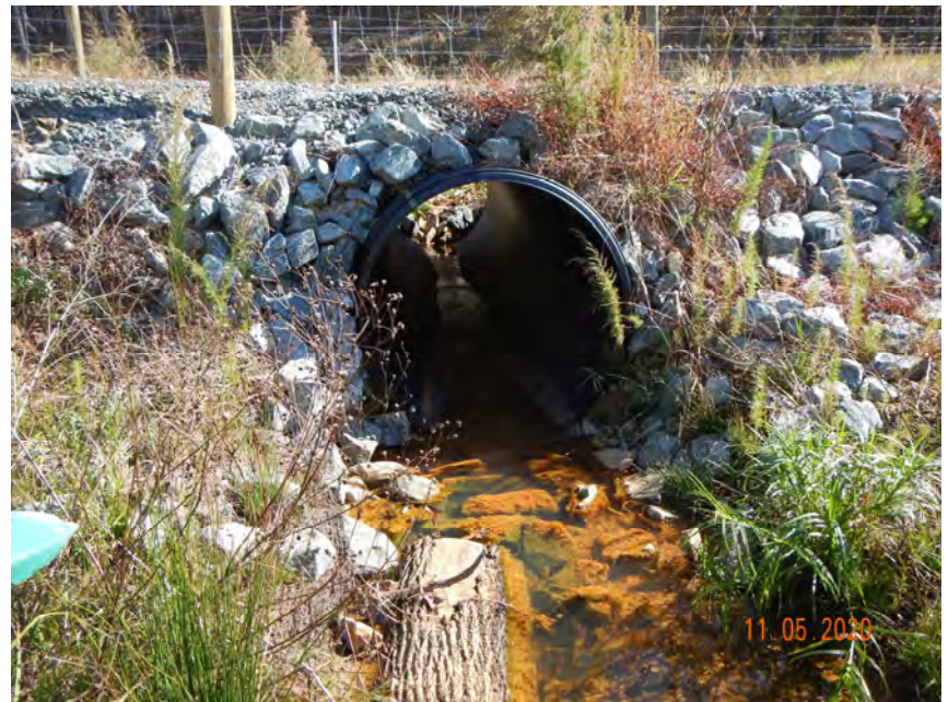
PS-2, R2, Culvert Crossing, Upstream (MY-01)
