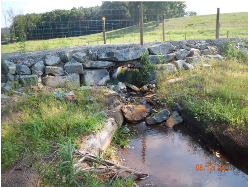
PS-6, R5, Culvert Crossing, Upstream (MY-00)
