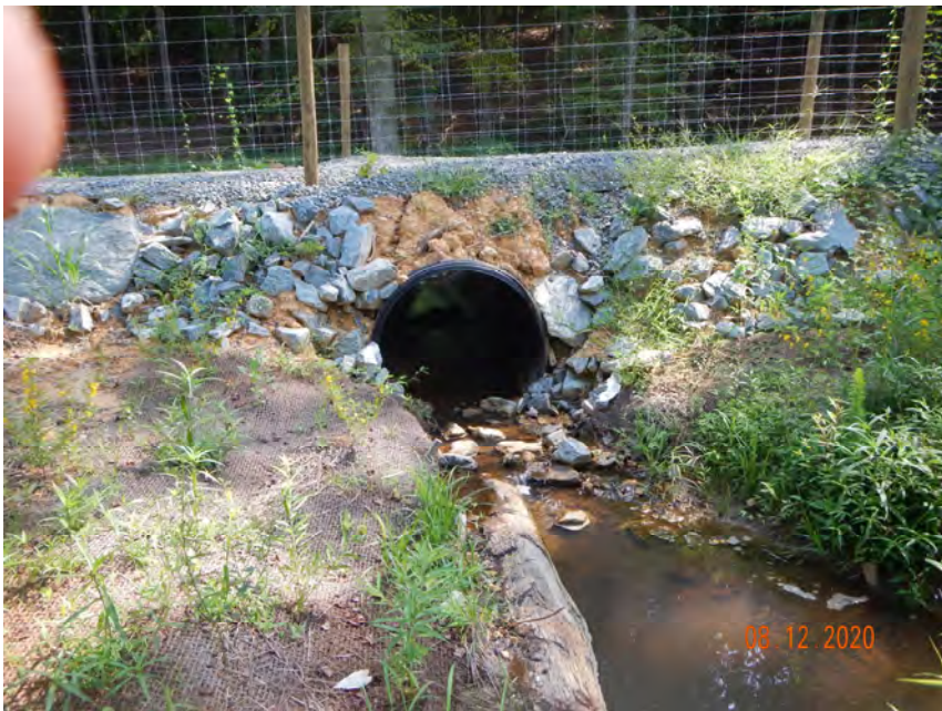
PS-3, R4, Culvert Crossing, Upstream (MY-00)
