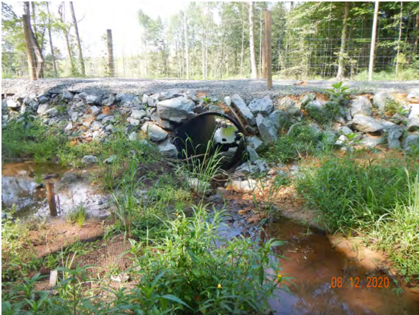
PS-3, R4, Culvert Crossing, Downstream (MY-00)
