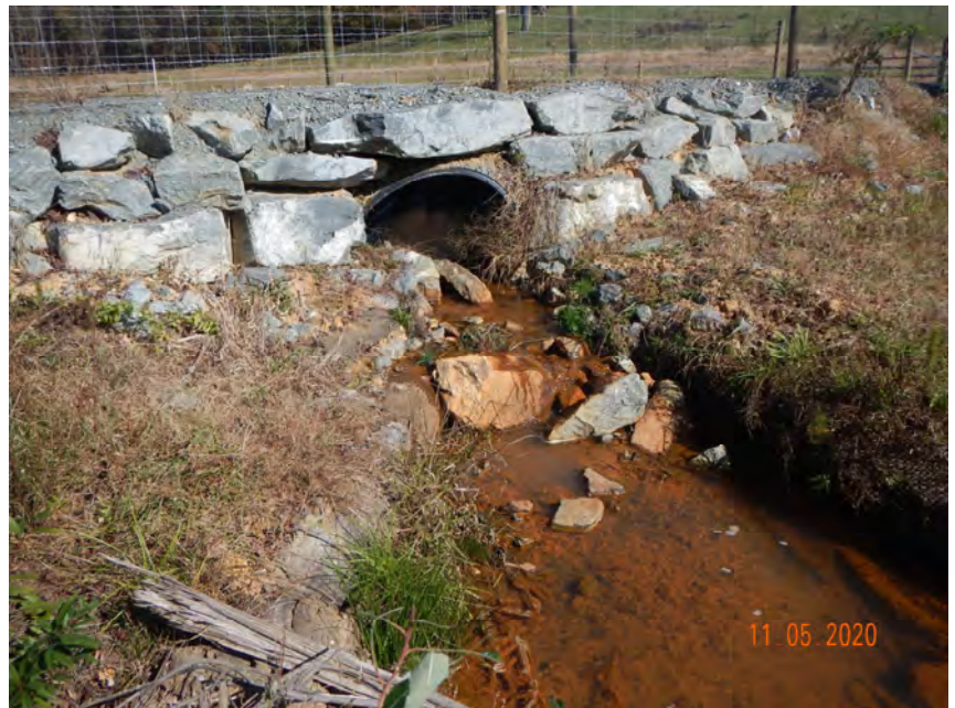
PS-6, R5, Culvert Crossing, Upstream (MY-01)
