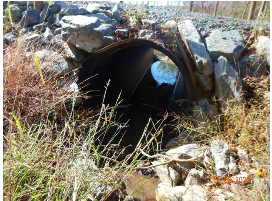
PS-3, R4, Culvert Crossing, Downstream (MY-01)
