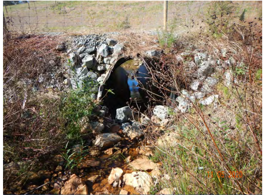
PS-2, R2, Culvert Crossing, Downstream (MY-01)
