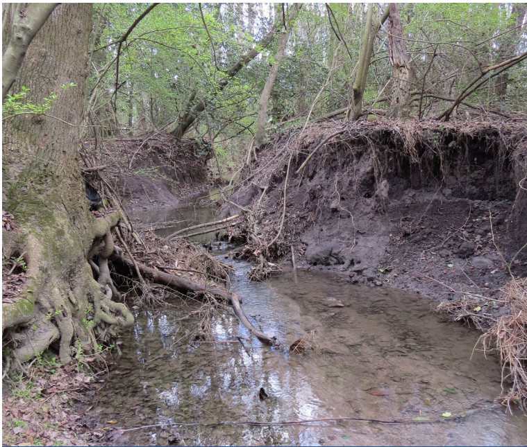
MS3 – Incised channel and bank with active scour 3/14/2018
