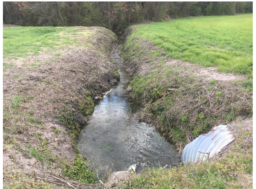
MS2 – Culvert above UT2/UT3 confluence (view south) 3/14/2018
