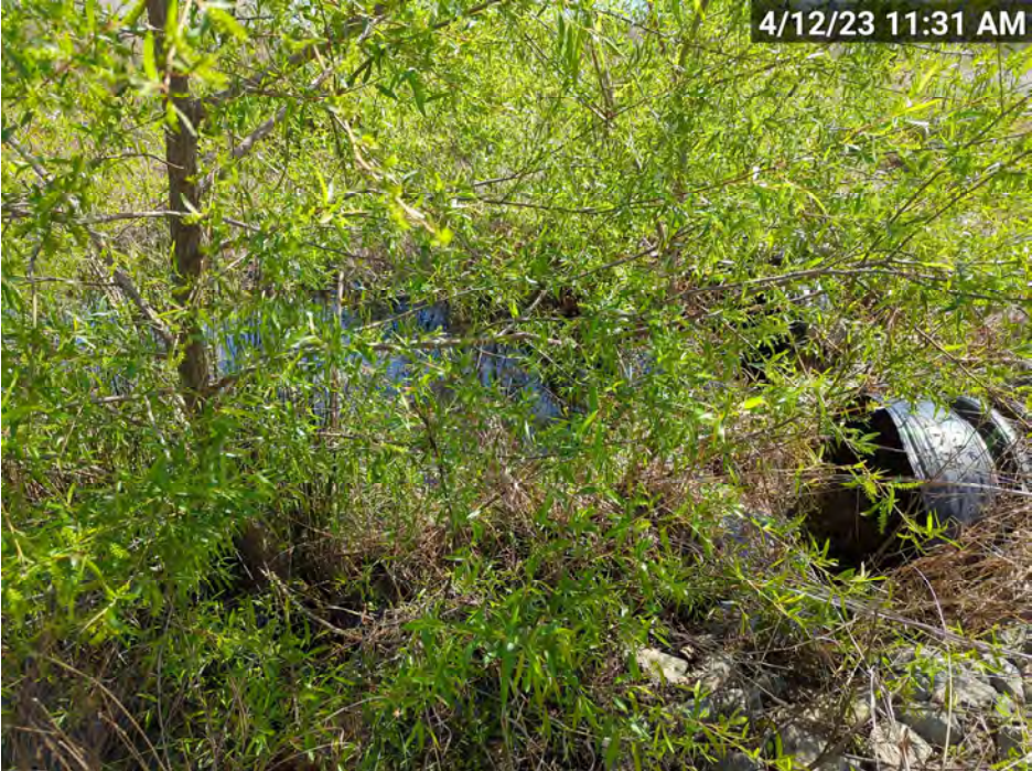
PS-2– MS2, Culvert Crossing, Downstream Left(MY-03)
