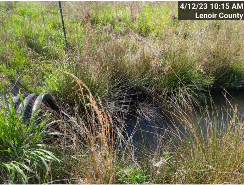
PS-1 – MS1, Culvert Crossing, Upstream Left (MY-03)
