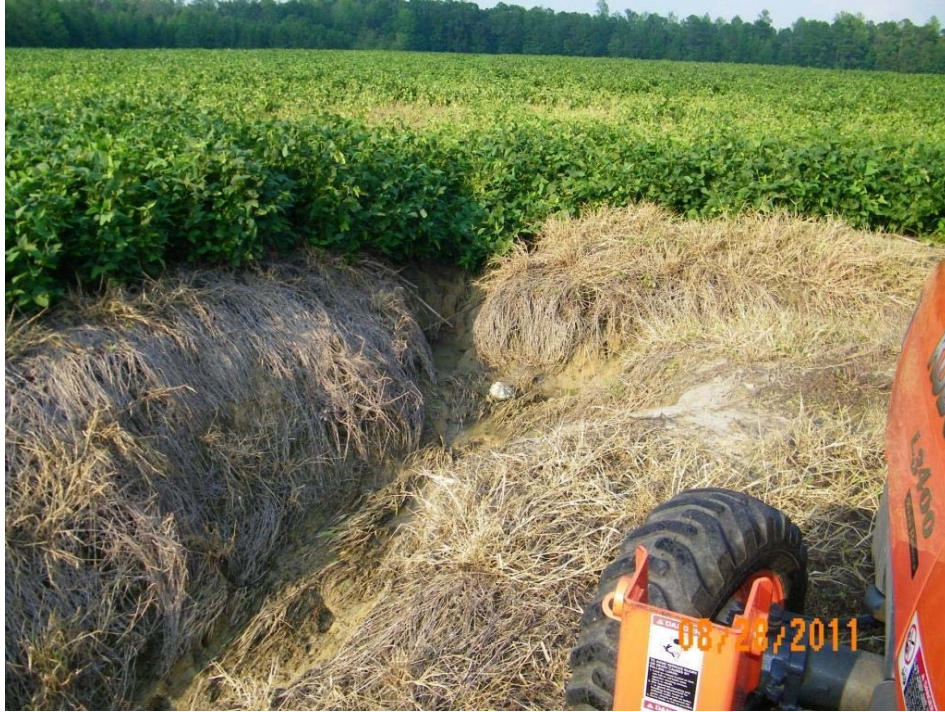
Photo #9: Facing upstream at confined flow path causing erosion from existing field
