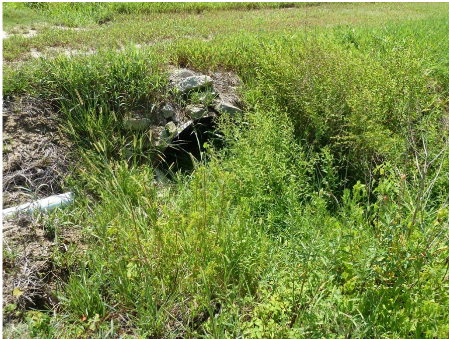
Photo #4: Facing upstream at existing culvert within proposed Reach 2
