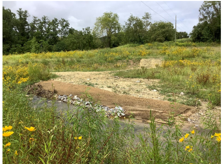
MY0-1 – NL Hunting Reach 1, 102+85 - 103+00 – Re-stabilized floodplain and left bank after repairs (09/26/2022)
