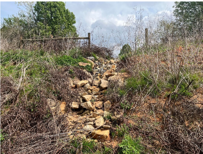
Photo Point 9a – Stabilized swale, view up valley (04/06/2023)
