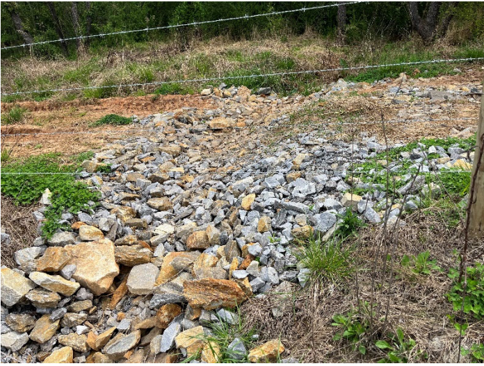
Photo Point 2a – Stabilized swale, view up valley (04/06/2023)
