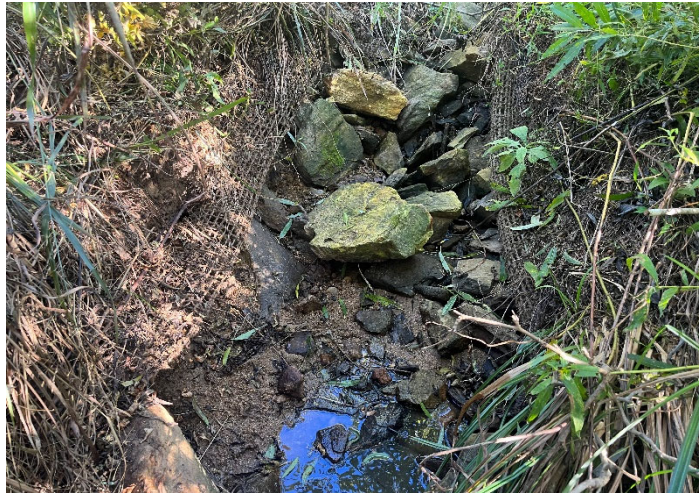
MY2-3 – UT1 Reach 3, station 219+80 to 219+86 – Isolated riffle scour (10/17/2023)
