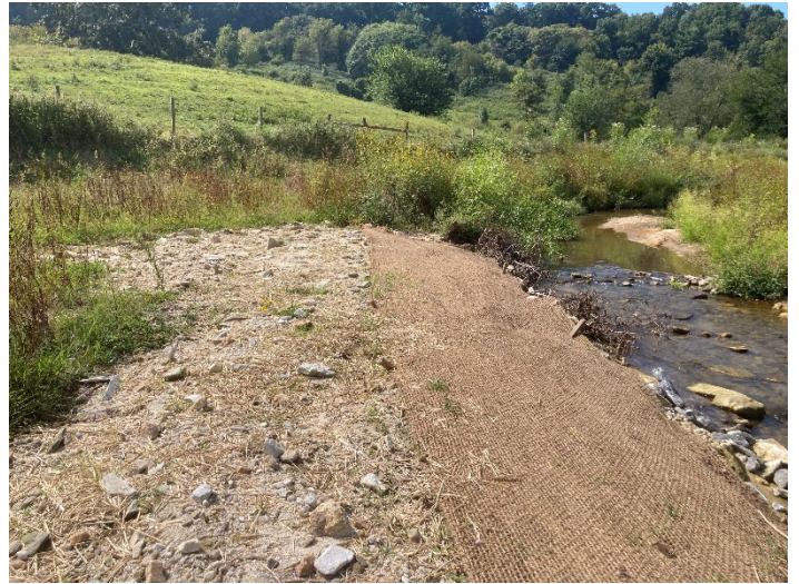
MY0-1 – NL Hunting Reach 1, 102+25 - 102+75 – Re-stabilized right bank after repairs (09/26/2022)
