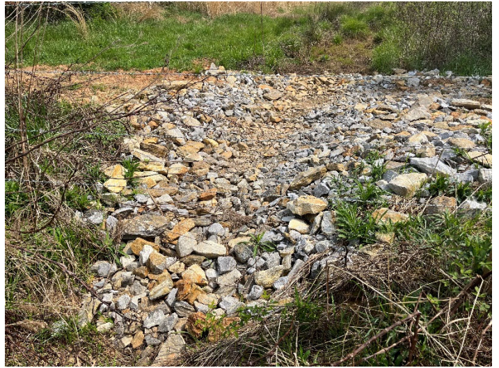
Photo Point 8a – Stabilized swale, view up valley (04/06/2023)
