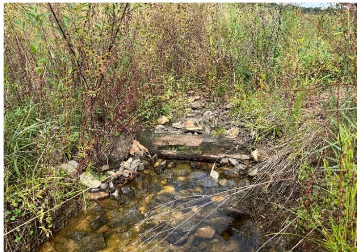
UT1 Reach 1, station 210+45 – Additional installed log sill after repairs (09/26/23)
