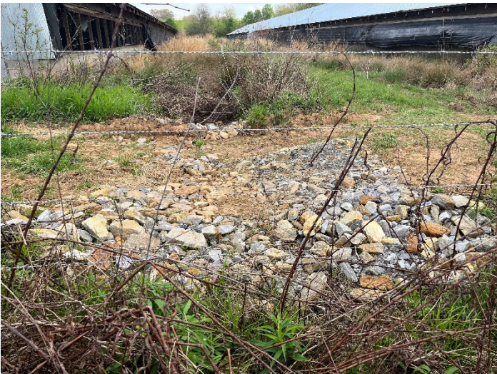
Photo Point 3a – Stabilized swale, view up valley (04/06/2023)
