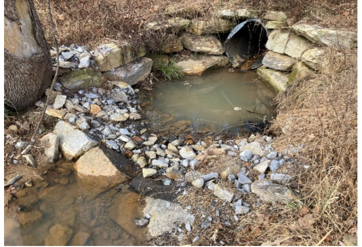
MY1-2 – UT1 Reach 3, station 218+23 – Rock sill after repairs (01/08/2023)
