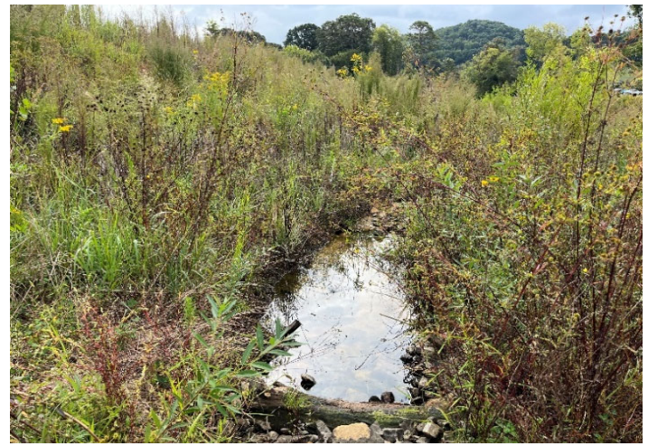
MY1-1 – UT1 Reach 1, station 210+50 to 210+70 – Re-stabilized riffle after repairs (09/26/2023)
