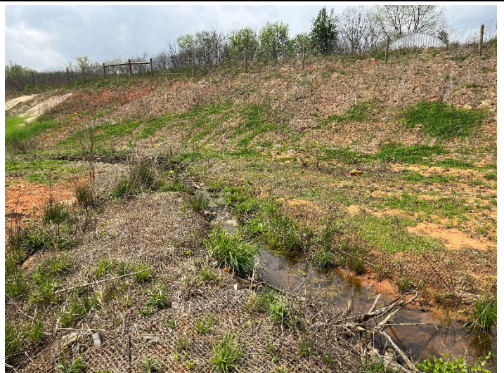
Photo Point 6a – Stabilized swale, view down valley (04/06/2023)
