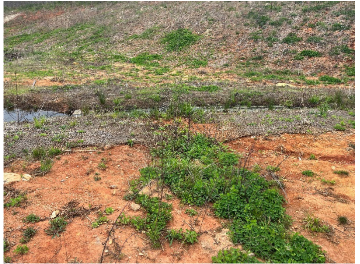
Photo Point 4a – UT1 Reach 1, view down valley (04/06/2023)
