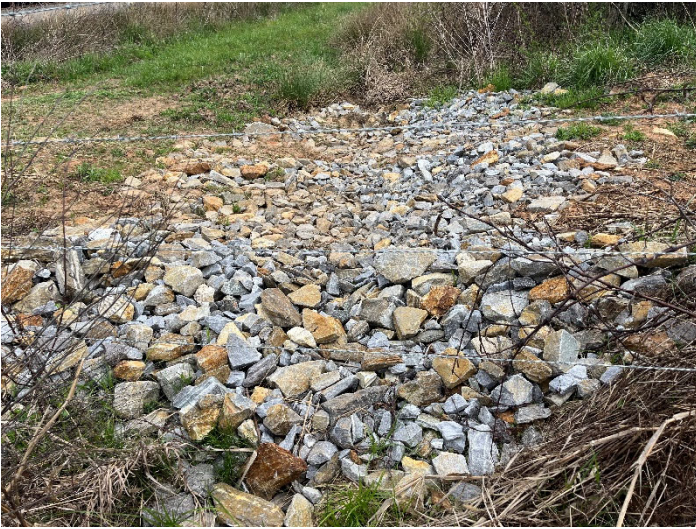
Photo Point 7a – Stabilized swale, view up valley (04/06/2023)
