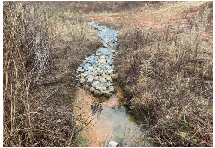
MY0-2 – UT1 Reach 1, station 210+50 to 212+00 – Re-stabilized riffle after repairs (01/08/2023)
