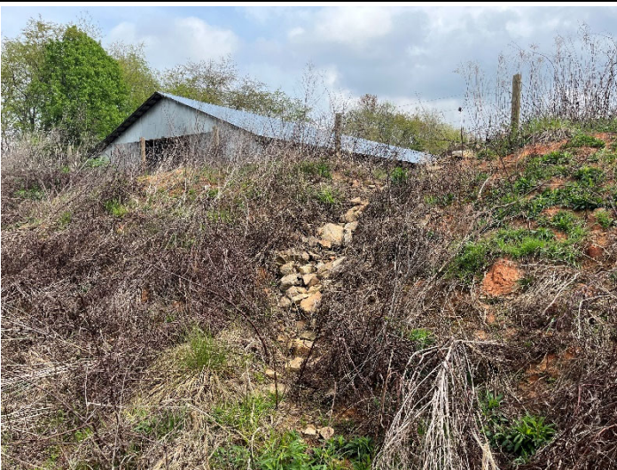
Photo Point 6a – Stabilized swale, view up valley (04/06/2023)
