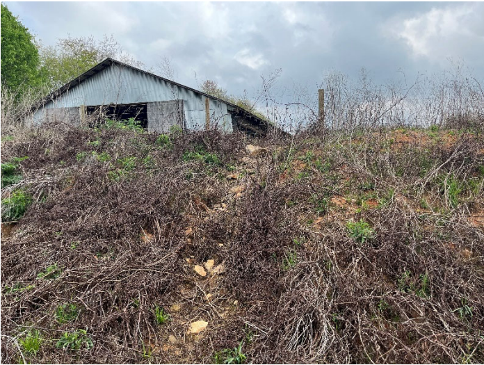
Photo Point 4a – Stabilized swale, view up valley (04/06/2023)
