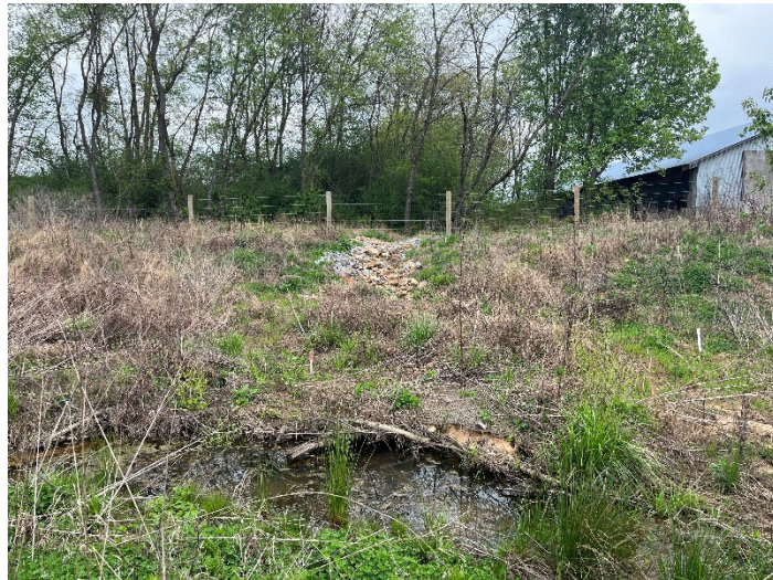
Photo Point 5a – Stabilized swale, view up valley (04/06/2023)
