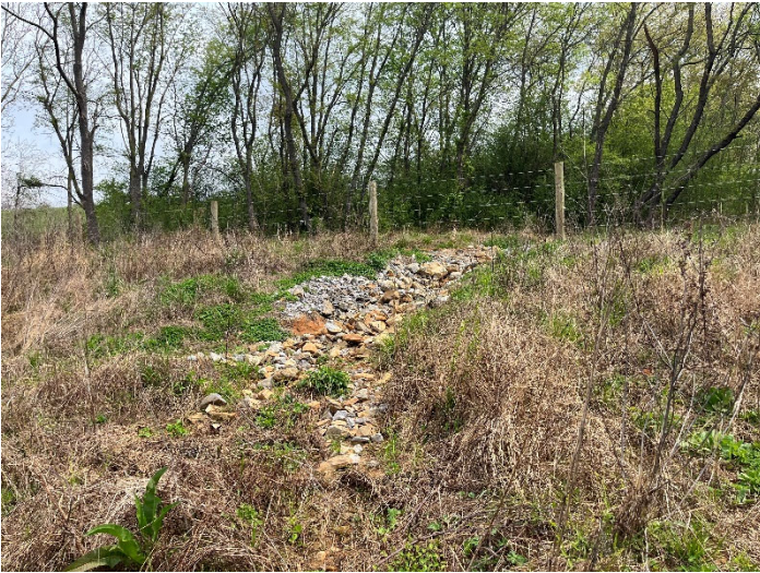
Photo Point 1a – Stabilized swale, view up valley (04/06/2023)
