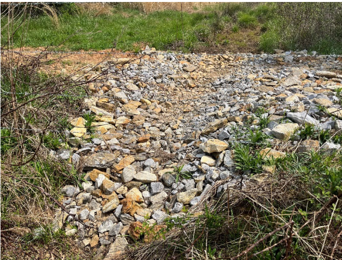
Photo Point 8a – Stabilized swale, view up valley (04/06/2023)
