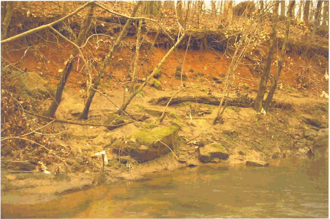
March 5 - Photo 64: Taken at Segment 63, 1632-1652 m., Left Bank
