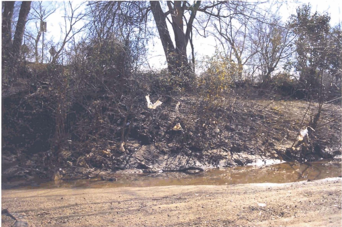
March 3 - Photo 35: Taken at Segment 9, 160-180 m., Left Bank
