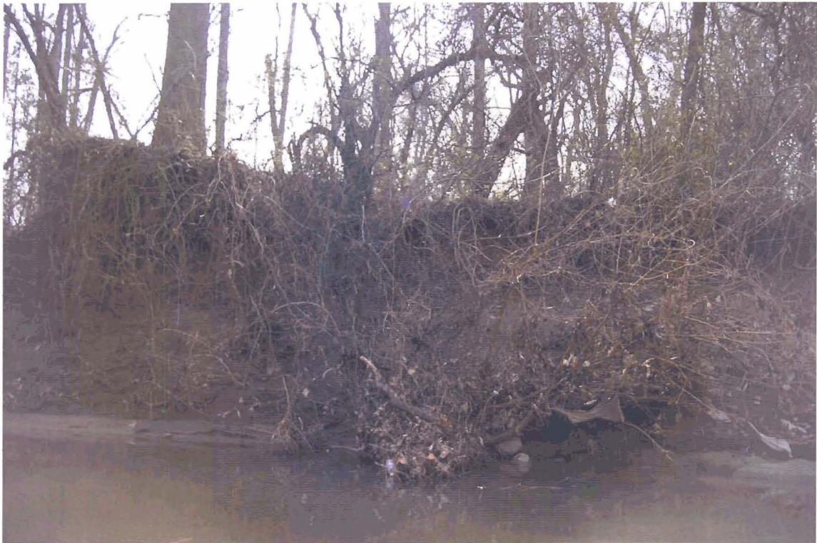
March 4 - Photo 29: Taken at Segment 21, 400-420 m., Left Bank
