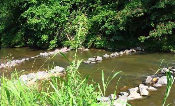
Photo Point 1: Downstream structure left in place to avoid disturbance to wetlands and stream banks in addition to provide potential aquatic habitat and channel grade control
