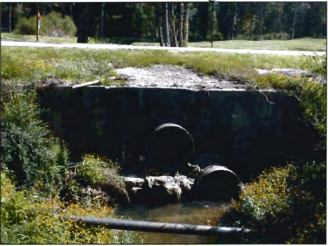
Channel A entrance road crossing/culverts
