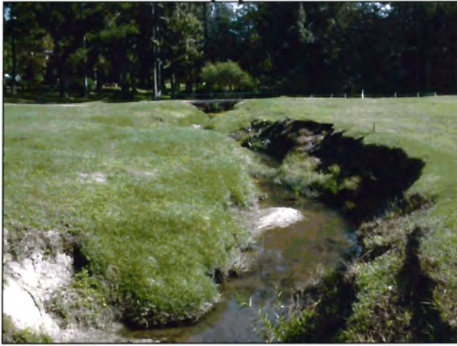
Channel A near end of project
