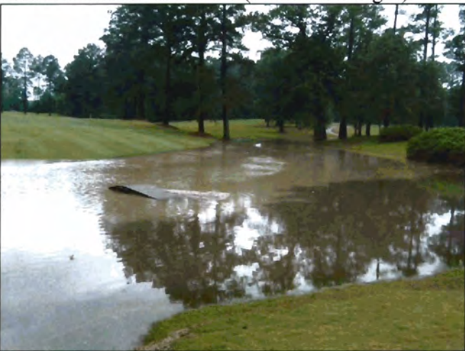
Channel A after rain event (note foot bridges)
