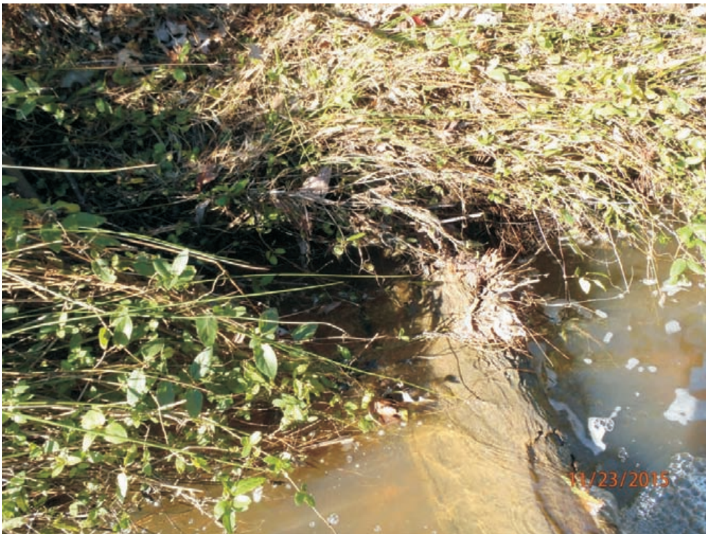
Reach 1A - Stream Problem Areas #10; Log Vane Undercut
