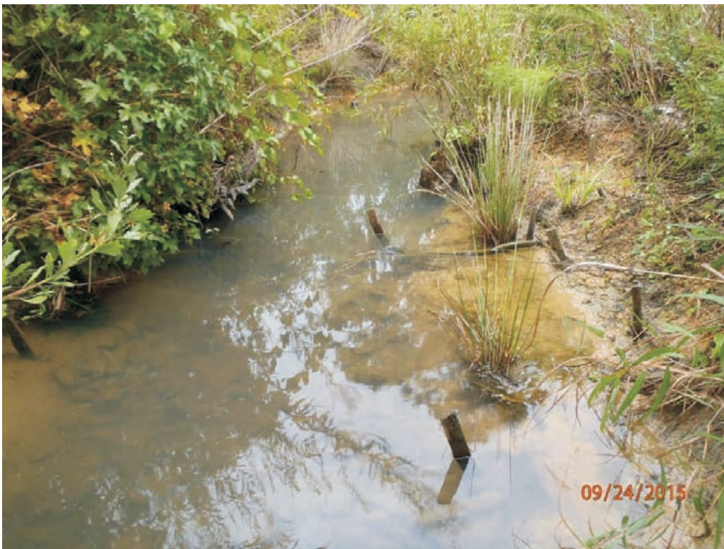
Reach 2A - Stream Problem Area #48; Scour
