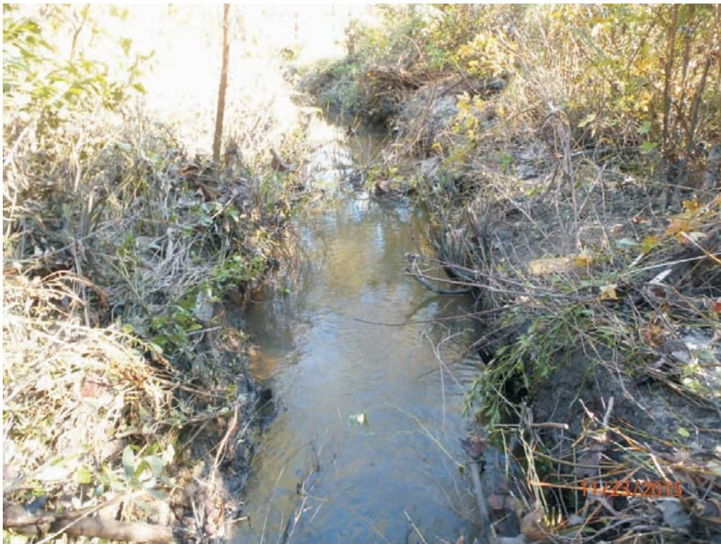
Reach 1A - Stream Problem Area #20; Degradation
