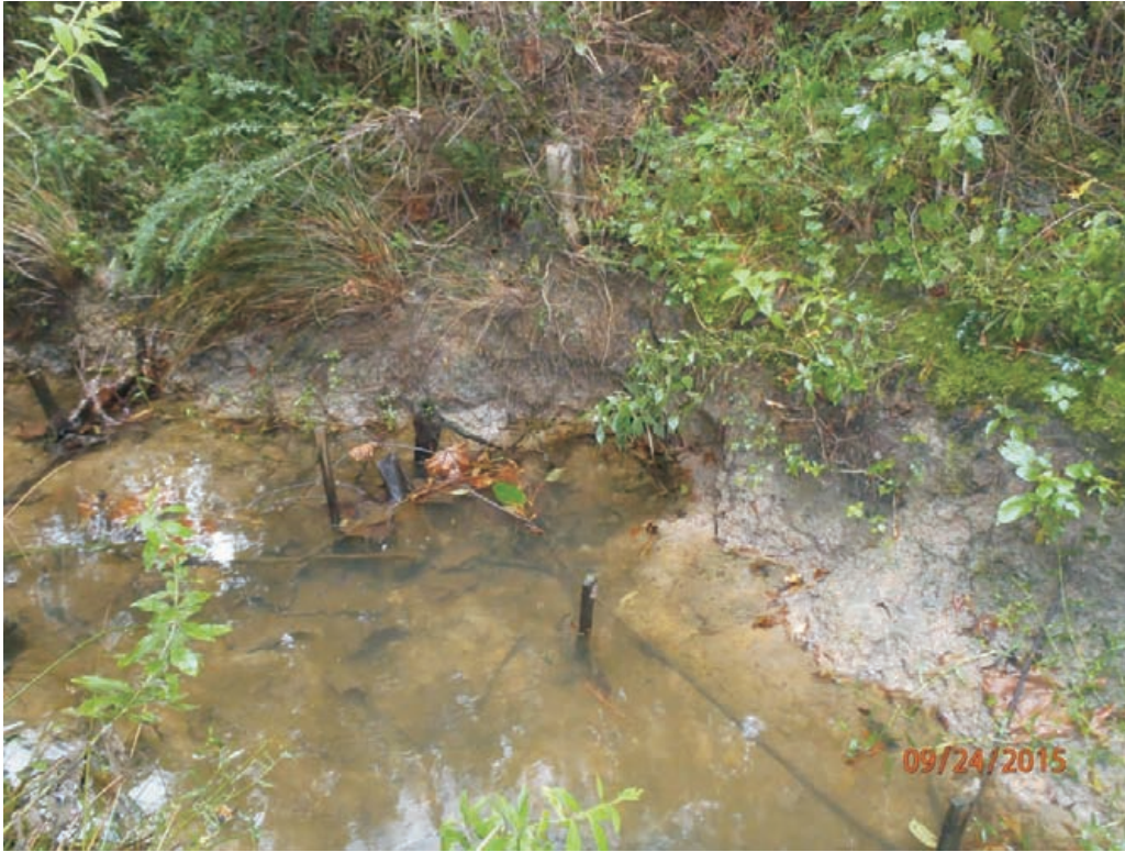
Reach 2A - Stream Problem Area #31; Scour
