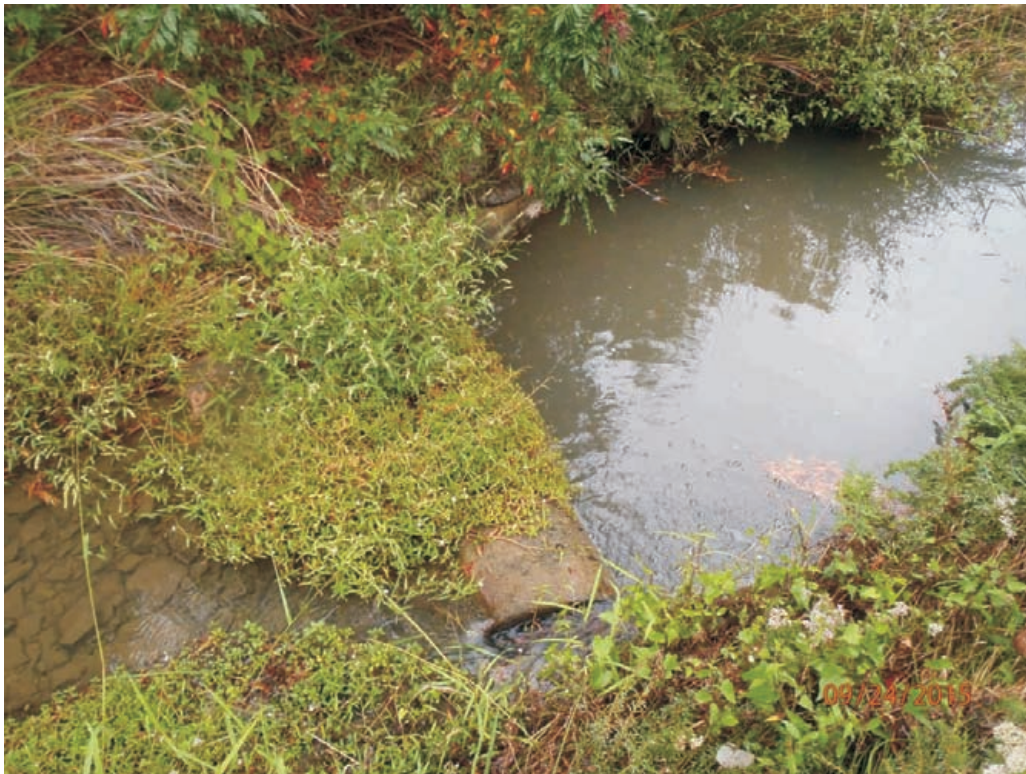
Reach 2A - Stream Problem Area #44; Log Vane Scour
