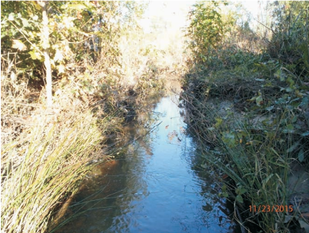
Reach 1A - Stream Problem Area #23; Degradation
