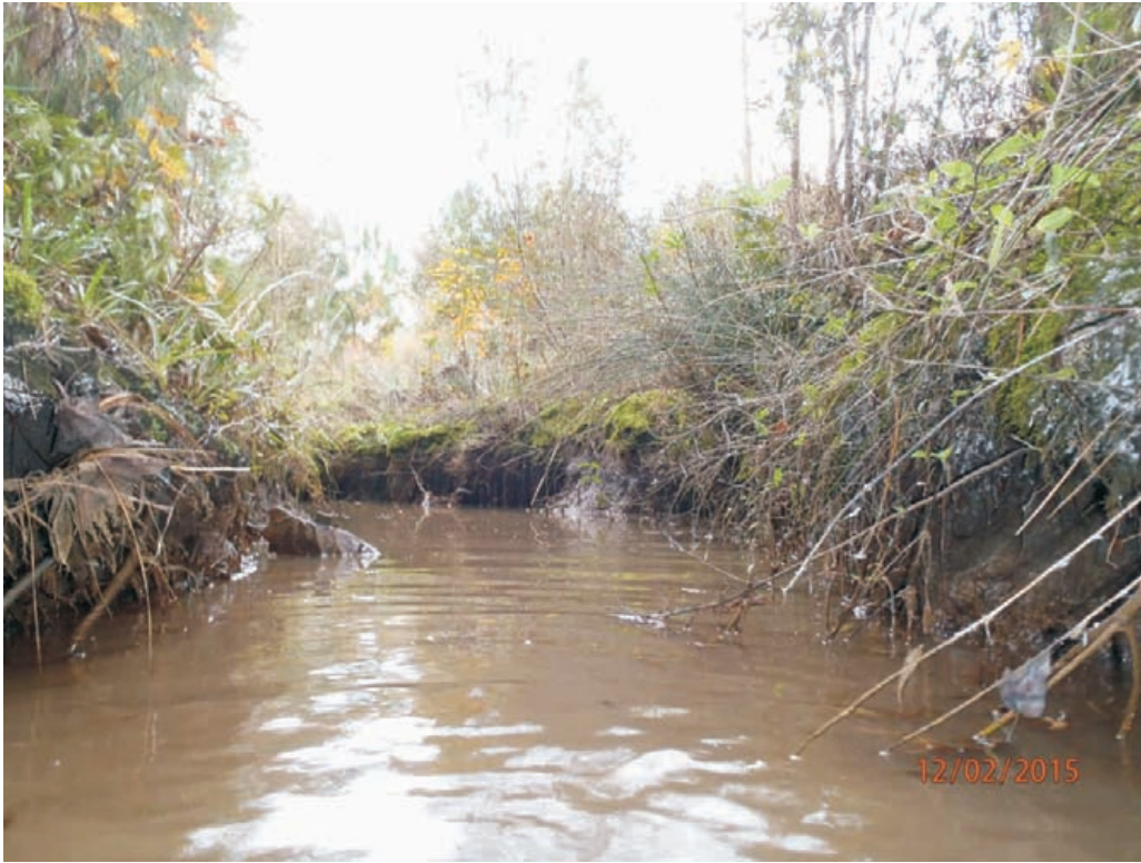
Reach 2A - Stream Problem Area #37; Undercut
