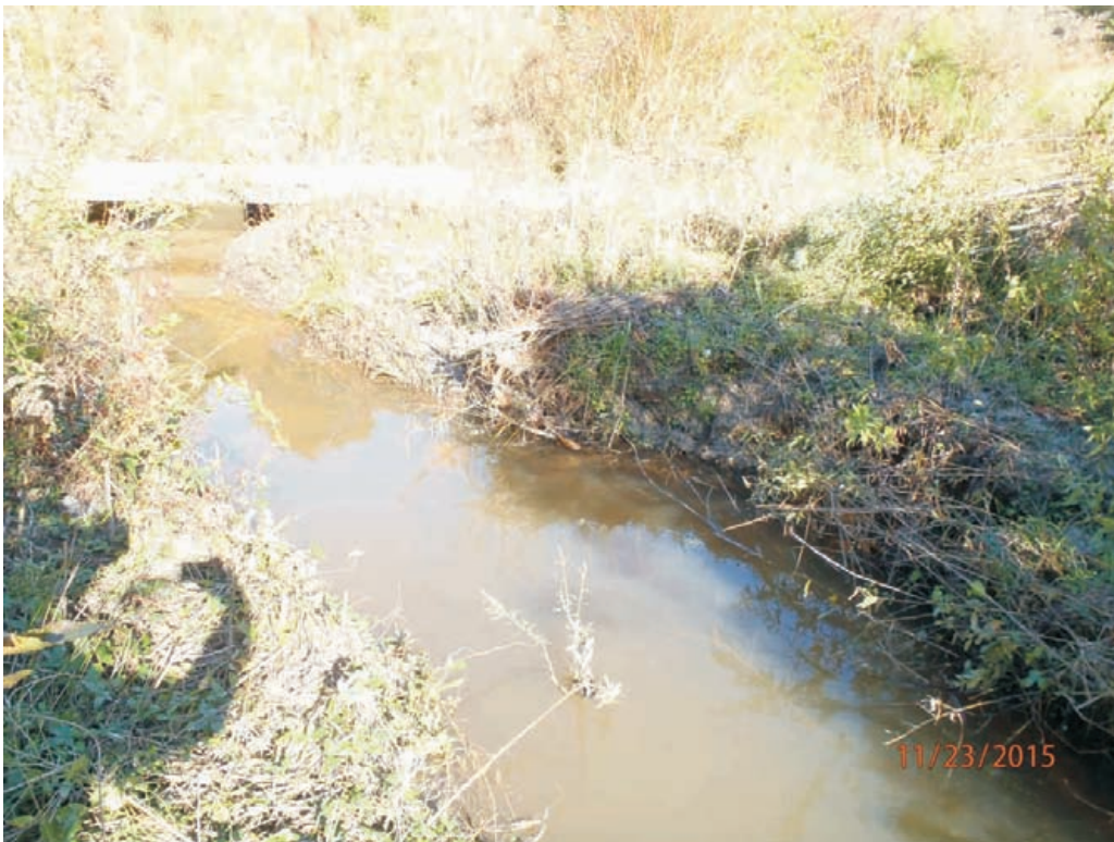
Reach 1A - Stream Problem Area #12; Scour
