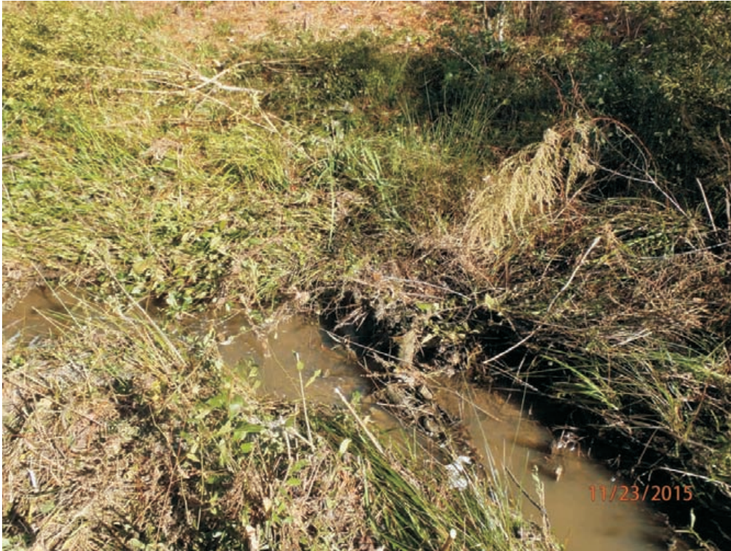
Reach B - Stream Problem Area #53; Undercut
