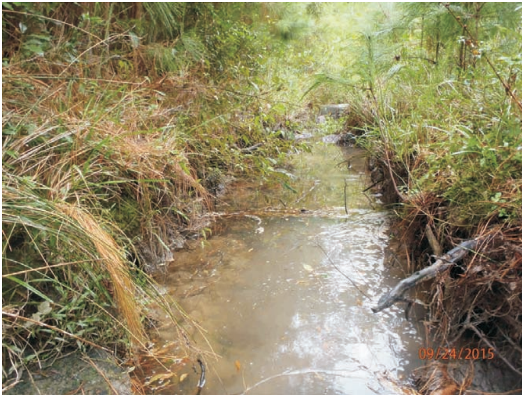
Reach 2A - Stream Problem Area #38; Degradation
