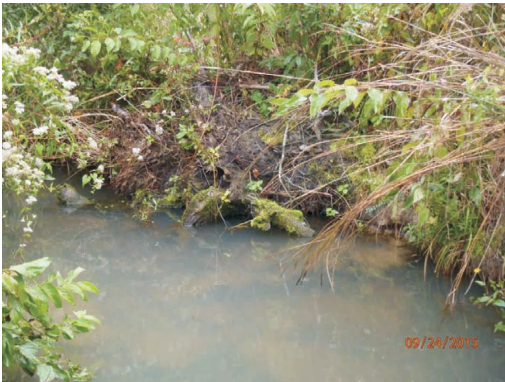
Reach 2A - Stream Problem Area #50; Undercut
