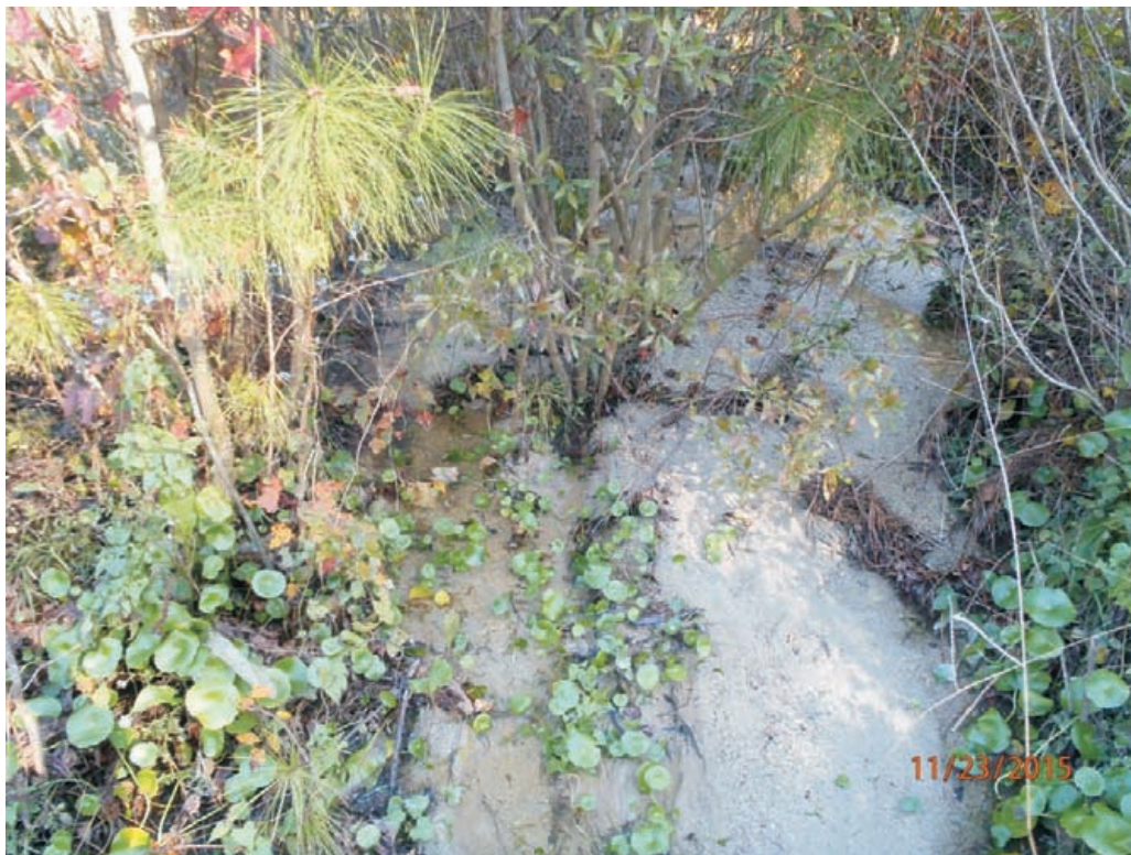
Enhancement Reach - Stream Problem Area #56; Aggradation
