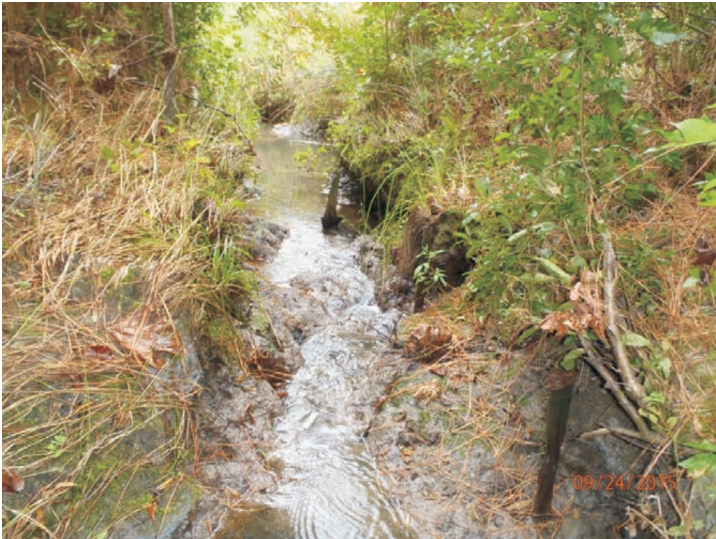
Reach 2A - Stream Problem Area #36; Degradation
