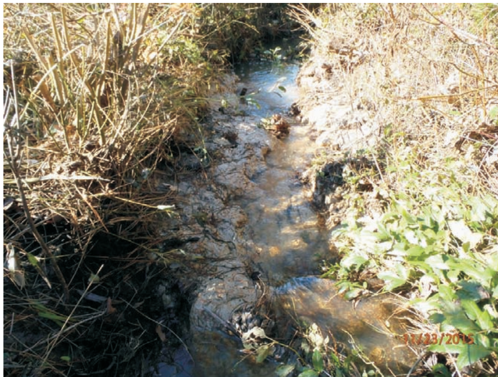
Reach B - Stream Problem Area #54; Degradation
