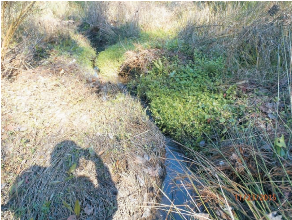
Reach 1A - Stream Problem Area 2; Degradation
