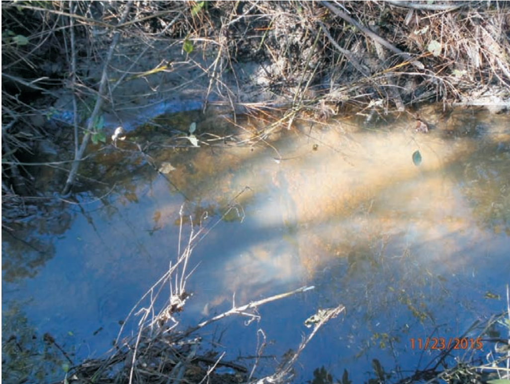
Reach B - Stream Problem Area #55; Undercut
