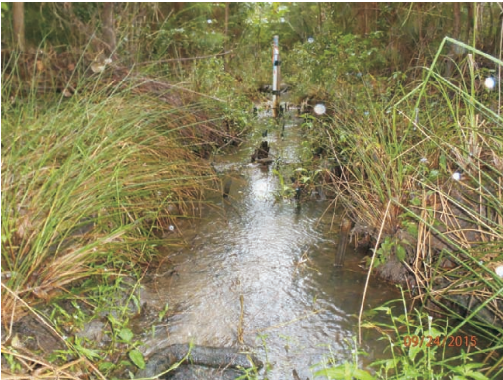
Reach 2A - Stream Problem Area #28: Degradation
