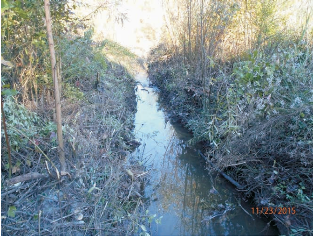
Reach 1A - Stream Problem Area #17; Degradation
