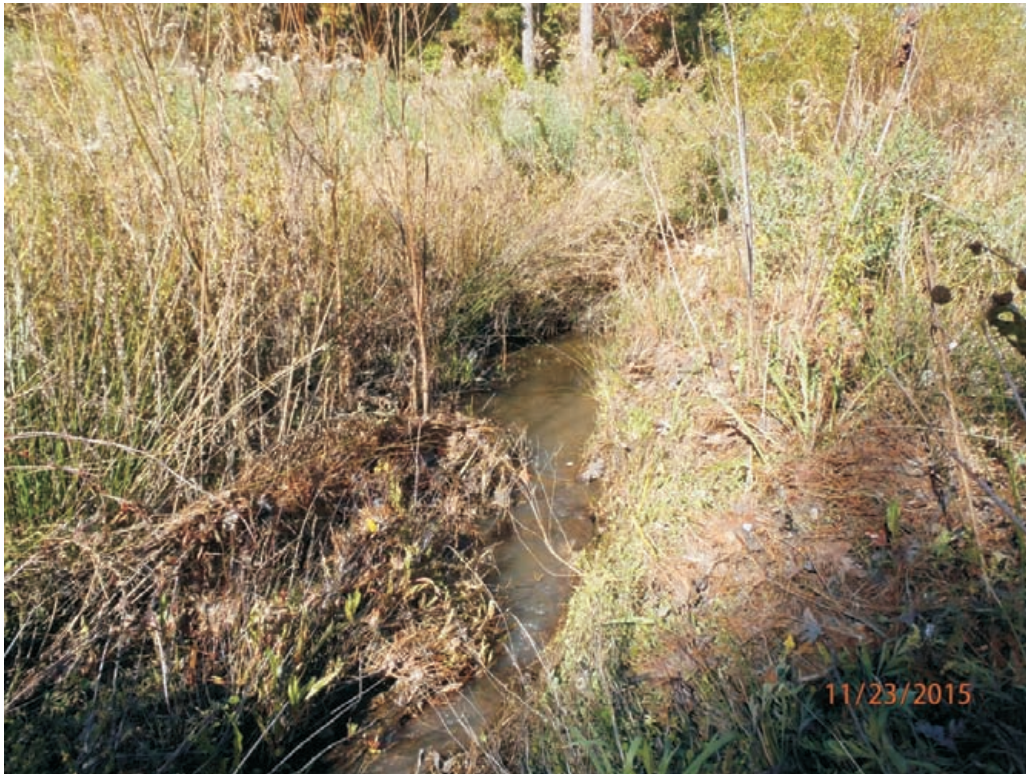
Reach 1A - Stream Problem Area #3; bank undercut
