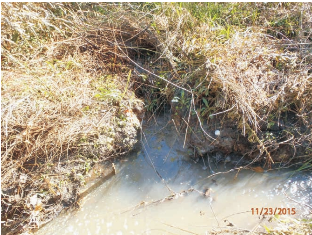
Reach B - Stream Problem Area #52; Mass Wasting
