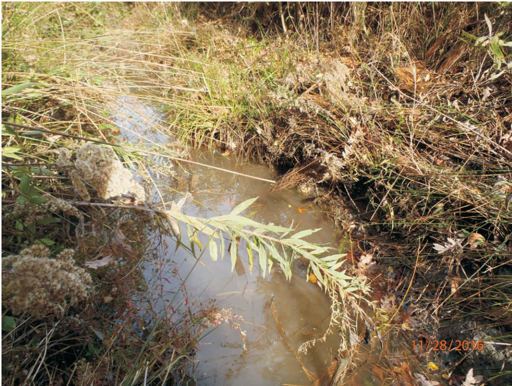
Reach 1A - Stream Problem Area #10; Log Vane Undercut becoming scour
