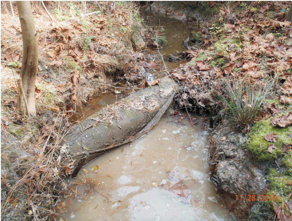
Reach 2A - Stream Problem Area #31; Scour
