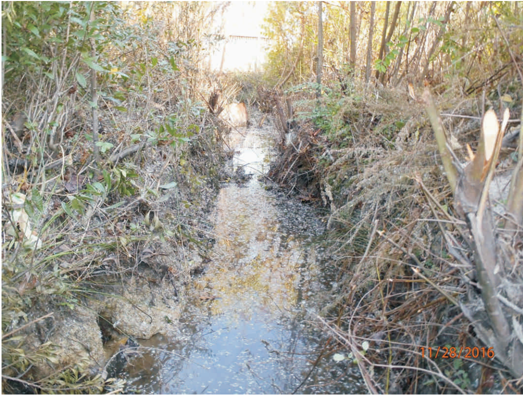
Reach 1A - Stream Problem Area #20; Degradation
