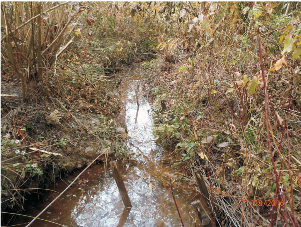
Reach B - Stream Problem Area #54; Degradation
