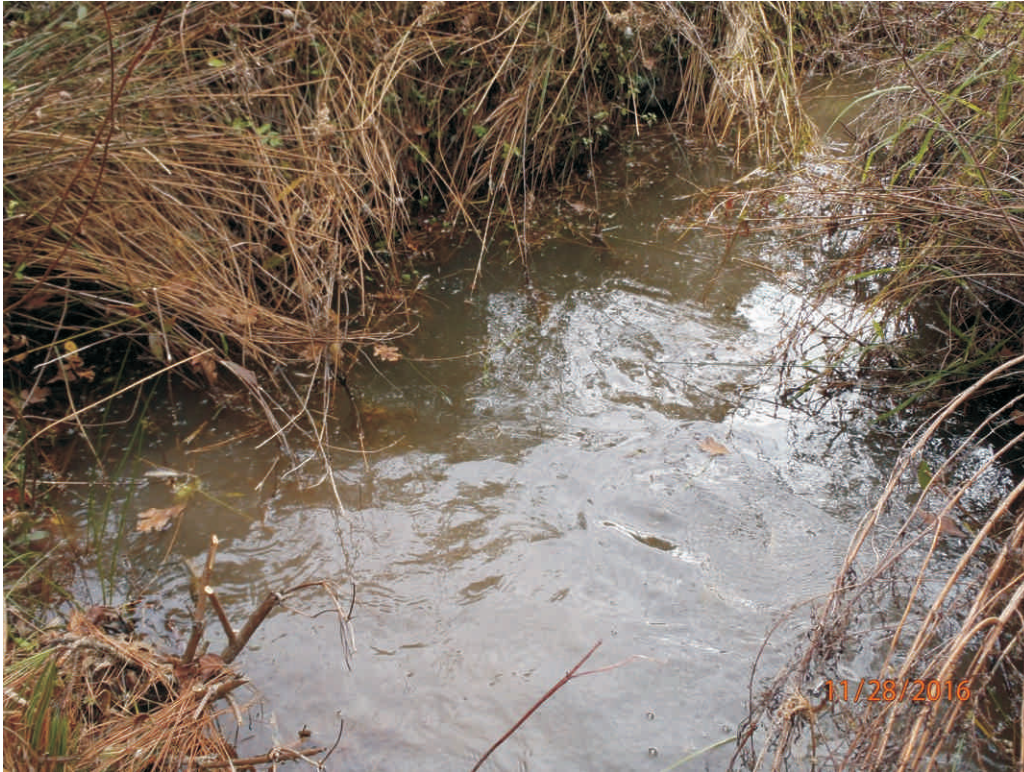
Reach 1A - Stream Problem Area #3a; scour
