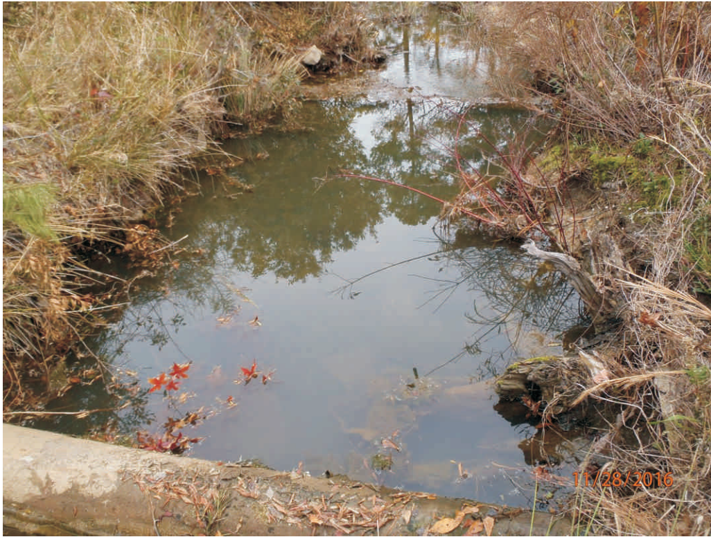
Reach 2A - Stream Problem Area #45a; Log Vane Scour
