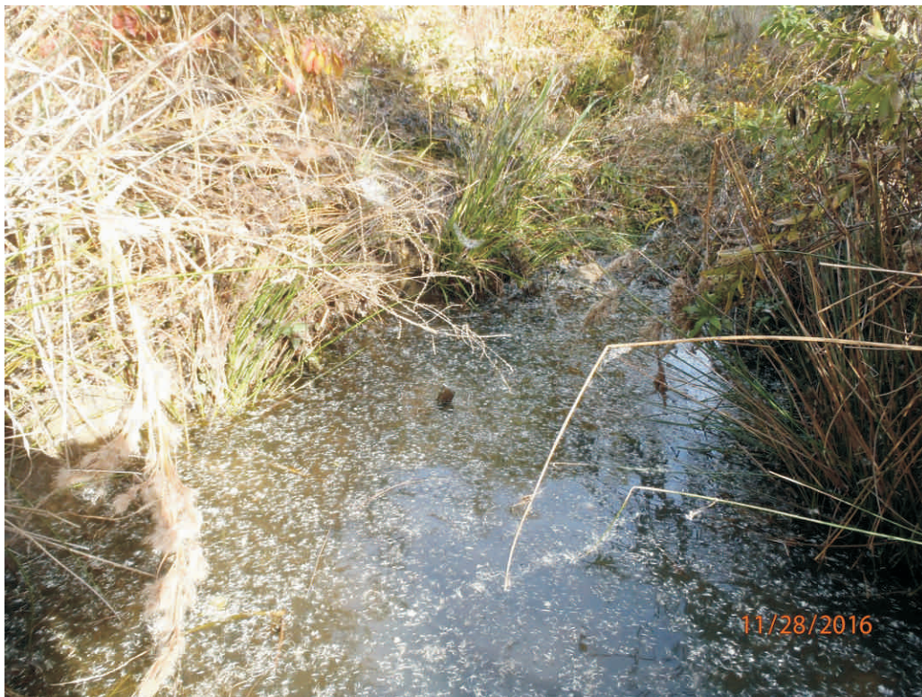
Reach 1A - Stream Problem Area #14; Scour
