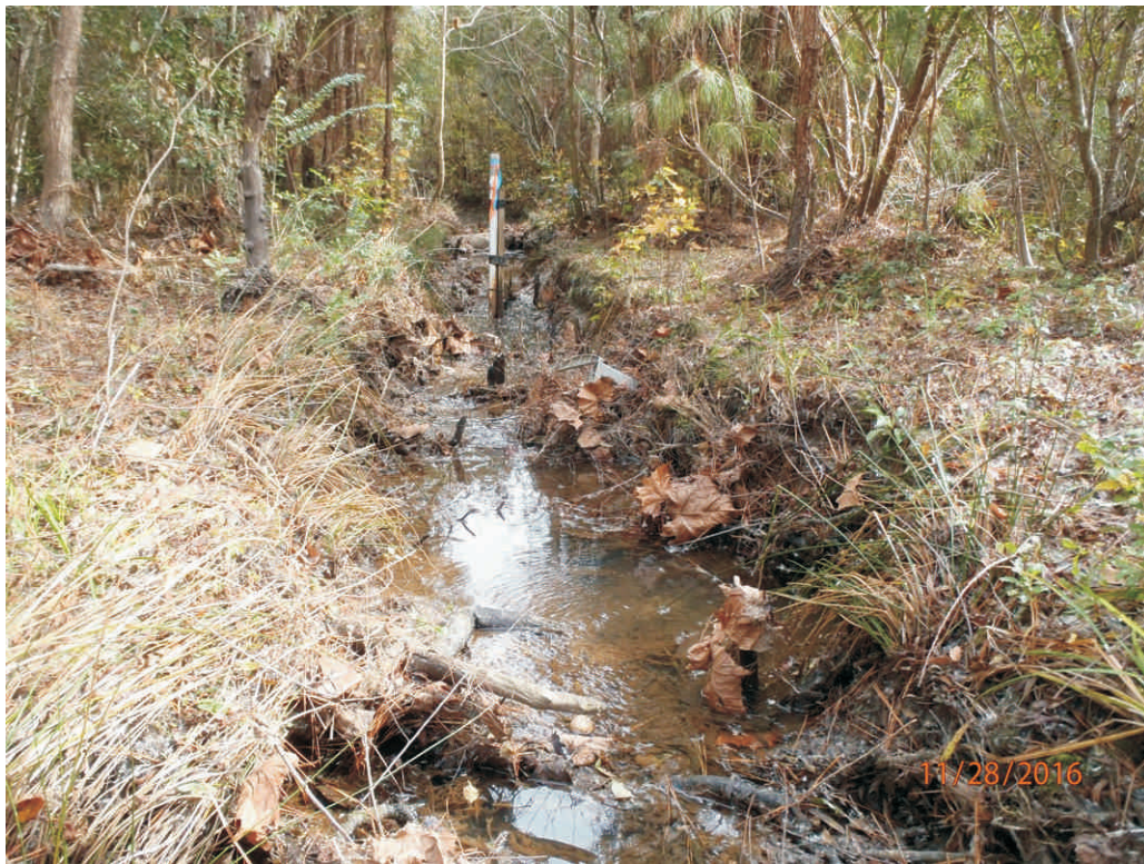
Reach 2A - Stream Problem Area #28; Degradation
