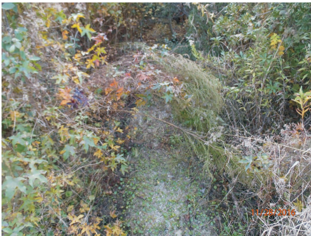
Enhancement Reach - Stream Problem Area #56; Aggradation
