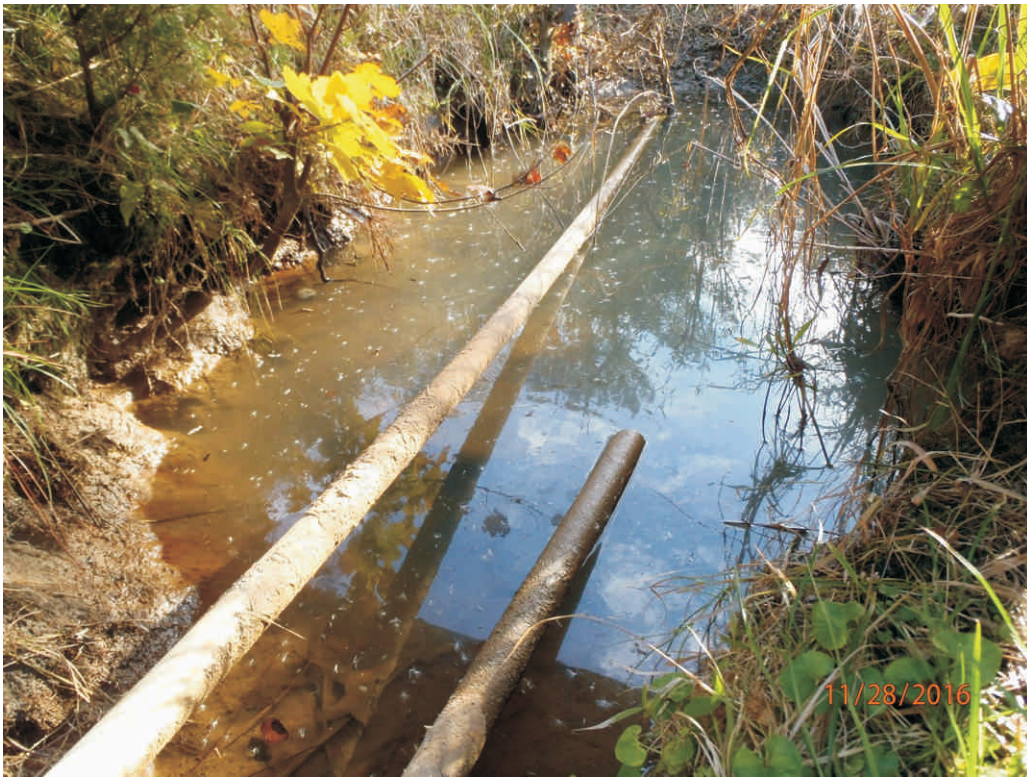
Enhancement Reach - Stream Problem Area #57a; Scour
