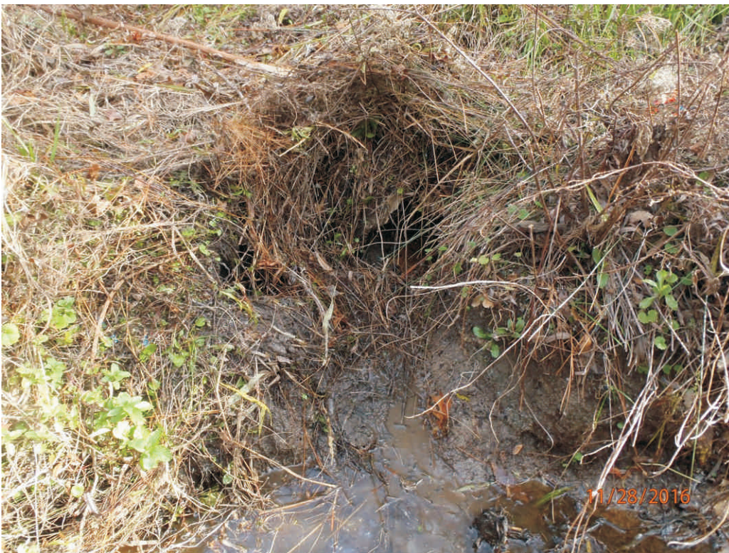
Reach B - Stream Problem Area #52; Mass Wasting
