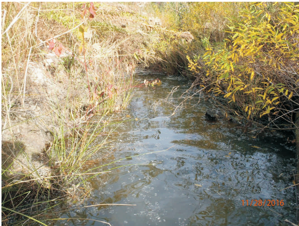
Reach 1A - Stream Problem Area #13a; Scour
