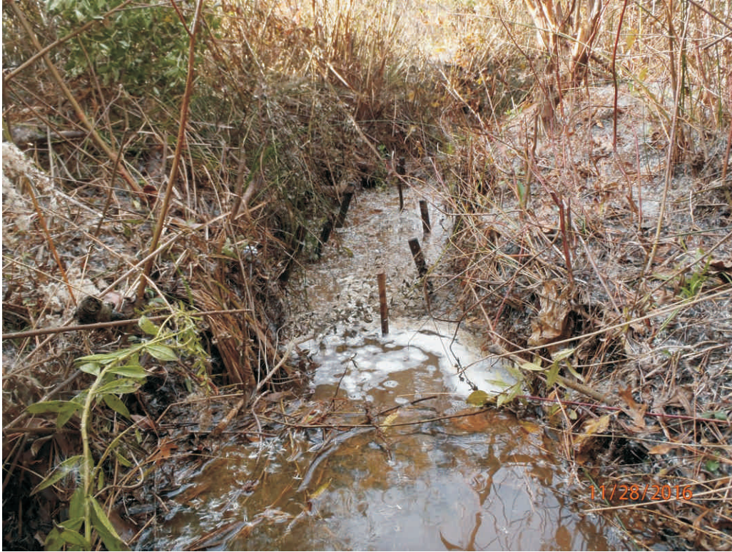
Reach B - Stream Problem Area #52a; Degradation
