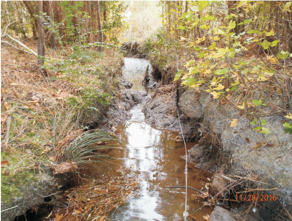
Reach 2A - Stream Problem Area #36; Degradation
