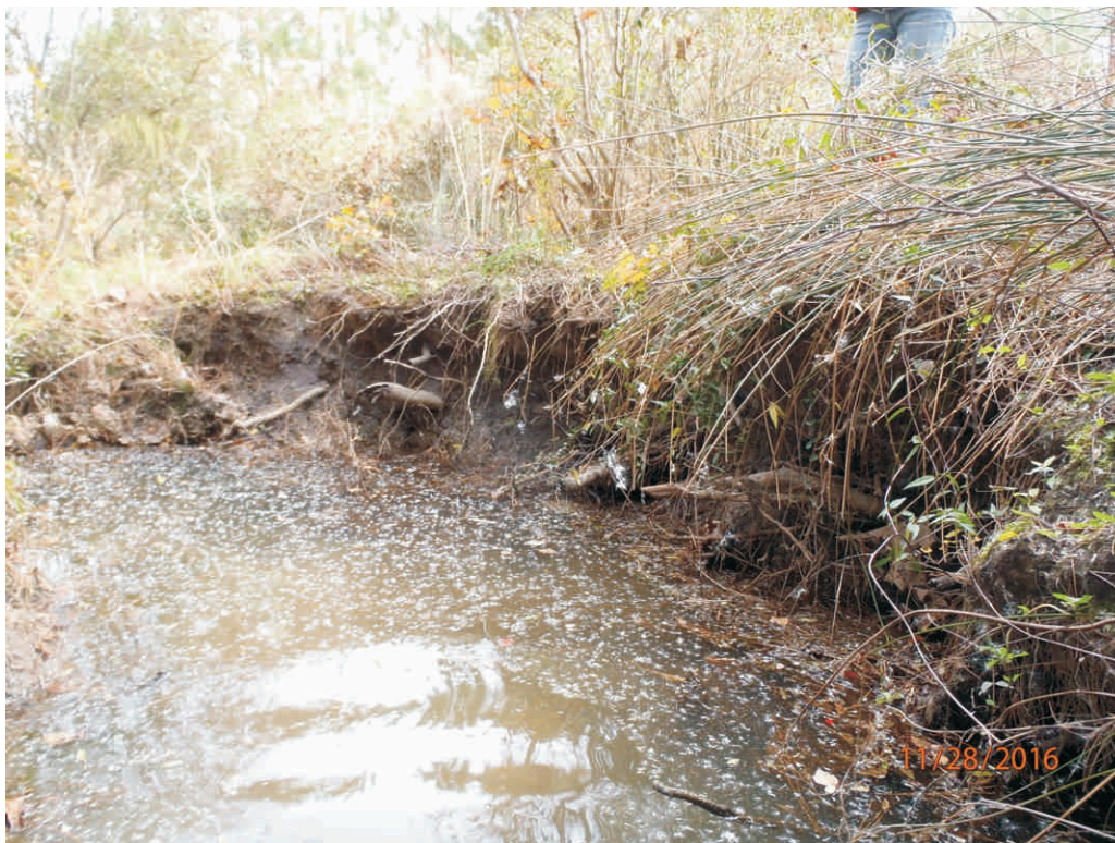
Reach 2A - Stream Problem Area #37; Undercut turning into Mass Wasting
