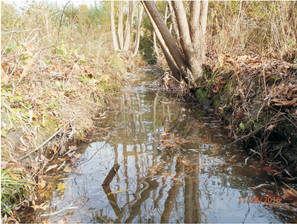
Reach 1A - Stream Problem Area #7; degradation
