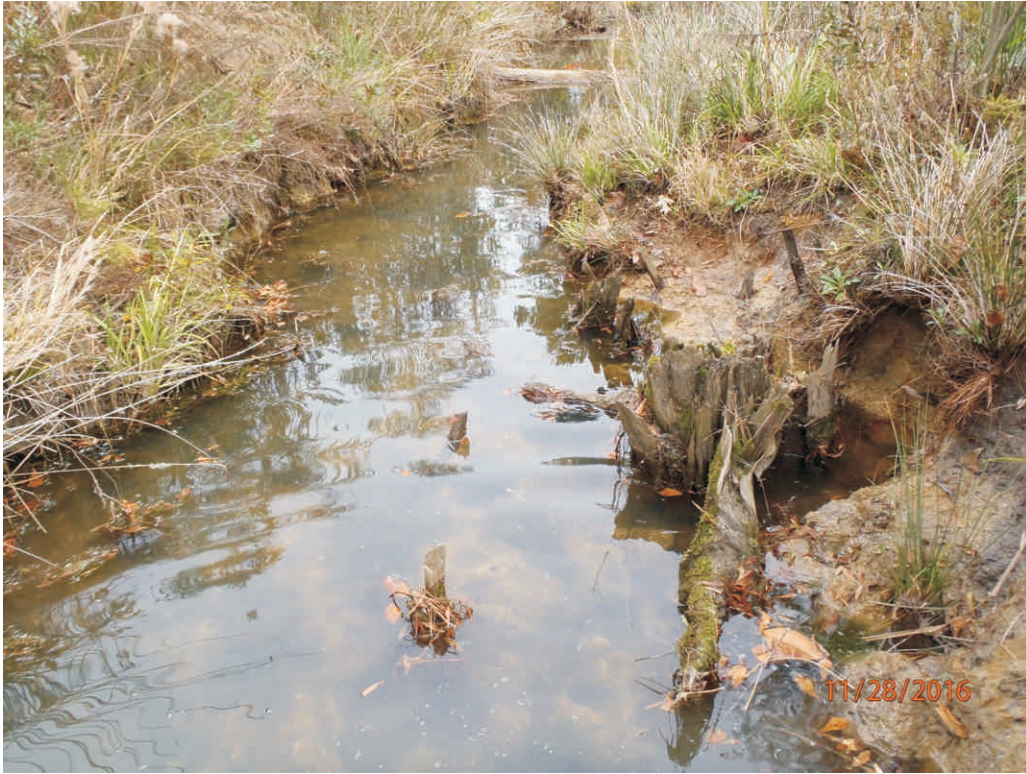
Reach 2A - Stream Problem Area #44; Scour
