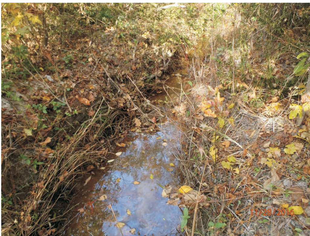
Reach 1A - Stream Problem Area #22; Degradation
